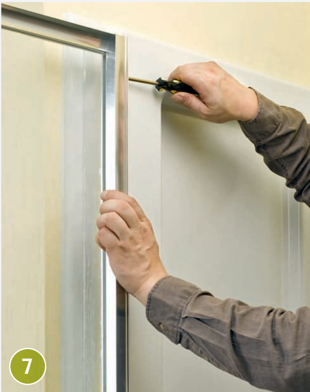
Fit the hinge jamb over the side jamb and adjust it as directed in your instruction manual. Once the clearances are correct, fasten the jambs to hang the door.
