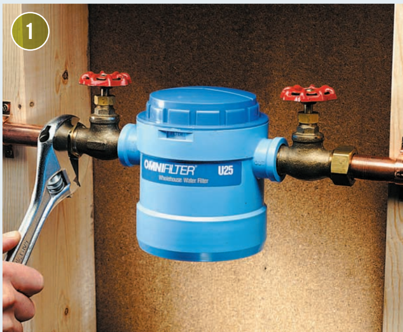
A whole-house water filtration system: (A) intake side, (B) supply pipe from the water meter pipe, (C) outlet side to the house supply pipe, (D) filter, and (E) filtration unit cover.
