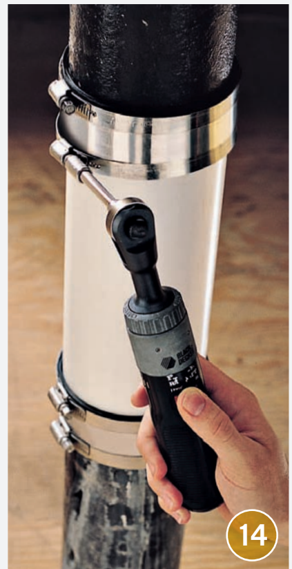
14 Tighten the screw clamps with a ratchet wrench or screwdriver.
