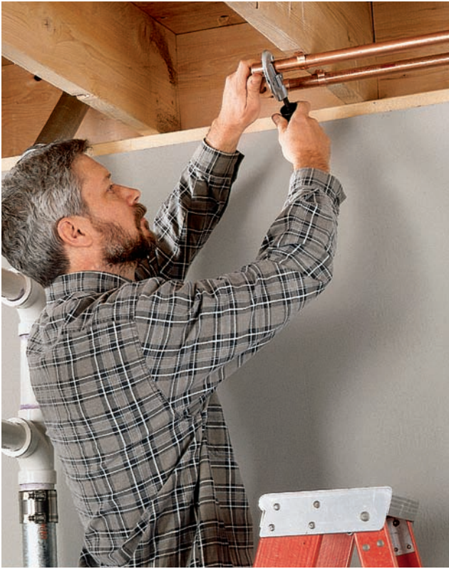
Use a tubing cutter to remove sections of branch supply lines.
