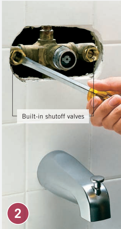
Turn off water supply at the built-in shutoff valves or the main shutoff valve.
