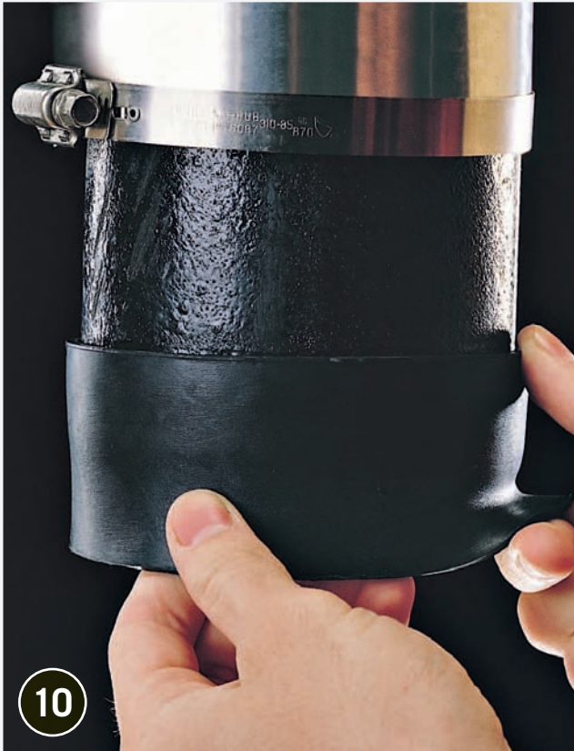
10 Fold back the end of each neoprene sleeve until the molded separator ring on the inside of the sleeve is visible.
