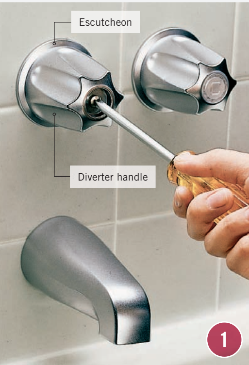
Remove the diverter valve handle with a screwdriver. Unscrew or pry off the escutcheon.
