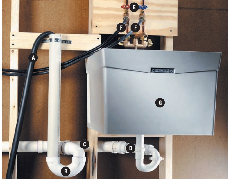
A washing machine with standpipe drain: washing machine drain hose (A), 2" standpipe drain with trap (B), waste line (C), utility sink drain pipe (D), hot and cold supply lines with hose bibs (E), rubber supply hoses to washing machine (F), and utility sink (G).
