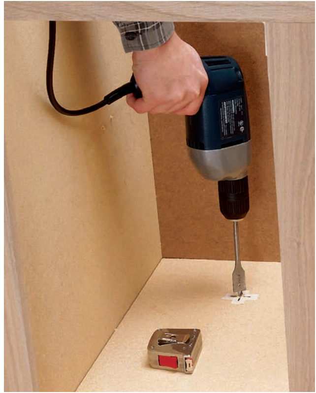
Drill access holes directly into a cabinet base to allow supply risers to enter the cabinet. The holes should align with access holes for the risers in the subfloor.
