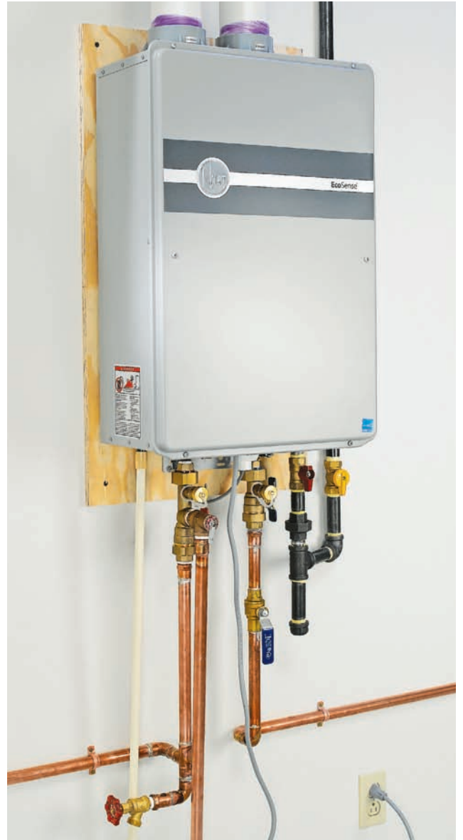
A tankless water heater can be installed near the old water heater’s location to minimize new water and gas pipe runs. It takes up far less space than a standard tank heater. The unit shown on the following pages is a gas-fired condensing unit, which requires two vent pipes; non-condensing units have only one vent pipe. Vent pipes run outside the house at a downward slope. There are connections and valves for a gas supply, a cold-water supply, and a hot-water line to the house, and the unit can simply be plugged into a 120-volt electrical receptacle.
