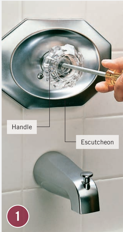
Use a screwdriver to remove the handle and escutcheon.
