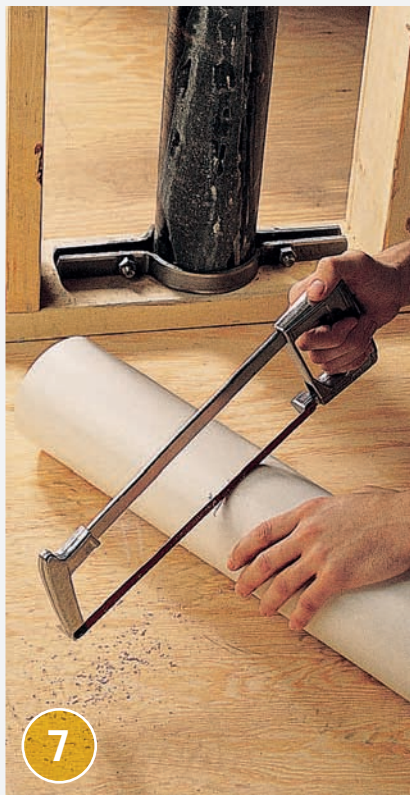
7 Cut a length of PVC plastic pipe to be ½" shorter than the section of cast-iron pipe that has been cut away.
