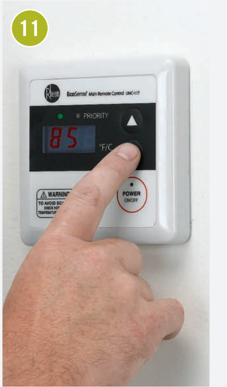
Program the thermostat. Turn off the gas and water to the water heater by closing the shutoff valves, and follow the manufacturer's instructions for setting the water temperature.
