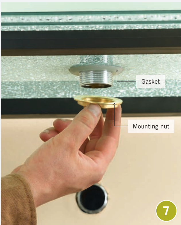
7 From underneath, push the large rubber gasket onto the threaded portion of the pop-up assembly. Thread the nut onto the pop-up assembly and tighten. Use an adjustable wrench or basin wrench to tighten an additional half turn. Thread the tailpiece onto the pop-up assembly.
