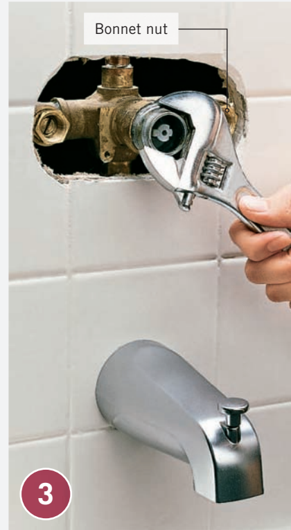
Unscrew and remove the retaining ring or bonnet nut using adjustable wrench.
