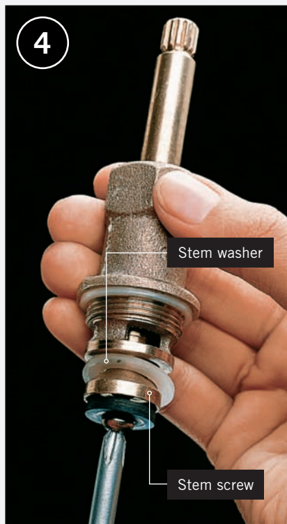
Remove brass stem screw. Replace stem washer with an exact duplicate. If stem screw is worn, replace it.
