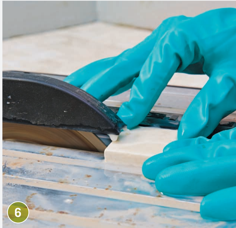
6 Cut the tiles along the trim lines using a tile saw. If you are not comfortable using a tile saw, score the tiles and cut them with tile nippers.
