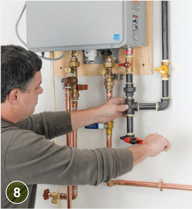
Hook up the gas connection. Working with black gas pipe, install a gas shutoff valve just below the unit, then install an union so you can easily disconnect the pipes for servicing. Connect the other pipes as shown; make sure to include a vertical sediment trap. Turn on the gas, and test with leak detector solution to make sure there are no leaks.
