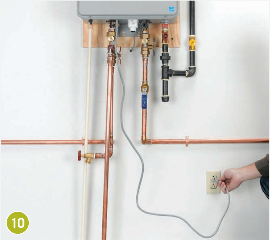
Test the water heater. Turn on the water supply and plug the unit into an electrical receptacle. Make sure you know which circuit breaker controls the water heater. When there is a demand for hot water (from a faucet or appliance), the water heater will turn on automatically and an electric spark will ignite the gas.
