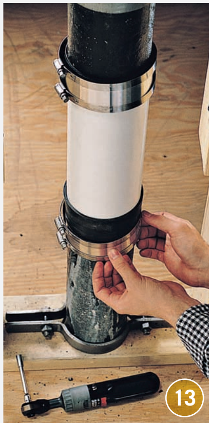
13 Slide stainless-steel bands and clamps over the neoprene sleeves.
