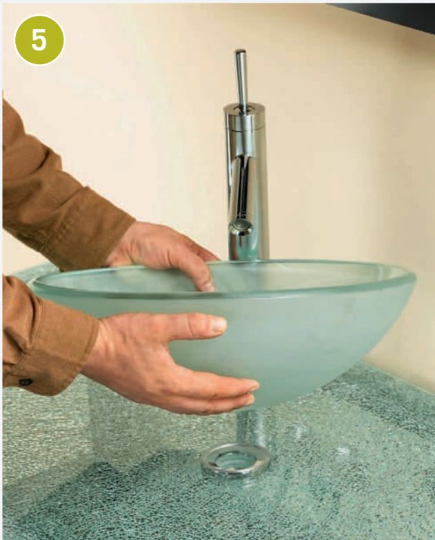
5 Place the vessel bowl on top of the O-rings. In this installation, the vessel is not bonded to the countertop.
