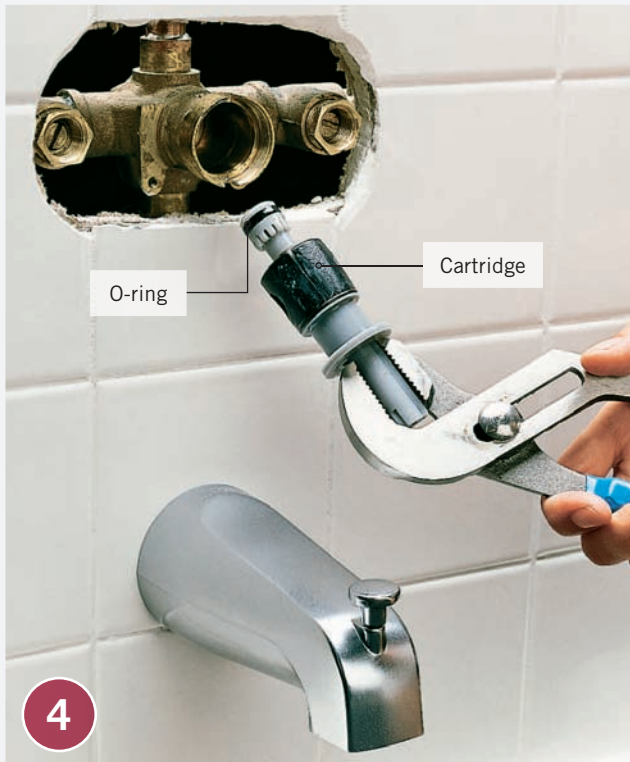
Remove the cartridge assembly by grasping the end of the valve with channel-type pliers and pulling gently.
