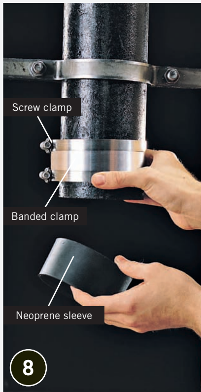
8 Slip a banded coupling and a neoprene sleeve onto each end of the cast-iron pipe.
