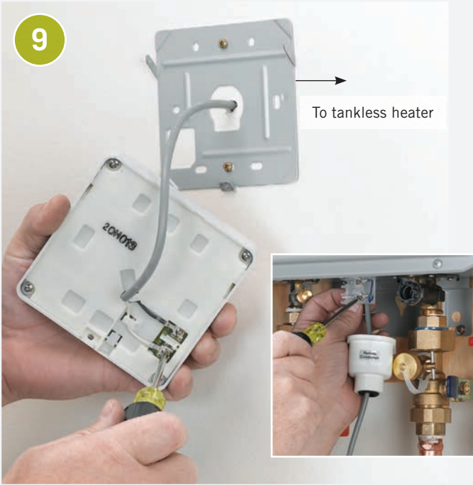
Connect the thermostat. Connect two-wire thermostat cable to the unit (inset), and run it to a convenient location for controlling the water heater. Attach the thermostat's plate to the wall and run the cable through it. Attach the wires to the back of the thermostat's cover, and snap on the cover.
