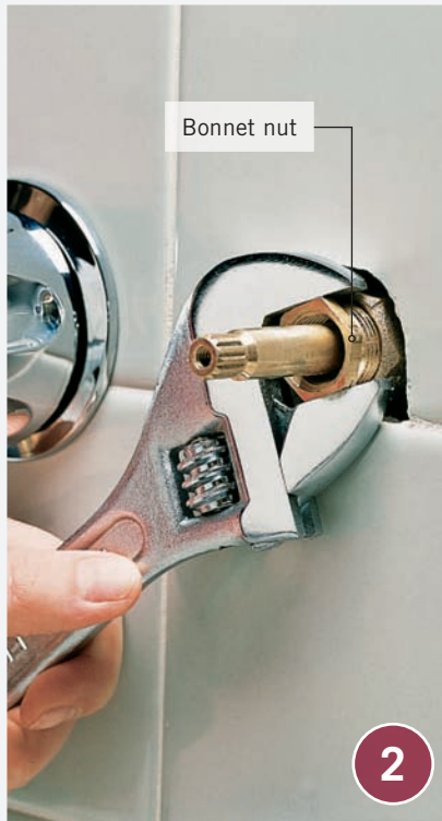
Remove bonnet nut with an adjustable wrench or channel-type pliers.
