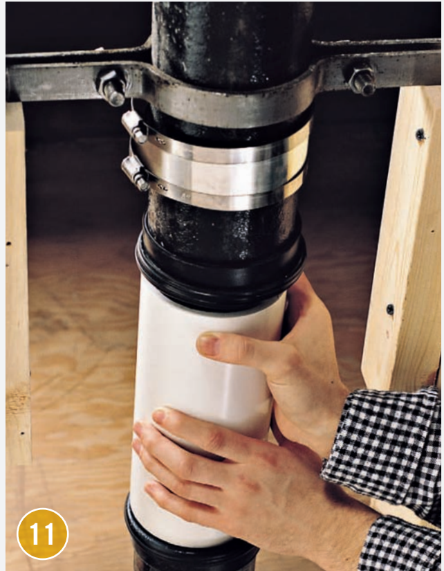
11 Position the new plastic pipe so it is aligned with the cast-iron pipes.
