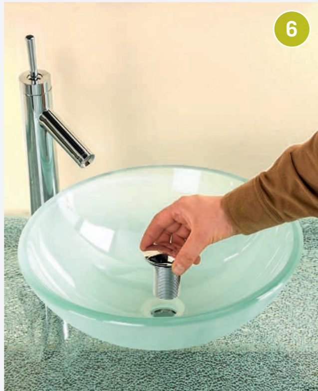
6 Put the small rubber gasket over the drain hole in the vessel. From the top, push the pop-up assembly through the drain hole.
