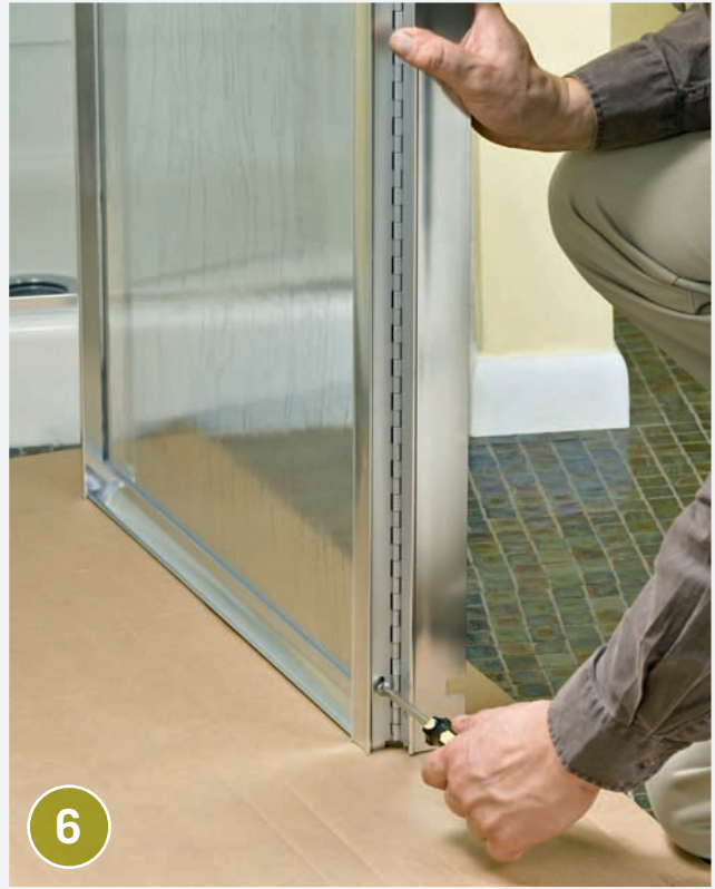
Attach the hinge to the door panel , according to the manufacturer's instructions. Attach any cap fitting that keeps water out of the jamb.
