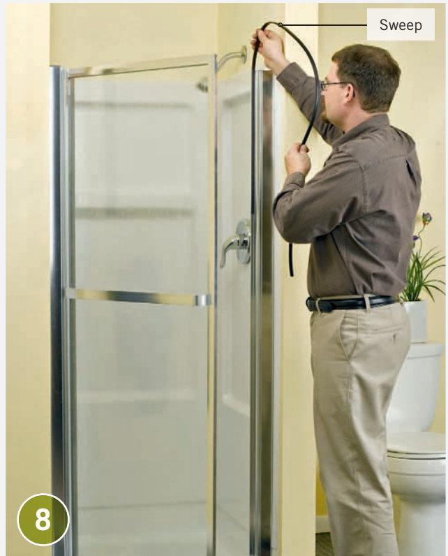
Install the magnetic strike plate and any remaining caps or accessories such as towel rods. Also attach the sweep that seals the passage, if provided.
