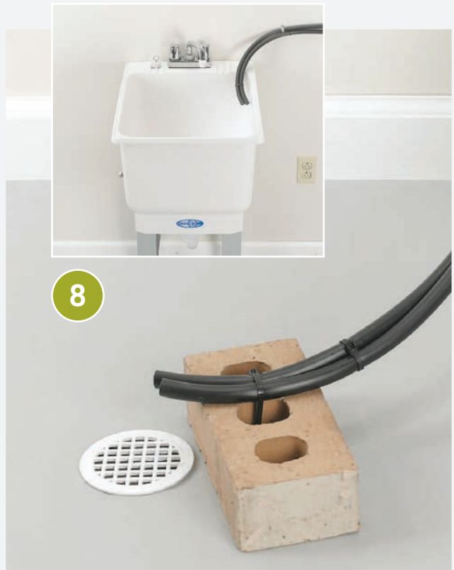
8 Run the tank overflow hose and the drain tube to a nearby floor drain or utility sink (not into a drain or vent pipe). The hoses should be secured so they don't flop around, and their ends must be at least 1½" above a drain.
