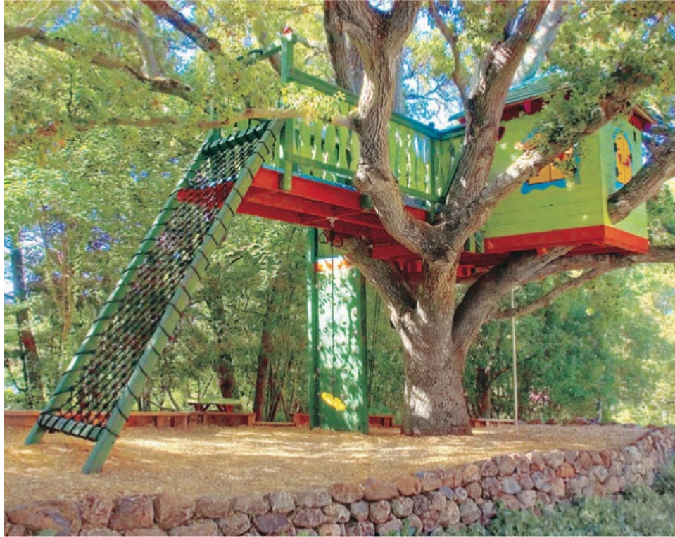
Vibrant colors and fun shapes add whimsy and playfulness to this treehouse, which also features a unique limb penetration through a sidewall.
