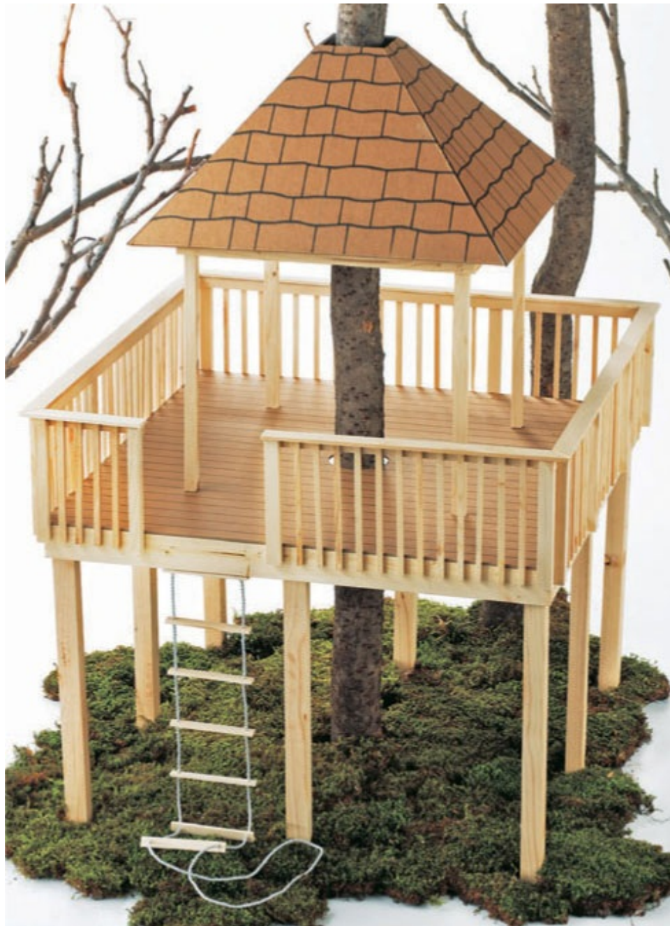
Hip roofs are sloped on all sides and are more difficult to frame than sheds and gables.
