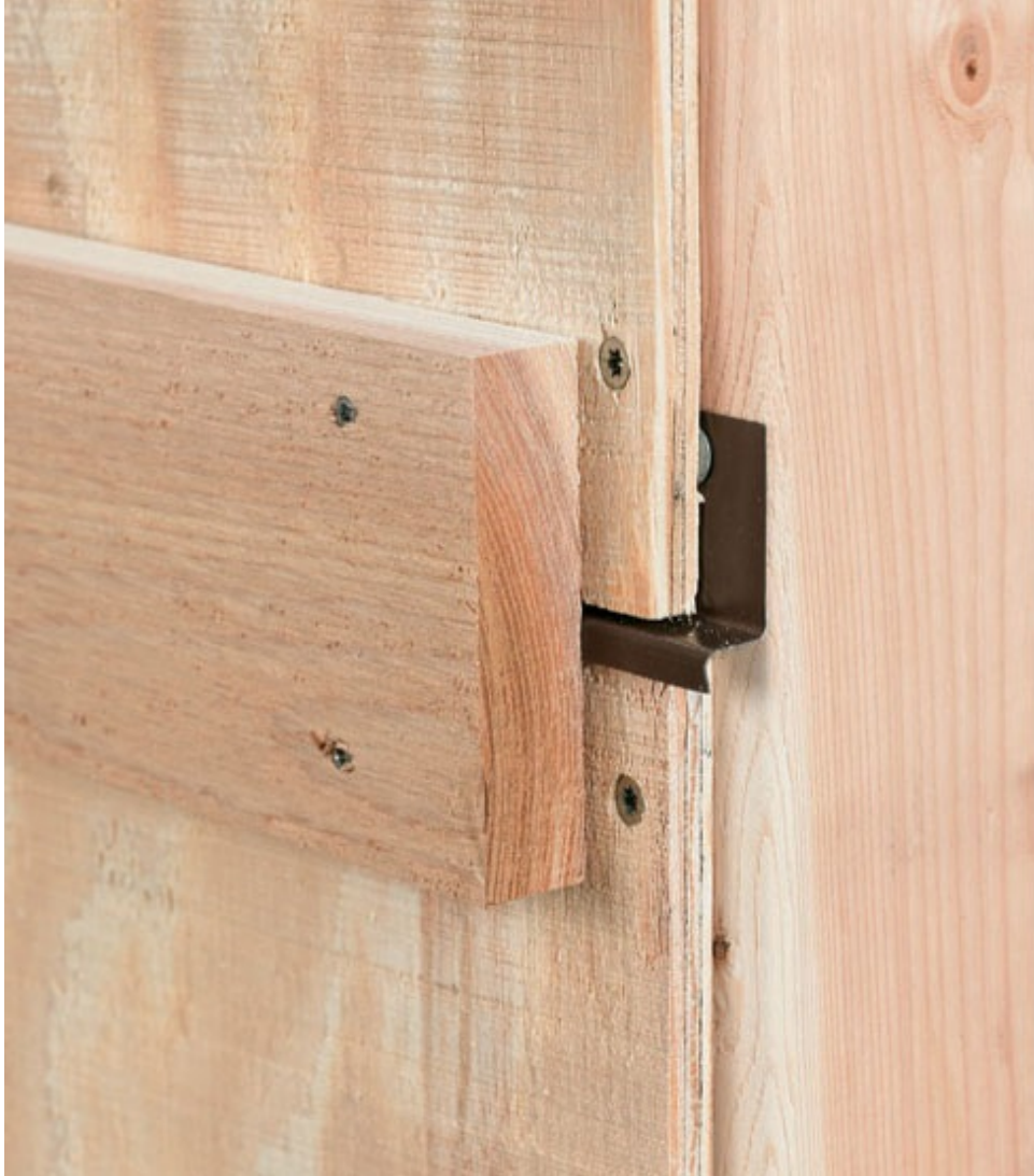
Horizontal siding joints and similar seams can be covered with trim so they look like design elements instead of construction joints.
