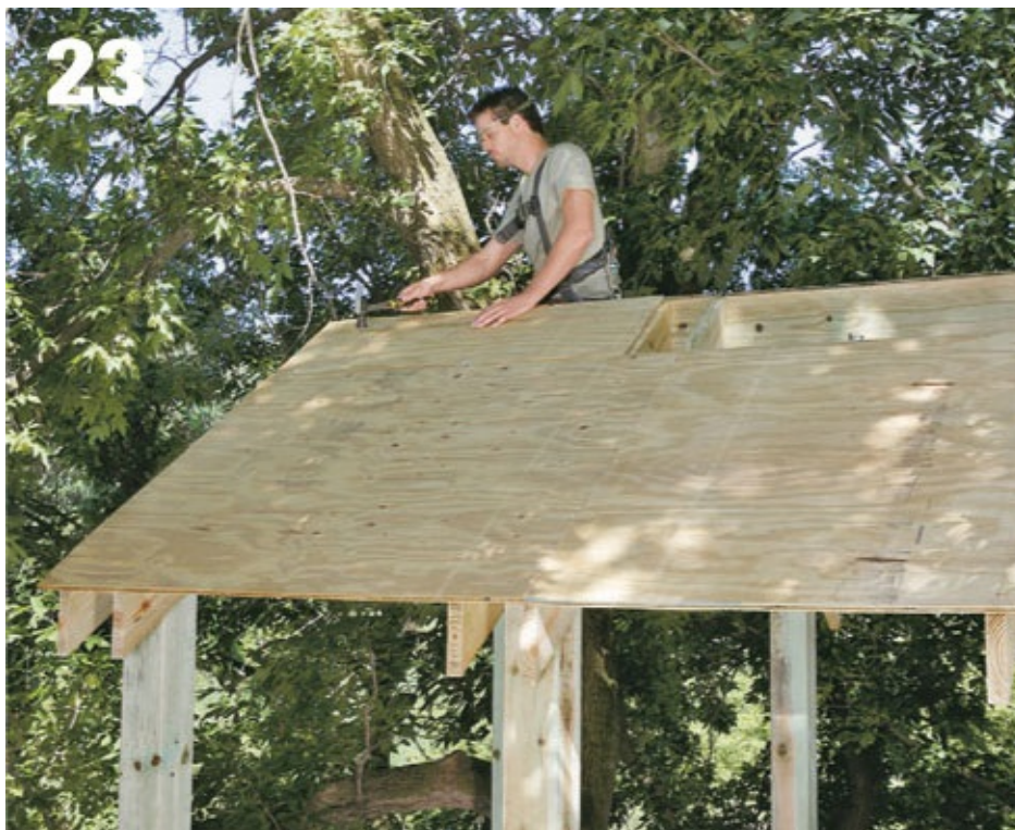
Tongue-and-groove roof decking is required for the relatively wide spans of the rafters. Follow the manufacturer's specifications for gapping between panels.
