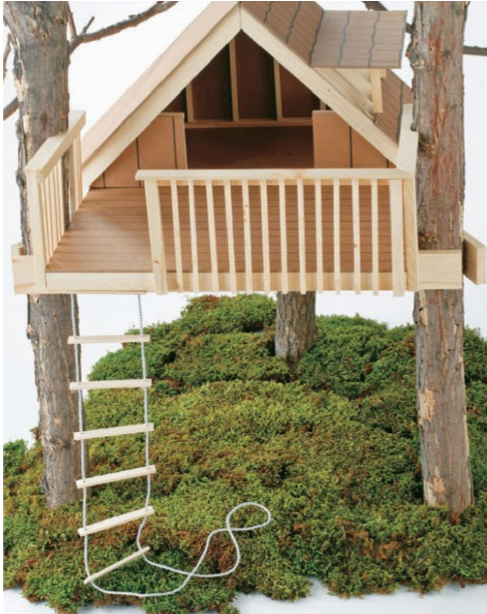
Stairs or a ladder require a top landing; adding a foot or two of space to the landing lets it double as a sitting area.
