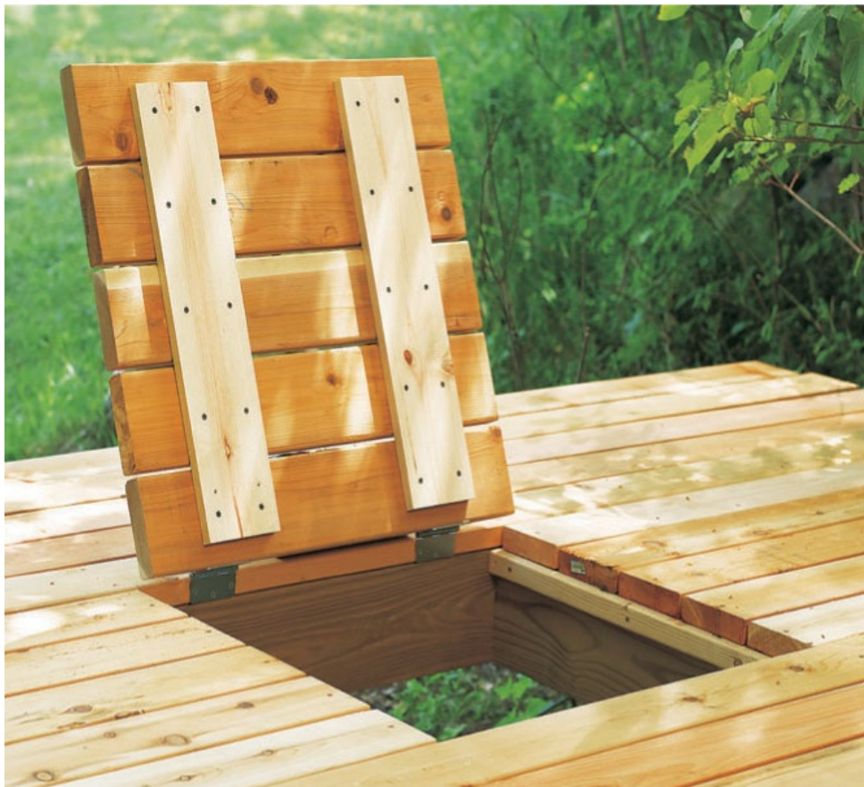
Joist headers support the ends of the cut joist and become two sides of the door opening frame.
