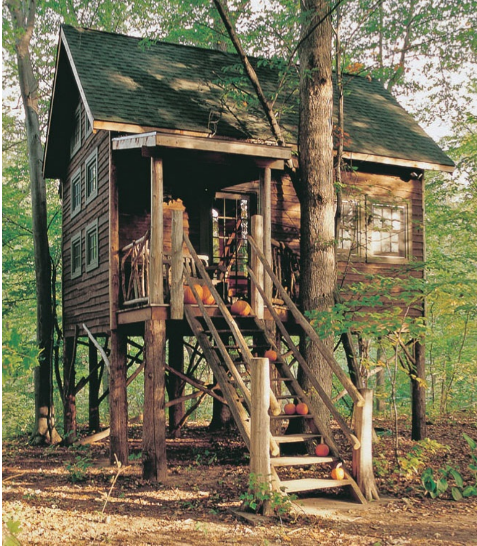
An elevated house in the trees with an independent post support system has the appeal of a tree-built treehouse but without many of the structural limitations.
