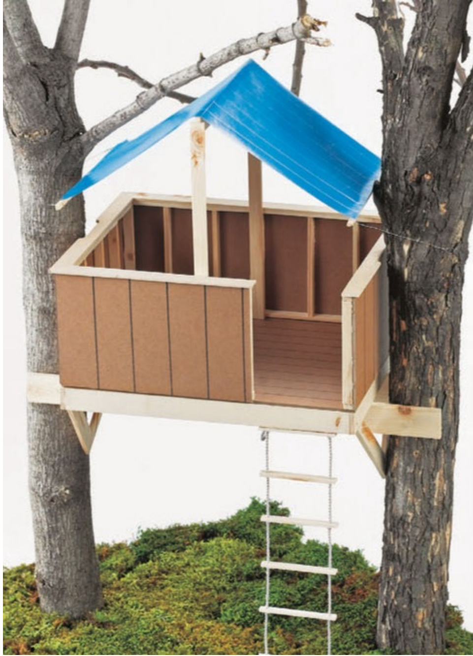
A removable roof made from canvas or a plastic tarp may be all you need to shelter a tree fort or sun deck.
