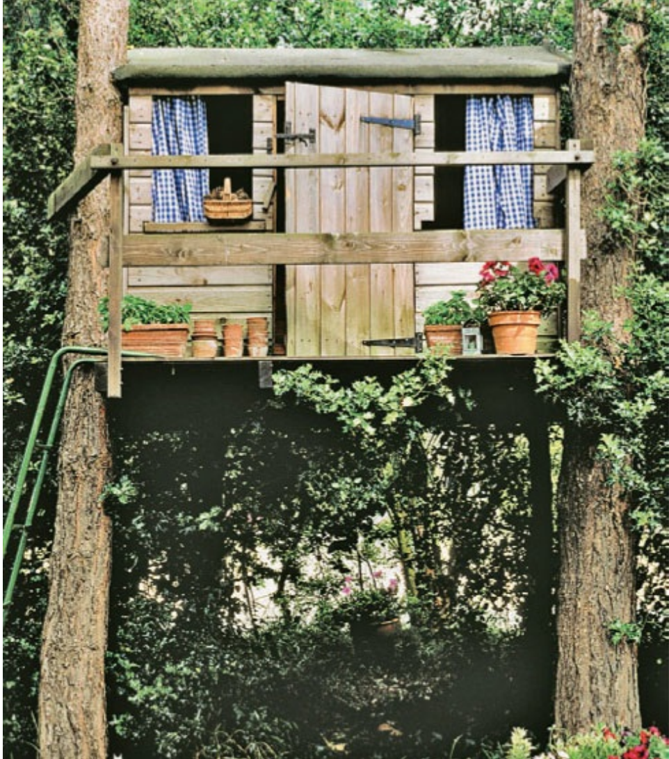
A pair of trees roughly the same size provide solid support for a treehouse that's nestled between them.
