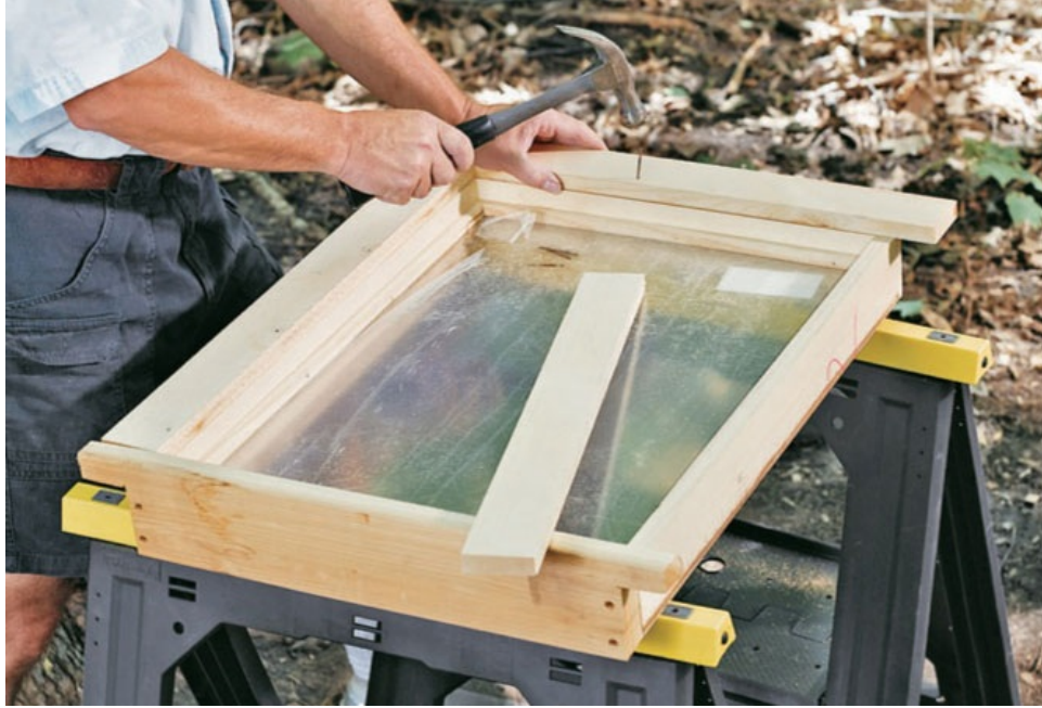
Simple homemade windows are easy to make with plastic glazing and scrap lumber.
