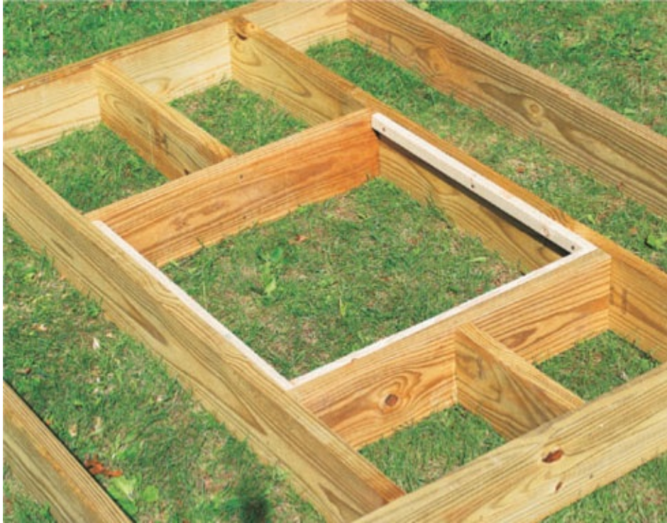
Joist headers support the ends of the cut joist and become two sides of the door opening frame.
