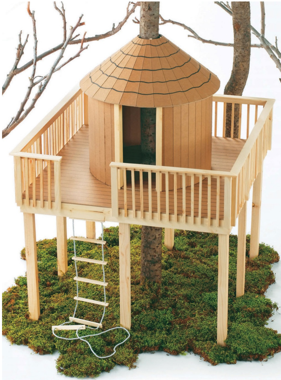
A conical roof is an impressive way to top a rounded wall. They're built with closely spaced rafters fanning out from the roof peak.
