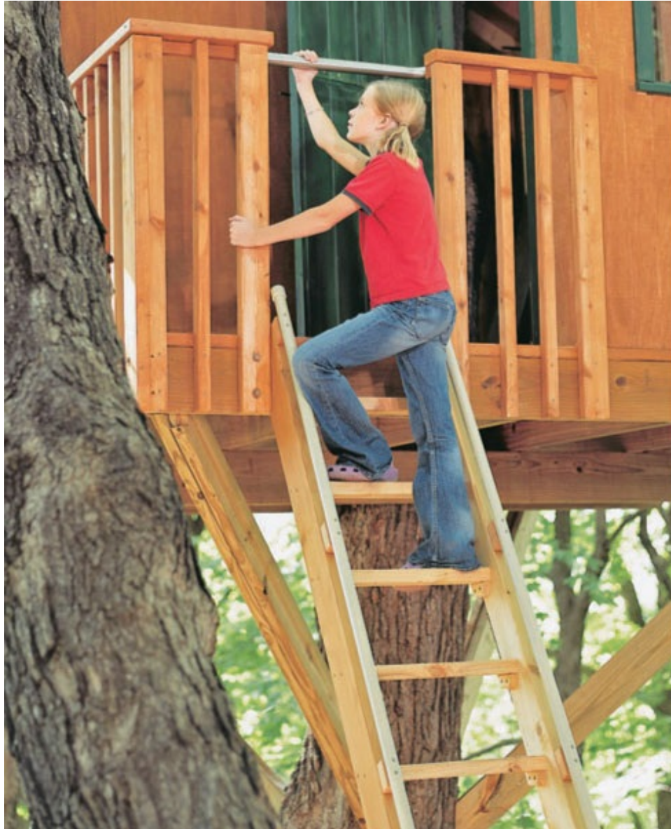
A sturdy handle is a welcome sight to tired climbers. Make sure all handles and mounting hardware are galvanized or otherwise corrosion-protected.
