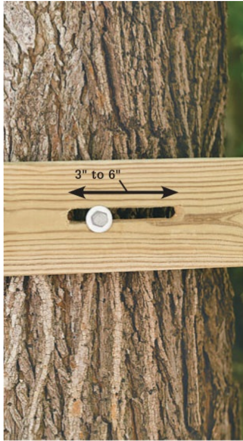
A slot-type sliding anchor allows single-directional movement between the tree or trees and the platform beams.
