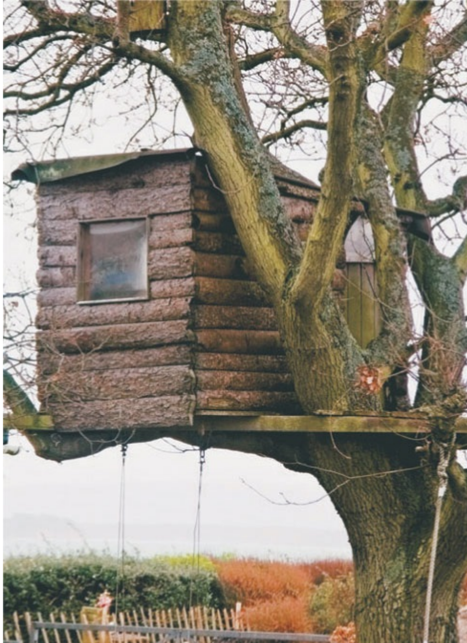
A treehouse is a fortress of fun even with siding from bark slabs and a tar paper roof. In fact, these simple materials have a beauty all their own that many designers find appealing.
