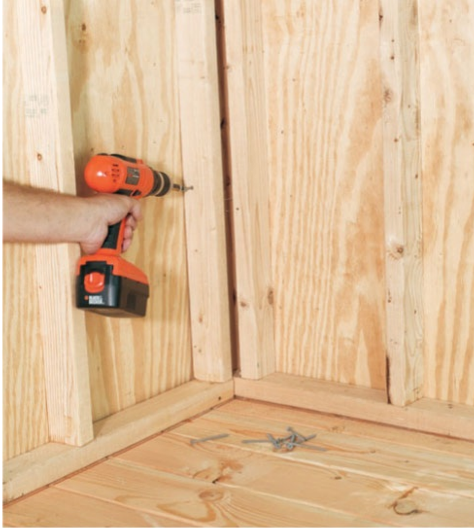
Join the walls with screws driven through the end studs.
