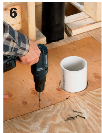
6 Cut a piece of exterior-grade plywood to fit the cutout floor area, and use a jigsaw to cut an opening for the toilet drain stub-out. Position the plywood, and attach it to joists and blocking with 2" screws.
