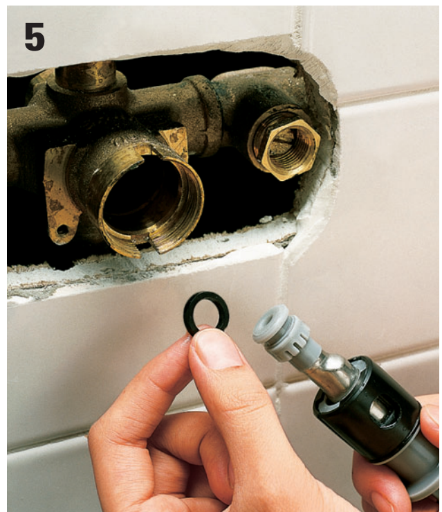
5 Flush the valve body with clean water to remove sediment. Replace any worn O-rings. Reinstall the cartridge and test the valve. If the faucet fails to work properly, replace the cartridge.
