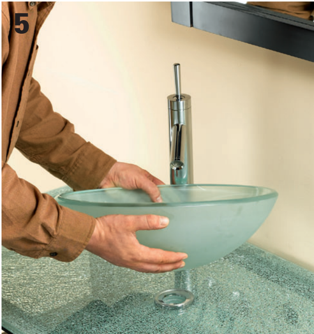
5 Place the vessel bowl on top of the O-rings. In this installation, the vessel is not bonded to the countertop.
