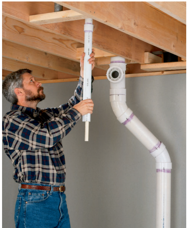
Probe wall and floor cavities with a long piece of plastic pipe to ensure that a clear pathway exists for running new pipe (left photo). Once you have established a route using the narrow pipe, you can use the pipe as a guide when running larger drain pipes up into the wall (right photo).
