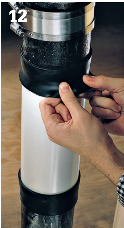
12 Roll the ends of the neoprene sleeves over the ends of the new plastic pipe.
