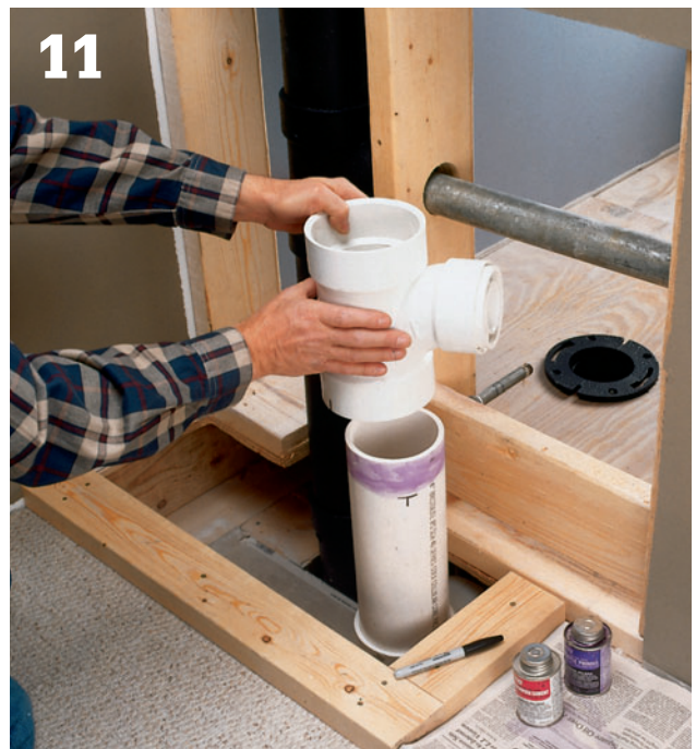
11 Add additional lengths of pipe, with waste T-fittings installed where other fixtures will drain into the stack. In our example, a waste-T with a \frac{1}{2} " bushing insert was installed where the vanity sink drain was attached to the stack. Make sure the T-fittings are positioned to allow for the correct downward pitch of the branch drains.
