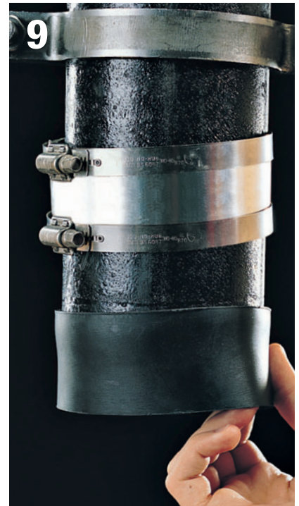
9 Make sure the cast-iron pipe is seated snugly against the rubber separator ring molded into the interior of the sleeve.
