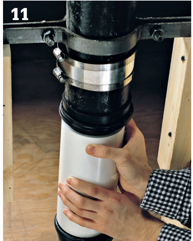
11 Position the new plastic pipe so it is aligned with the cast-iron pipes.
