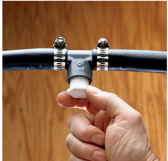
Connect lengths of PE pipe with a barbed PVC fitting. Secure the connection with stainless steel hose clamps.
