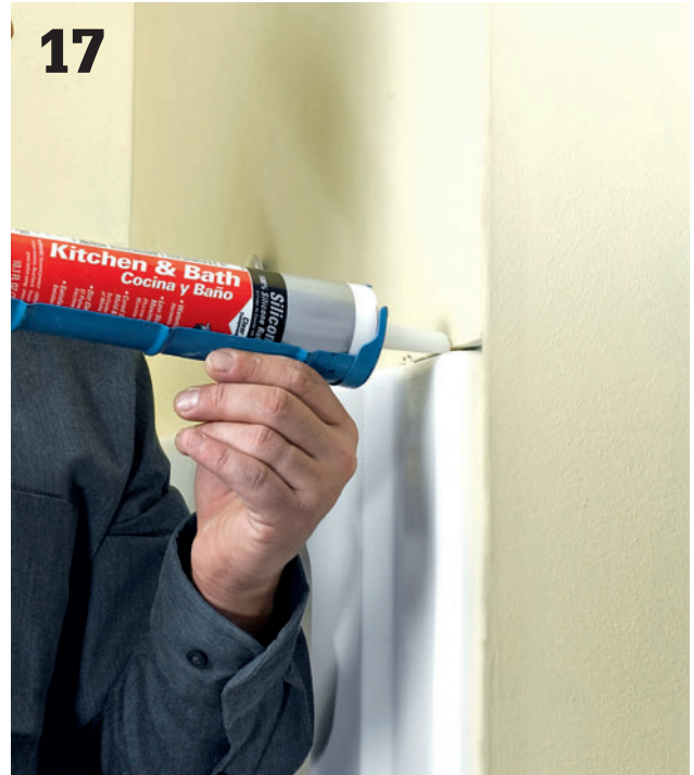
17 Finish the walls and then caulk between the enclosure panels and the wallcoverings with silicone caulk.
