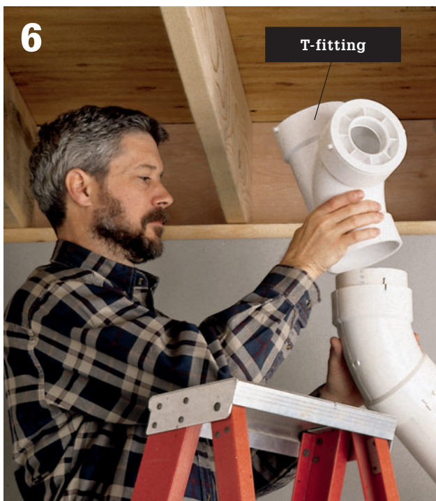
Dry-fit a waste T-fitting on the stack , with the inlets necessary for any branch drains that will be connected in the basement. Make sure the fitting is positioned at a height that will allow the branch drains to have the correct \frac{1}{4} " per ft. downward slope toward the stack.
