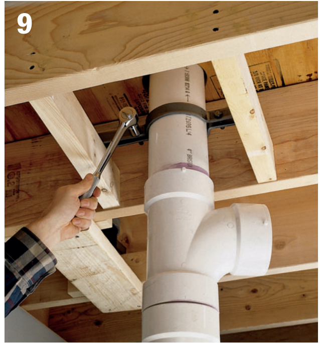
9 Check the length of the stack, then solvent-glue all fittings together. Support the new stack with a riser clamp resting on blocks attached between basement ceiling joists.
