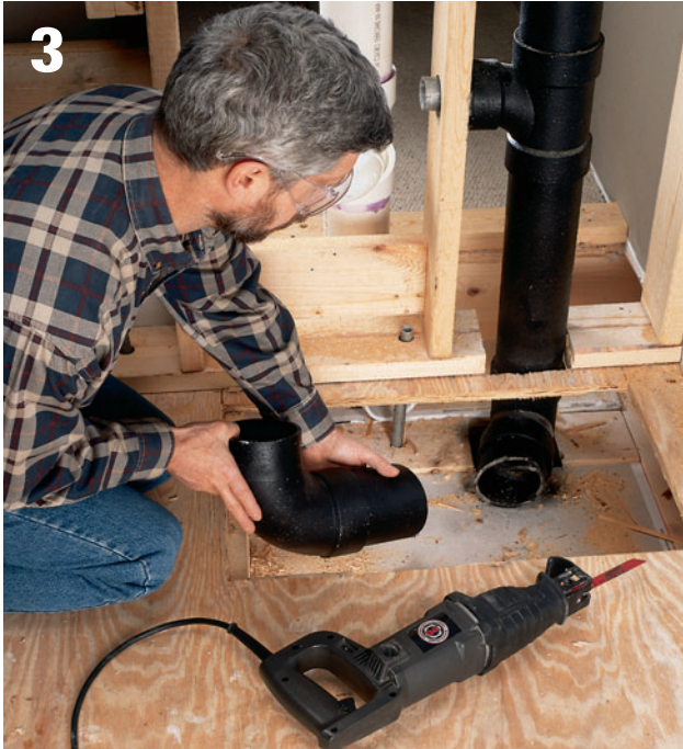
3 Cut away the old closet bend as close as possible to the old waste-vent stack, using a reciprocating saw with metal-cutting blade, or a cast iron cutter.
