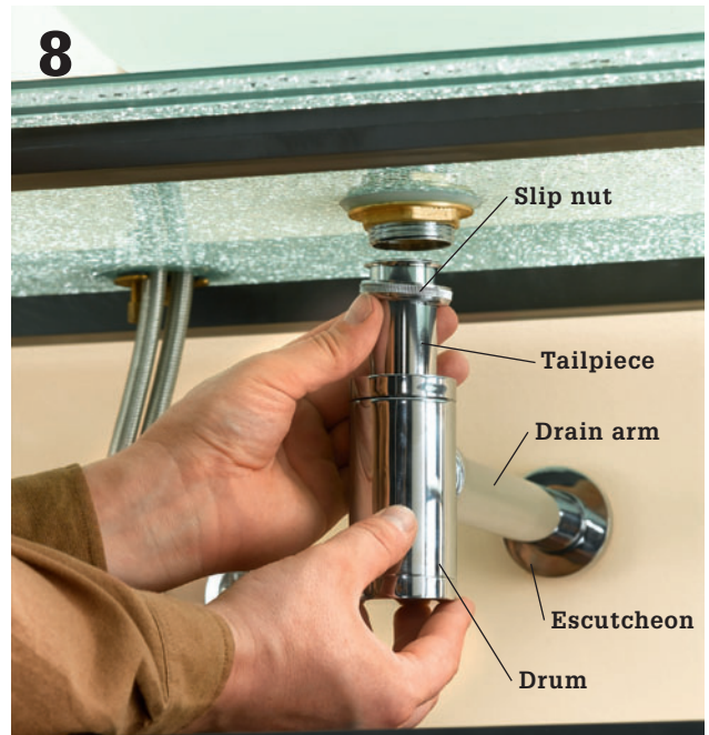
8 Install the drum trap. Loosen the rings on the top and outlet of the drum trap. Slide the drum trap top hole over the tailpiece. Slide the drain arm into the side outlet, with the flat side of the rubber gasket facing away from the trap. Insert the drain arm into the wall outlet. Hand tighten the rings.
