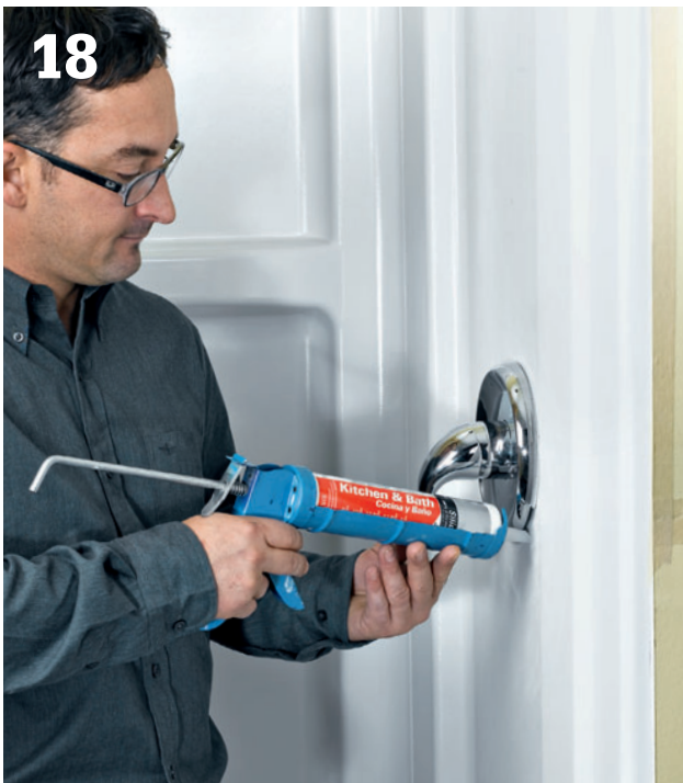
18 Install the faucet handles and escutcheon and caulk around the escutcheon plate. Install the shower arm escutcheon and showerhead.
