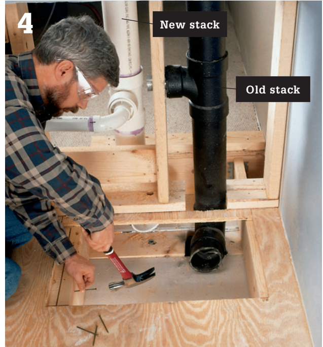
4 If a joist obstructs the route to a new waste-vent stack, cut away a section of the floor joist. Install double headers and metal joist hangers to support the ends of the cut joist.
