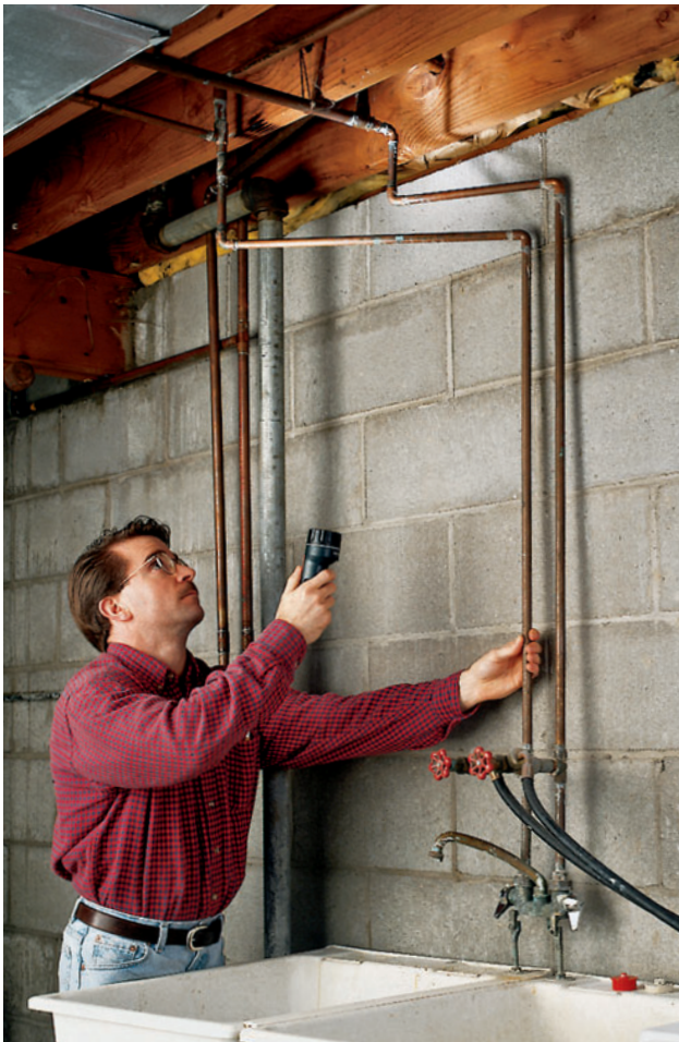
Snoop around your basement for clues about the locations of supply, drain, vent, and gas pipes in your walls.
