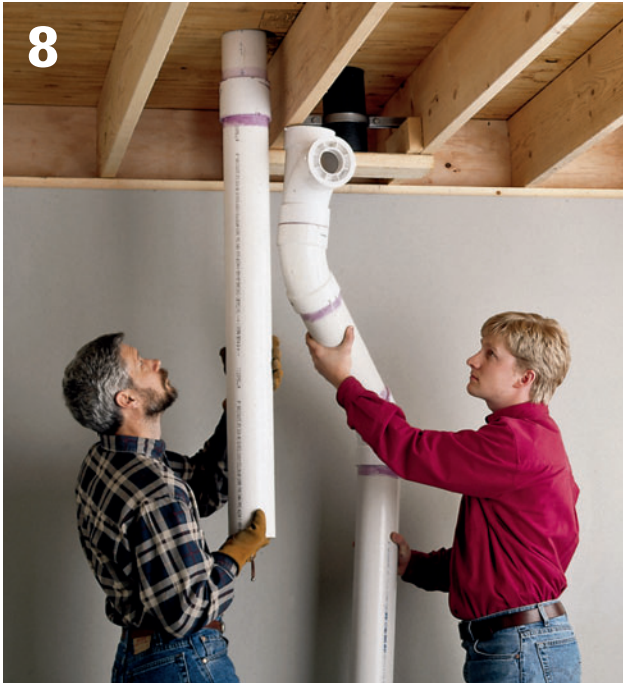
8 Cut a PVC plastic pipe to length, raise it into the opening, and dry-fit it to the T-fitting. Note: For very long pipe runs, you may need to construct this vertical run by solvent-gluing two or more segments of pipe together with couplings.
