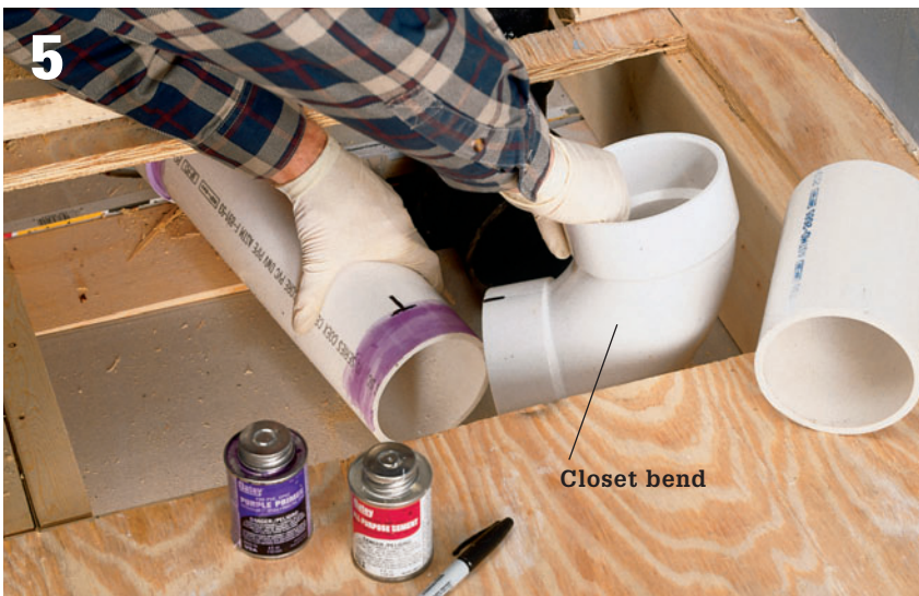
5 Create a new toilet drain running to the waste-vent stack, using a closet bend and a straight length of pipe. Position the drain so there will be at least 15" of space between the center of the bowl and side wall surfaces when the toilet is installed. Make sure the drain slopes at least \frac{1}{4} " per ft. toward the stack, then support the pipe with plastic pipe strap attached to framing members. Insert a 6" length of pipe in the top inlet of the closet bend; once the new drain pipes have been tested, this pipe will be cut off with a handsaw and fitted with a toilet flange.
