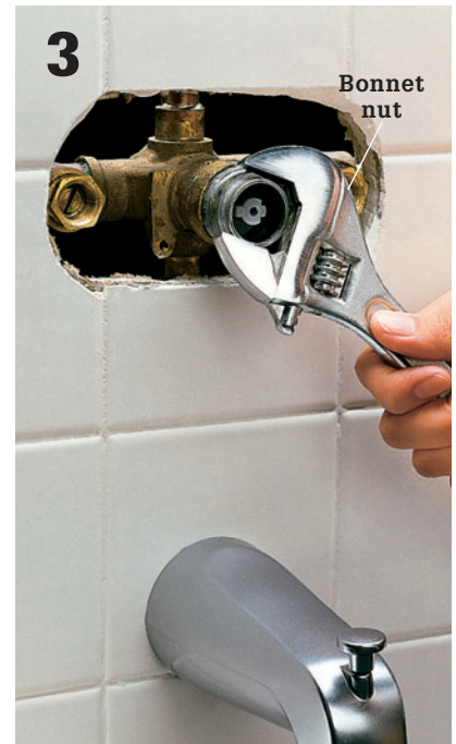
3 Unscrew and remove the retaining ring or bonnet nut, using adjustable wrench.
