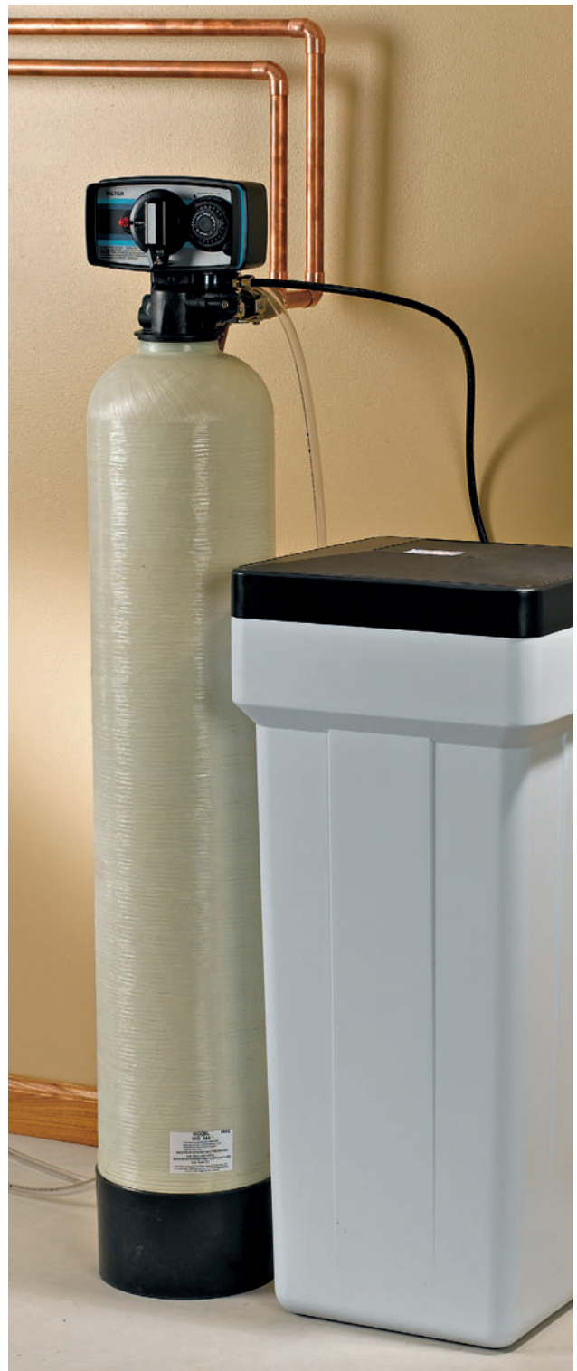
A water softener is a two-part appliance that includes the water softener itself (to the left, above) and an attached salt storage tank (right).
