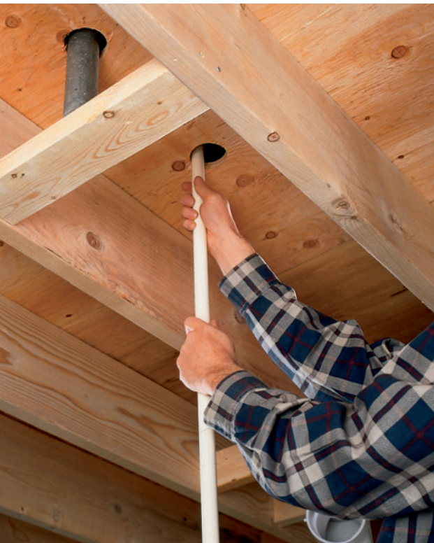
Probe wall and floor cavities with a long piece of plastic pipe to ensure that a clear pathway exists for running new pipe (left photo). Once you have established a route using the narrow pipe, you can use the pipe as a guide when running larger drain pipes up into the wall (right photo).
