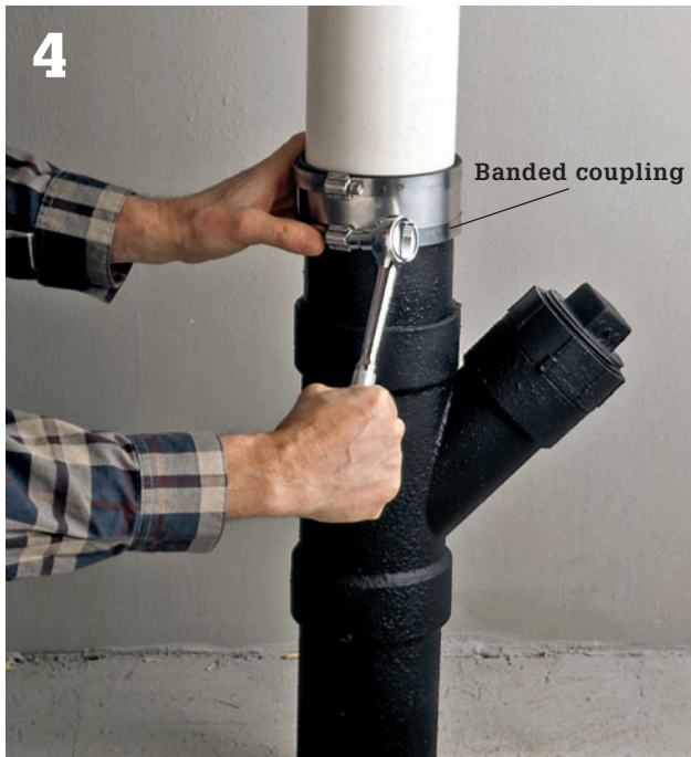
Attach a 5-ft. segment of PVC plastic pipe the same diameter as the old waste-vent stack to the exposed end of the cast-iron cleanout fitting, using a banded coupling with neoprene sleeve.
