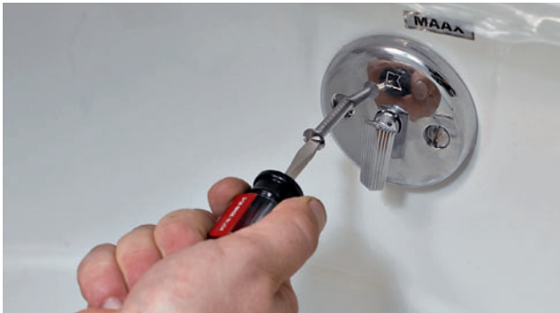
Secure the drain/overflow assembly by tightening the overflow coverplate and the drain strainer onto the assembly, from inside the tub.
