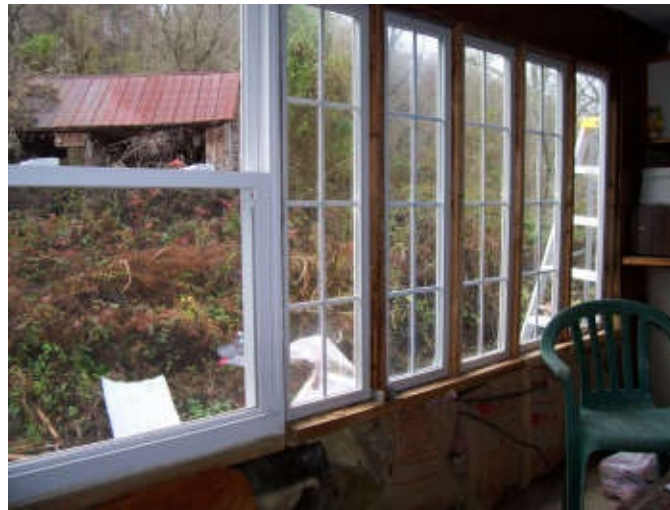
We closed in our trailer with double-glazed windows.
