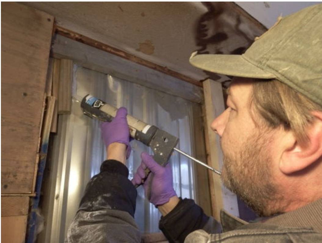
Sealing any cracks with silicone will keep cold air out in the winter. In this
