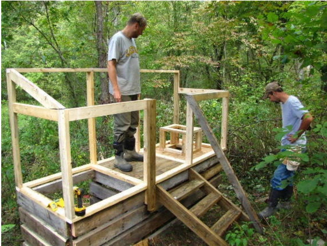
Our composting-toilet system combines features of outhouses with the hot-composting method outlined in The Humanure Handbook .
