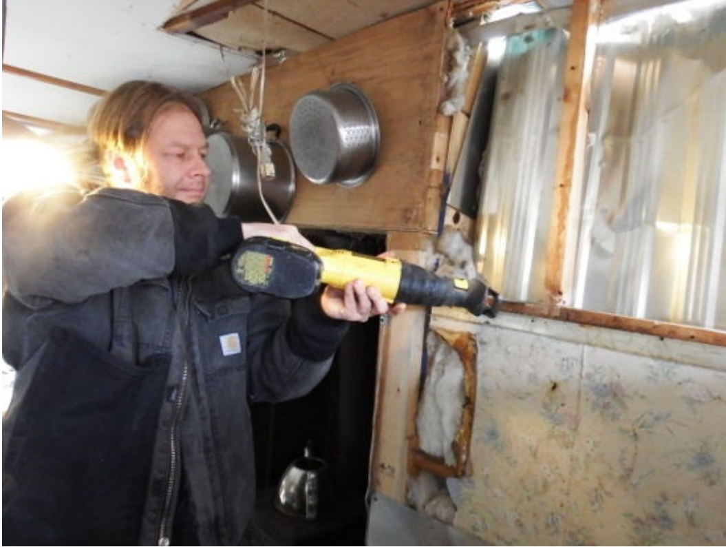
A problematic stud is easy to remove with a reciprocating saw.
