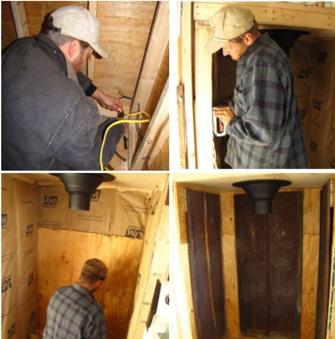
We used old roofing metal spaced an inch away
