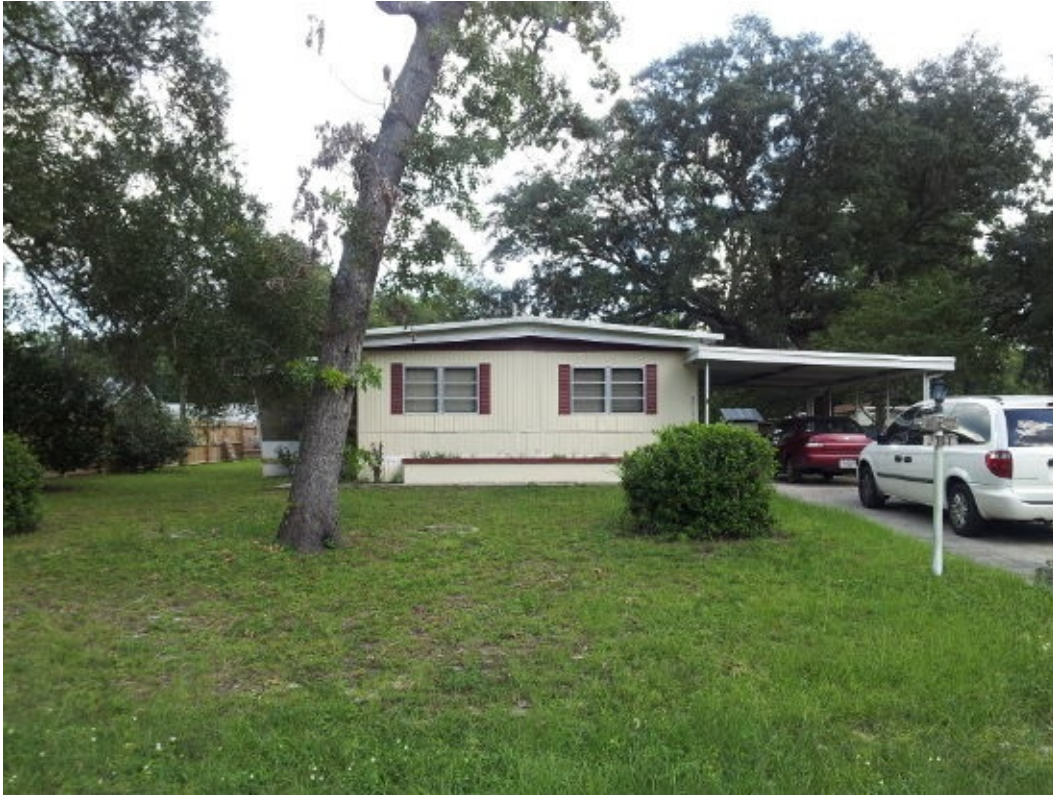
The double-wide trailer, land, and associated facilities cost $14,500 in 2014. Photo credit: Brian and Stephanie Larsen.
