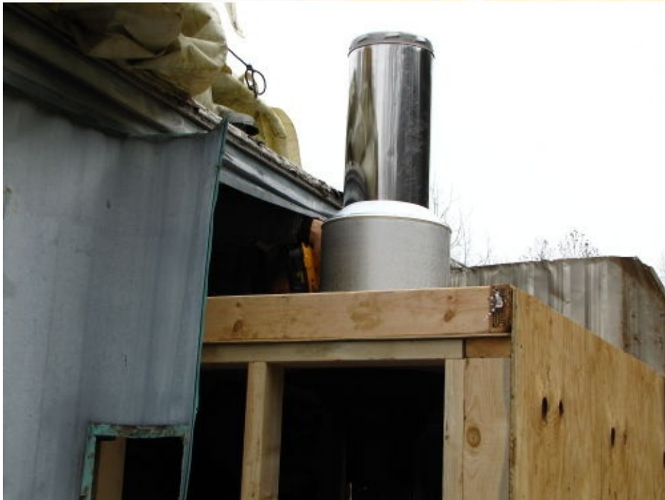
A ceiling support kit, available for around $300 or less from a store like Lowes, will expedite wood-stove installation.
