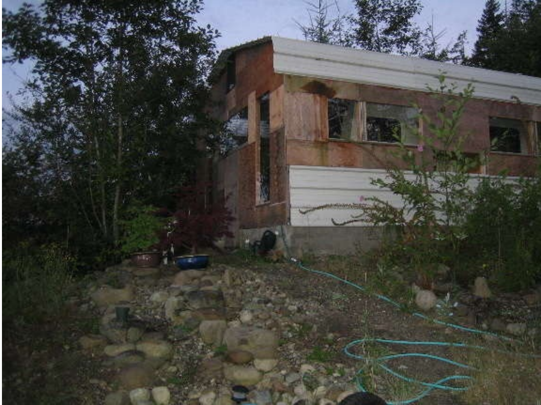
To keep the trailer warm, Will erected a passive-solar shell around it. Photo credit: Will.
