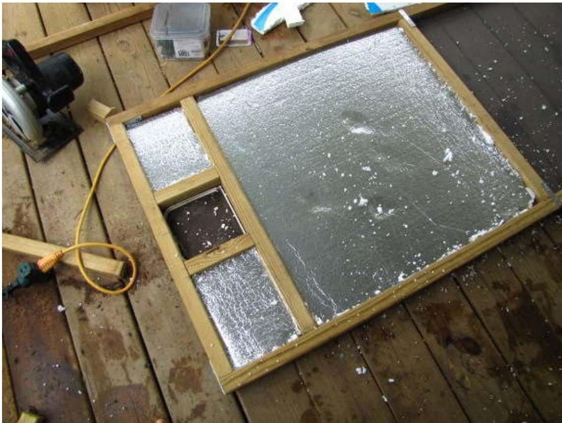
Styrofoam forms an insulative core within the solid part of the door.
