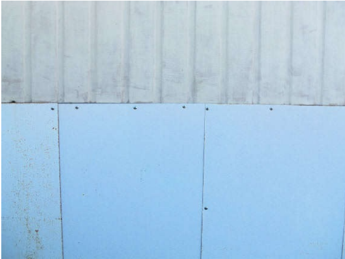
Jonathan's insulated skirting is made of pieces cut out of door panels. Photo credit: Jonathan Combs.
