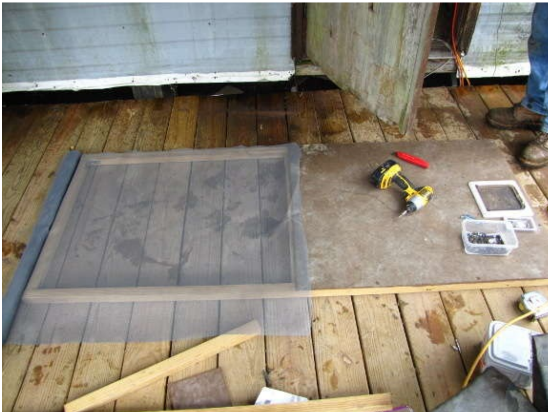
Two-by-twos, a bit of particle board, a few brackets and screws, and some screen formed the majority of the door.
