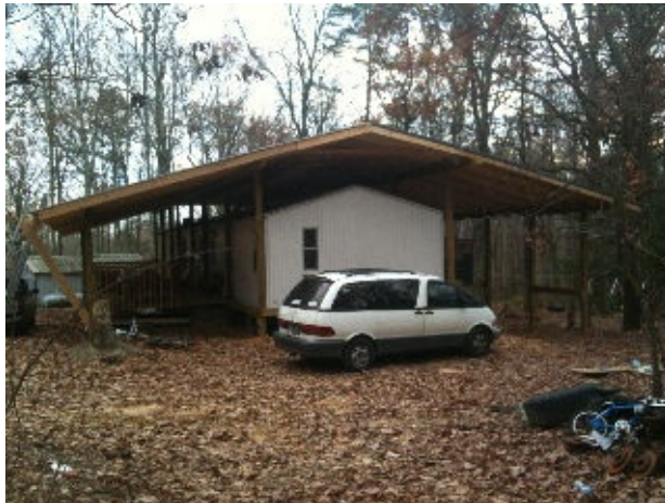
A pavilion-style roof protects two joined trailers. Photo credit: Lindsey and Keith.
