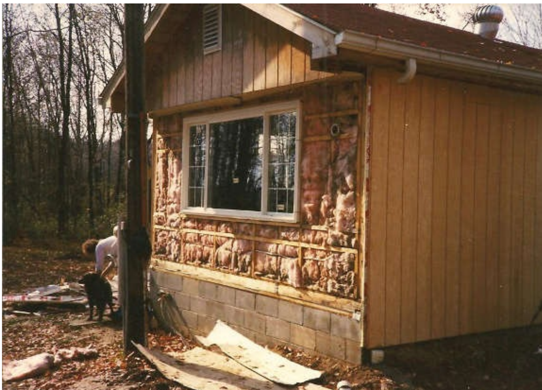
Removing the siding exposes the insulation. Photo credit: David and Mary.
