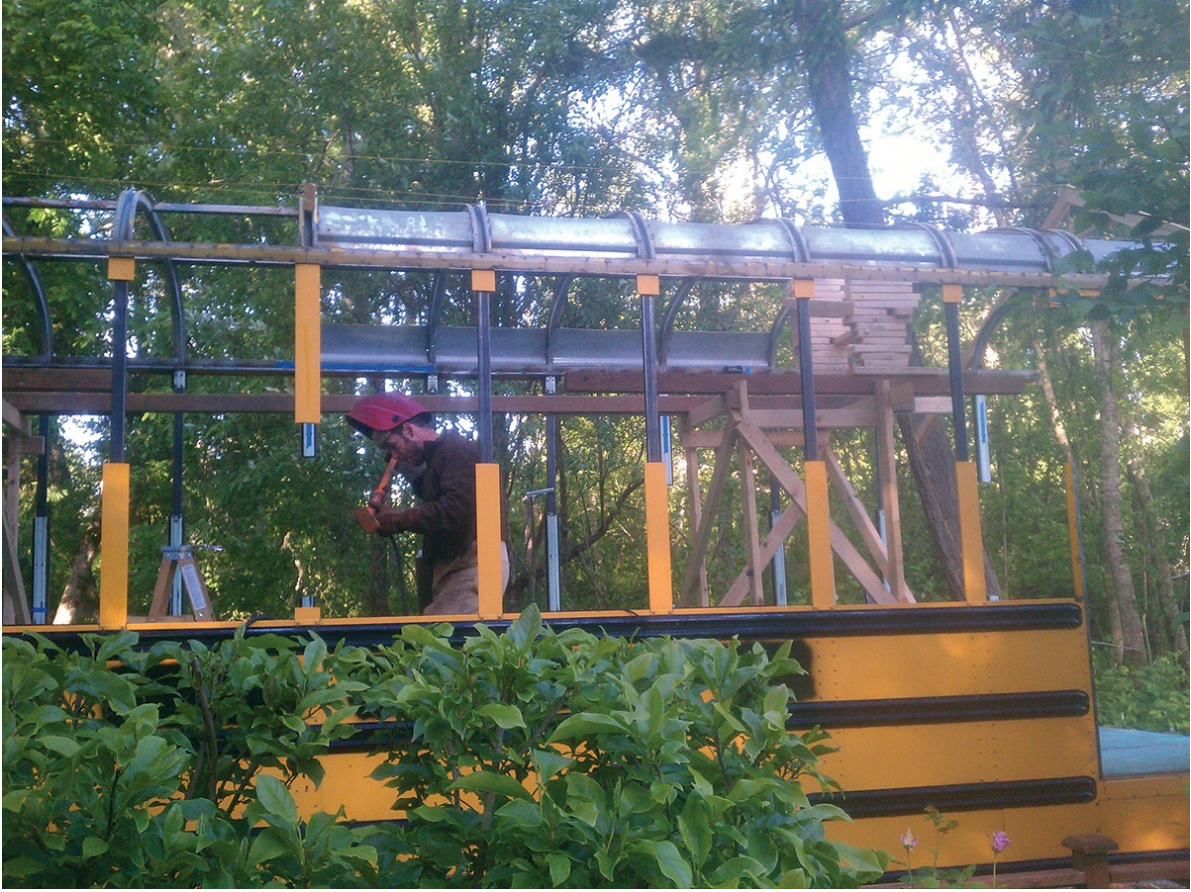
Raising the roof on the Thompson bus.
