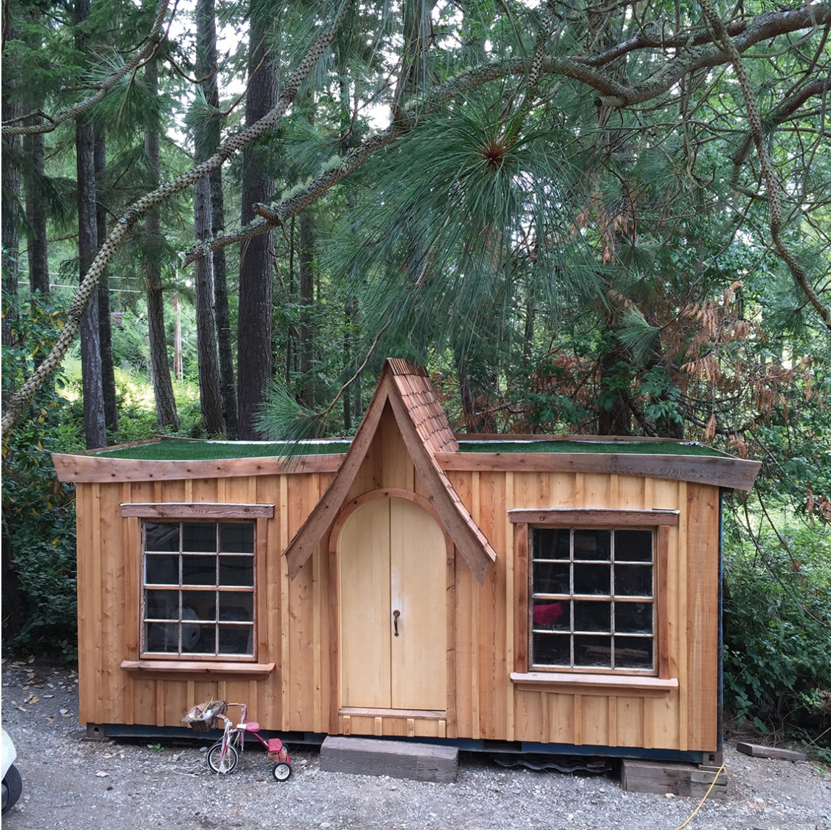
Jeremy's latest project is retrofitting a recycled shipping container into a cottage-style workshop. The structure sports the same whimsical, shingled aesthetic as the main house bus. It features an insulating green roof done with sod and a functional workshop interior.
