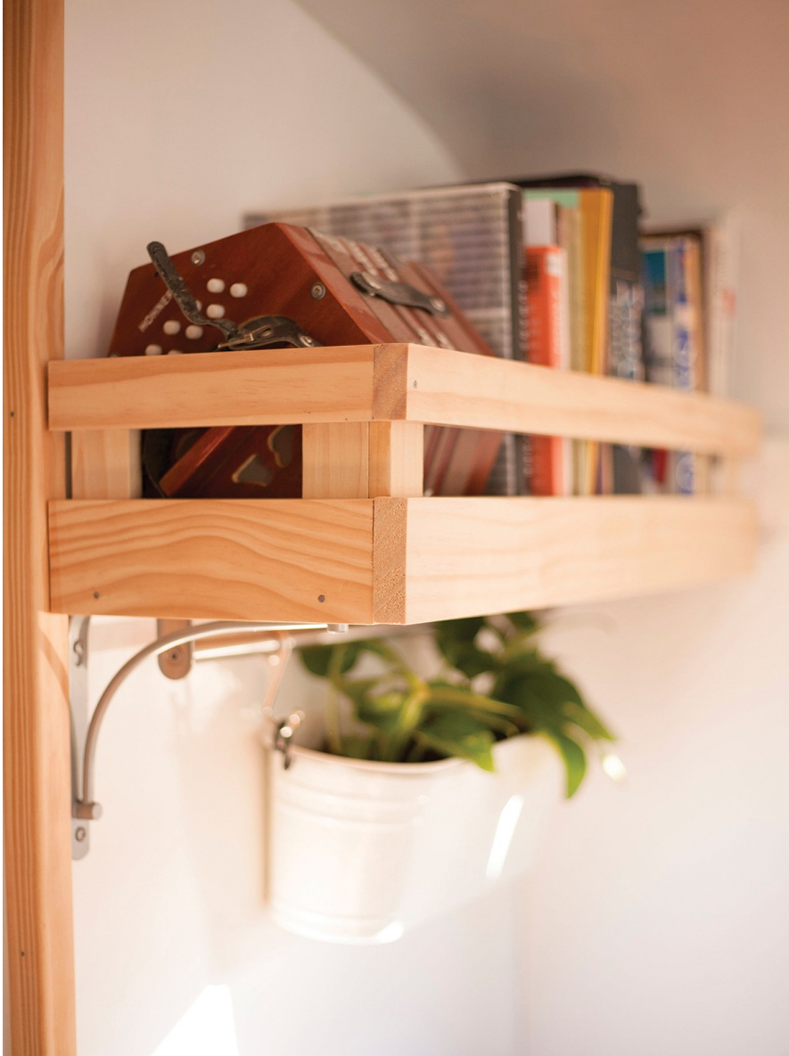
A set of bookcases is made from stacked milk crates and finished with pine boards. Wooden rods are inserted into the milk crate openings to keep books secure while the bus is in motion.
