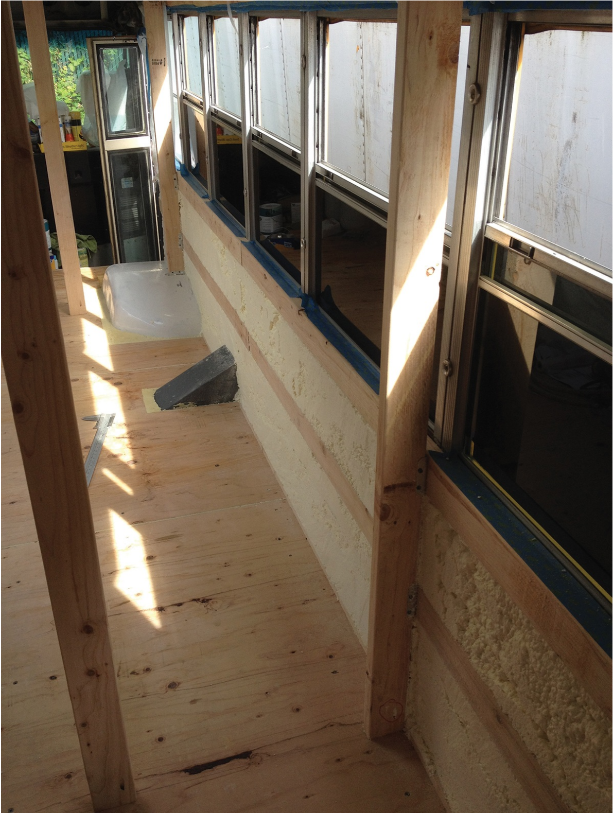
Spray foam insulation for Big Bertha.
