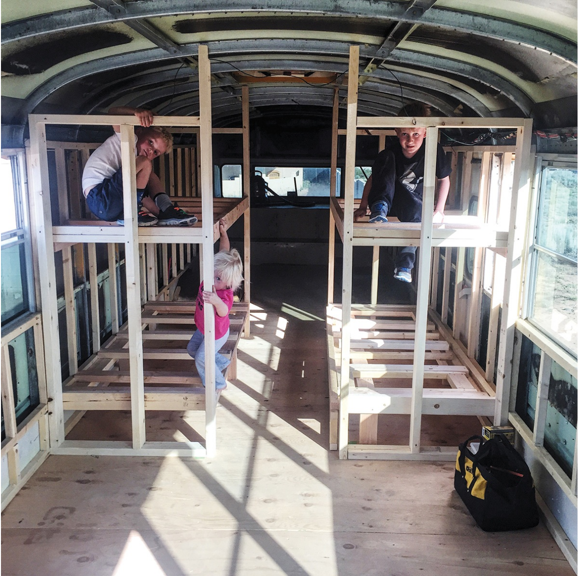
Framing out the children's bunk beds on the Trebitowskis' bus, Blue Steel.
