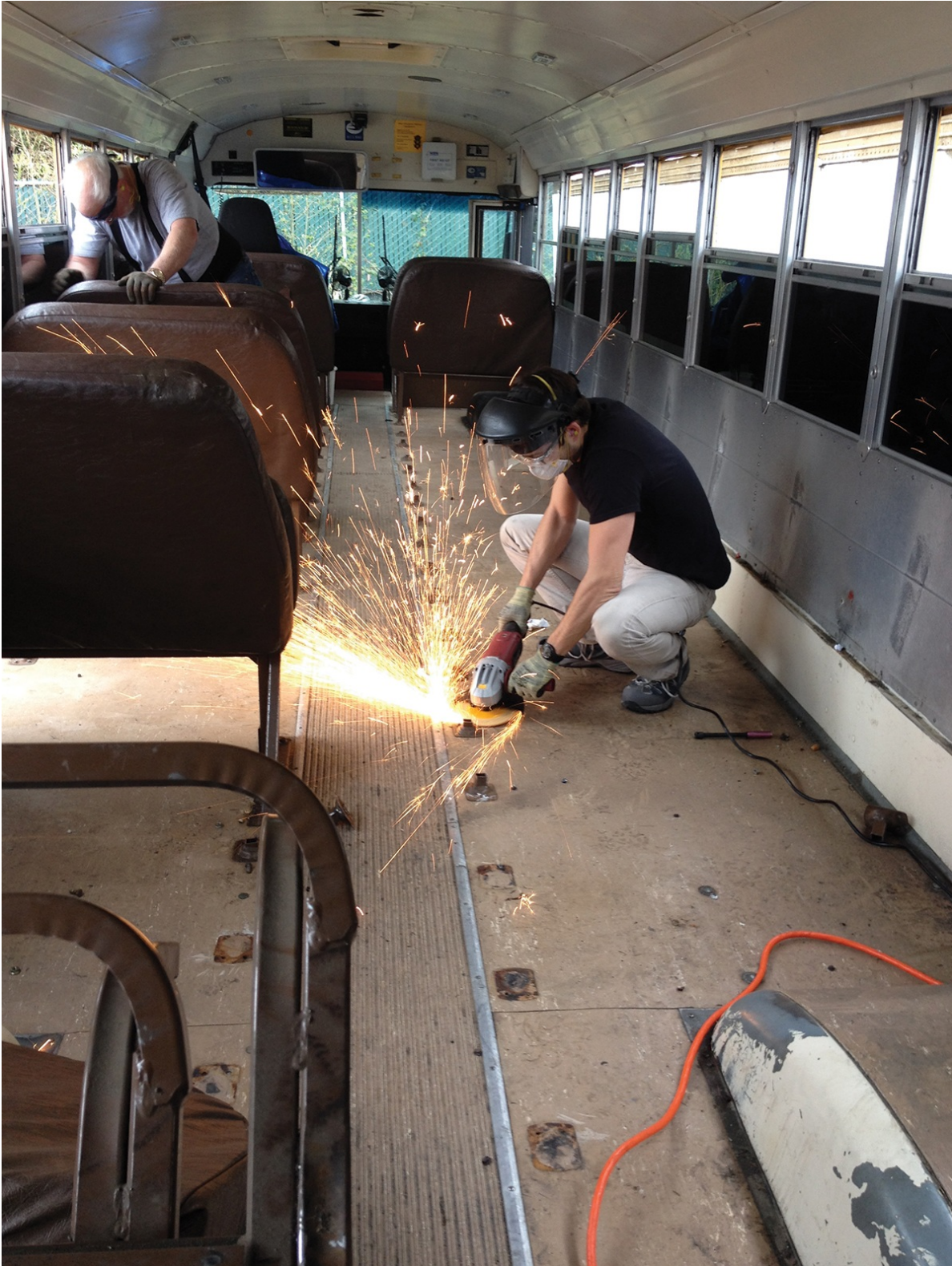
Removing seats on Big Bertha with an angle grinder.
