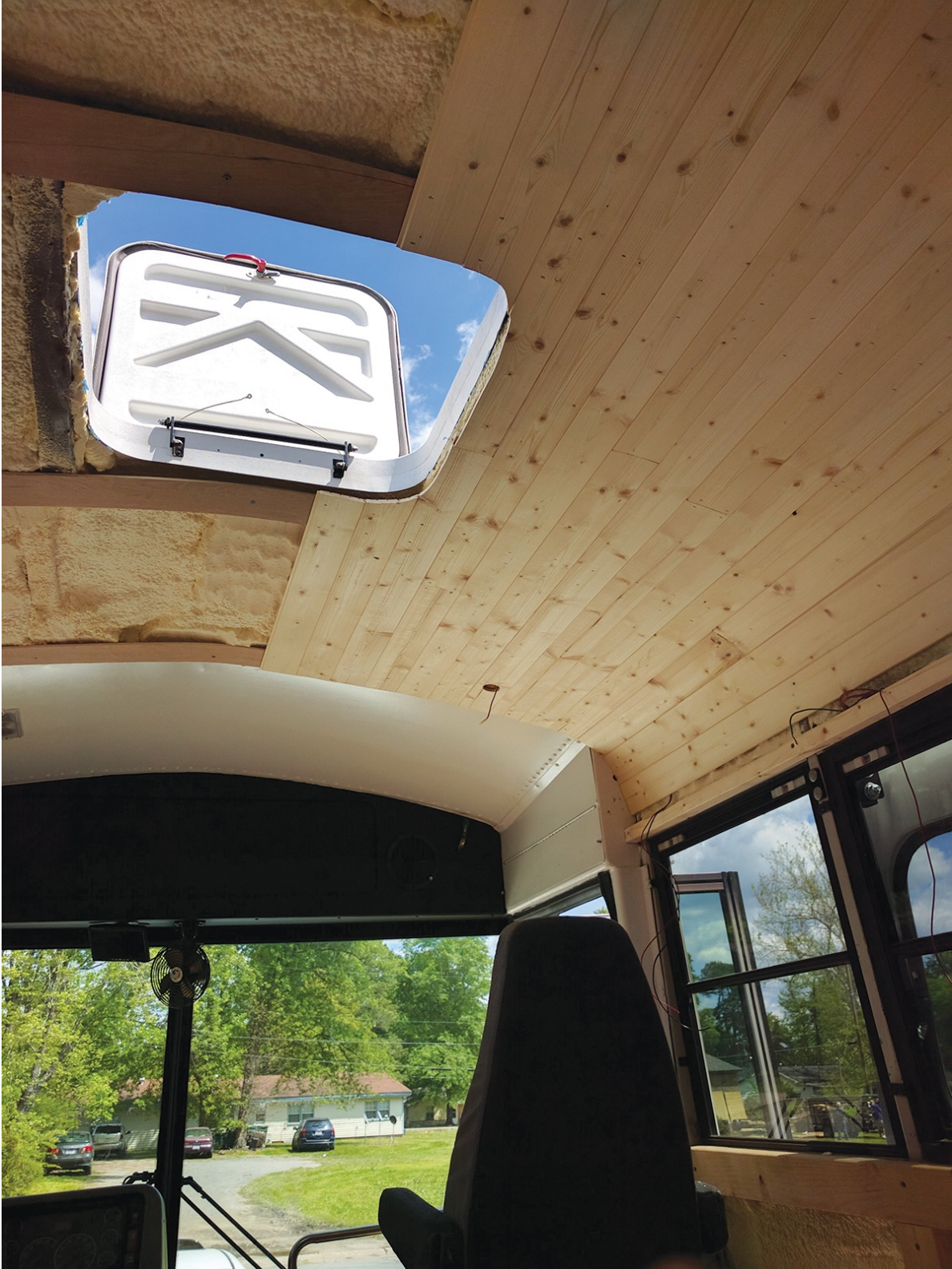
Wood siding is attached to wooden furring strips, which are in turn attached to the metal ribs on the roof of Zack Andrews and Annie King's bus, Stormy.
