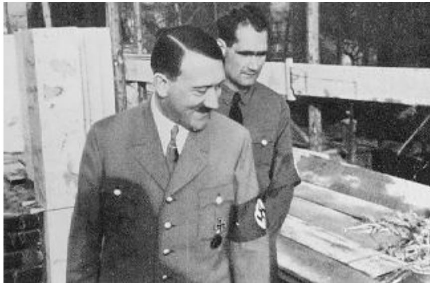
The Leader and Rudolf Heß inspect the construction of The Leader House in München.
