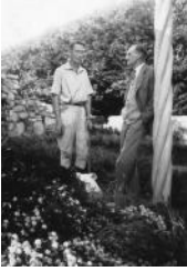
18. Robinson, Frederick Mortimer Clapp, and Haig Tor House courtyard, 1936
