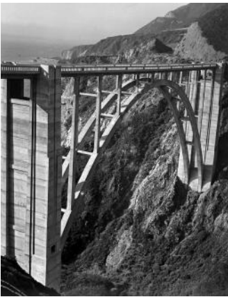
25. Bixby Bridge, Big Sur, 1937 Photograph by Julian P. Graham
