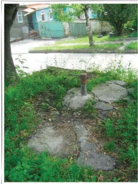
The hydrant to get water
