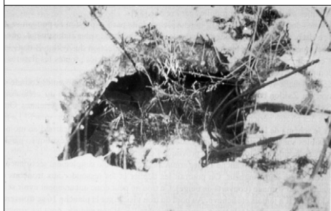
Illustration 7: Alleged Zyklon B input hatch in the ceiling of mortuary 1 (‘gas chamber’) of crematorium II. It is clearly visible that the reinforcing bars in the reinforced concrete were not even removed; they were merely bent back.
