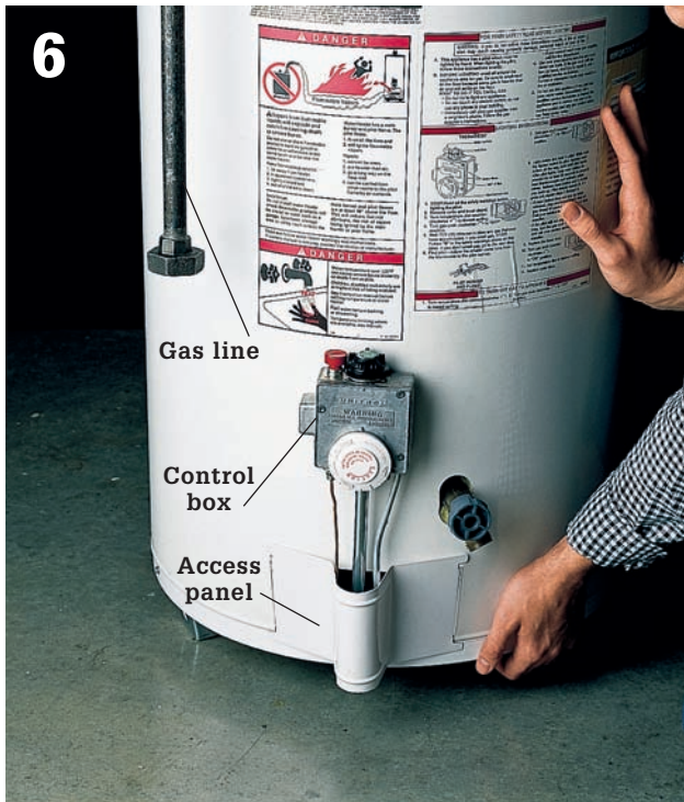
Position new heater so that control box is close to gas line, and access panel for burner chamber is not obstructed.
