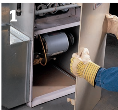
1 Remove the access panel to the blower housing and inspect the motor.
