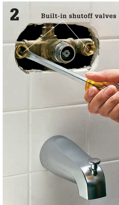
Turn off water supply at built-in shutoff valves or main shutoff valve.
