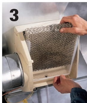
3 Remove the evaporator pad from the frame.
