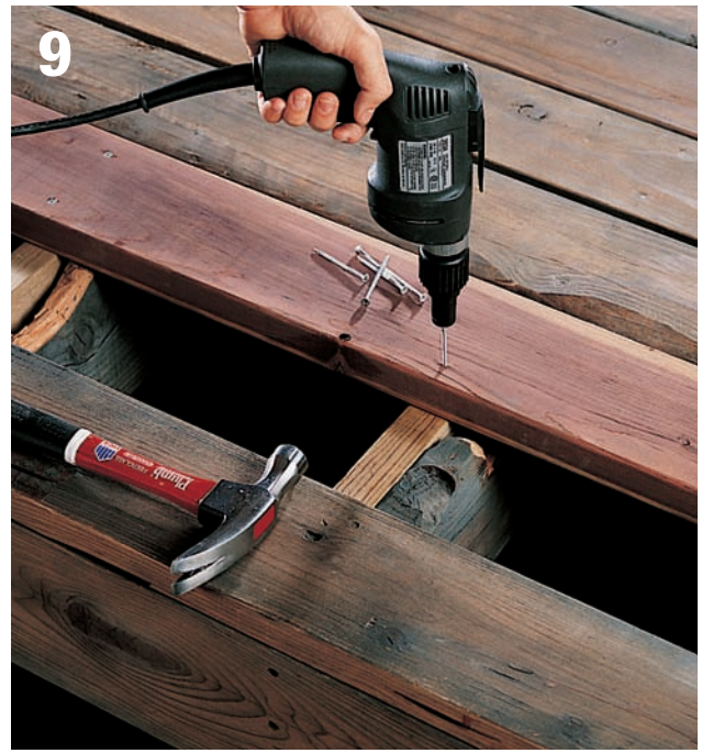
9 Position the new decking and attach to joists with galvanized deck screws or nails. Make sure space between boards matches that of existing decking.
