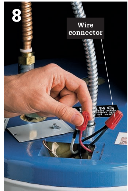
8 Connect the circuit wires to the water heater wires, using wire connectors.
