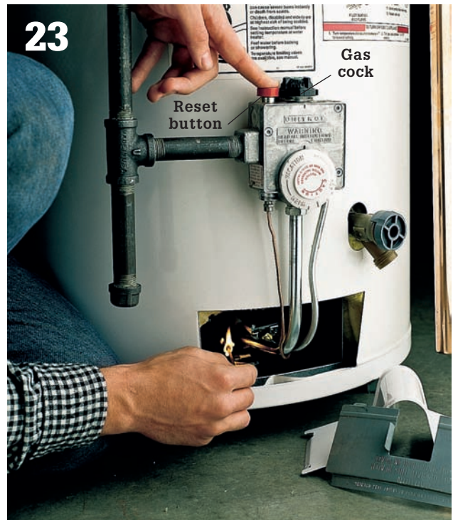
While holding match next to end of pilot gas tube , press the reset button on top of control box. When pilot flame lights, continue to hold reset button for one minute. Turn gas cock to ON position, and replace the inner and outer access panels.
