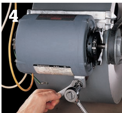
4 Loosen the pulley tension adjustment nut slightly to tighten the belt.
