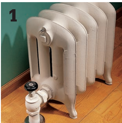
Hot-water radiators circulate heated water through pipes. As it cools, water is drawn back to the boiler for reheating.
