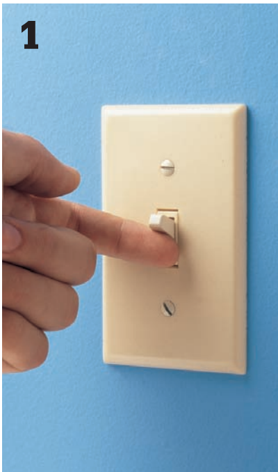
Switch on all light fixtures. Remember to turn on closet lights, basement lights, and exterior lights.
