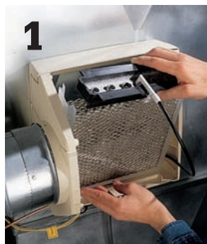
1 Remove the distribution tray from the humidifier.
