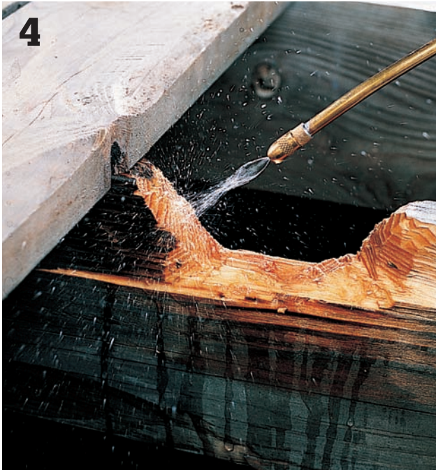
4 Apply a thick coat of sealer-preserved to damaged joist. Let dry, then apply a second coat of sealer. Cut a reinforcing joist (sister joist) from pressure-treated lumber.
