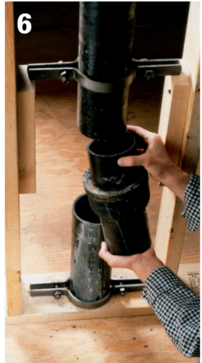
6 Repeat cutting at the other chalk line. Remove cut section of pipe.
