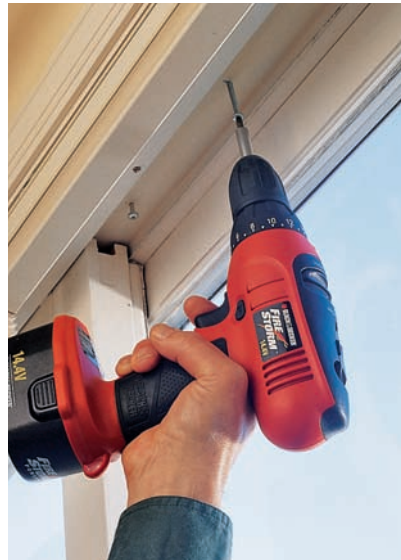
Drive screws into the upper track to keep the sliding panel from being pried up and out of the lower track. Use sturdy pan-head screws, spaced about every 8", and drive them so their heads just clear the top of the door. For metal door frames, use self-tapping screws and a low drill speed.
