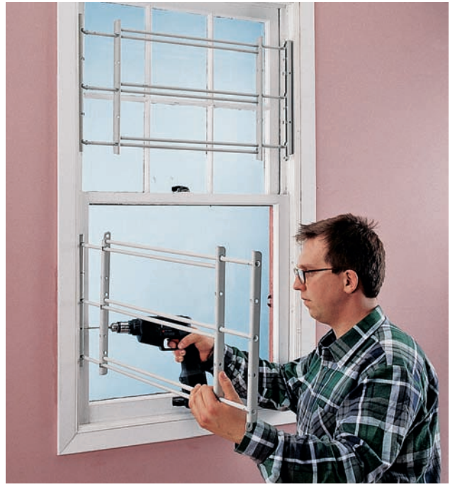
Security bars or gates can be installed in ground-floor windows to prevent intruders from gaining entry to your home.
