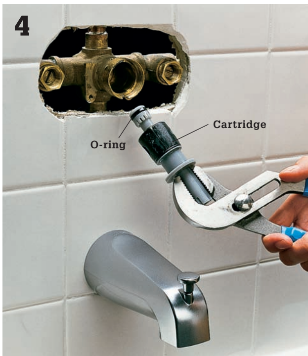
Remove cartridge assembly by grasping end of valve with channel-type pliers and pulling gently.
