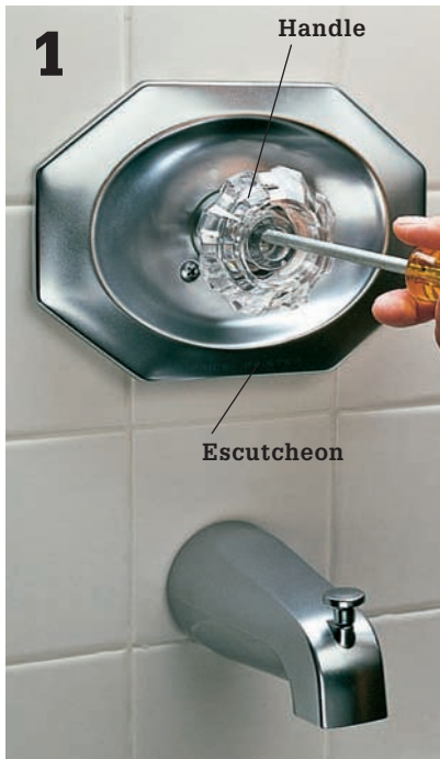
Use a screwdriver to remove the handle and escutcheon.
