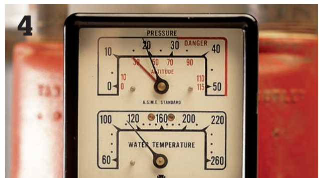
4 The boiler should reach a pressure of 20 psi before you turn the power back on.
