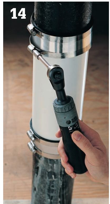
14 Tighten the screw clamps with a ratchet wrench or screwdriver.
