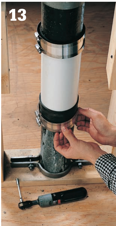
13 Slide stainless steel bands and clamps over the neoprene sleeves.
