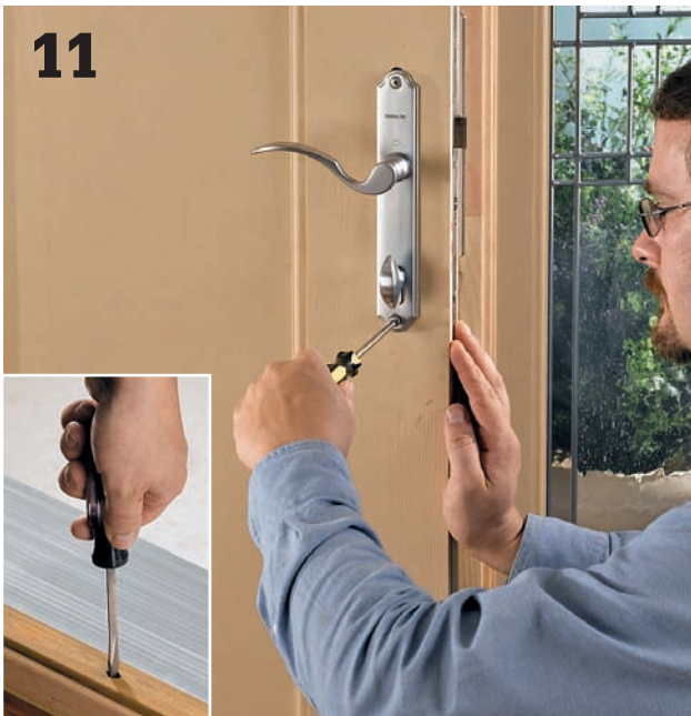
11 Install the lockset , strikeplates, deadbolts or multipoint locks, and any other door hardware. If the door finish has not been applied, you may want to do so first, but generally it makes more sense to install the hardware right away so the door can be operated and locked. Attach the door sill to the threshold and adjust it as needed, normally using the adjustment screws (inset).
