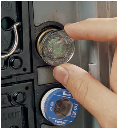
Shut off power to the proper circuit at the fuse box or main service panel before beginning work.
