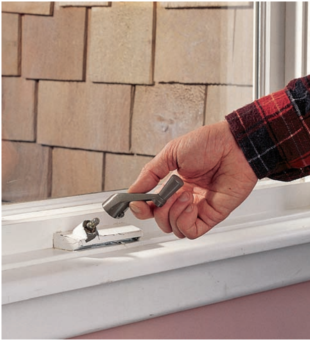
Removing the handles from casement and awning windows keeps intruders from cranking the window open after breaking the glass.
