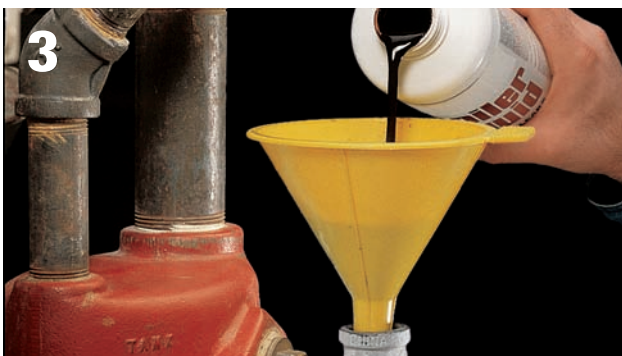
3 Using a funnel, add a recommended rust inhibitor to the boiler through the valve or gauge fitting.
