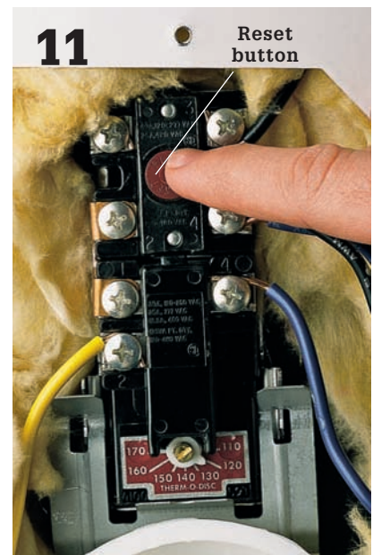
11 Press reset button on thermostats. Replace the insulation and access panels. Turn on power.
