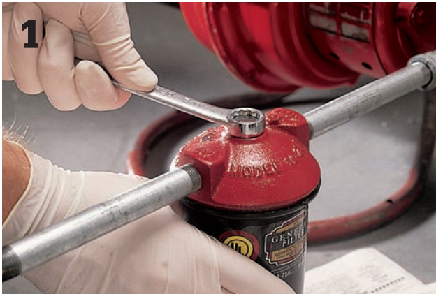
1 Have a disposable plastic bag ready, and unscrew the top of the filter cartridge.
