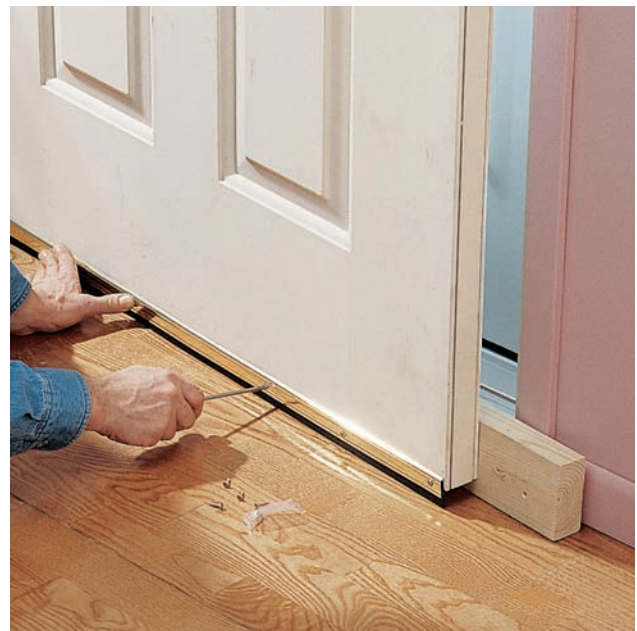
A felt door sweep can seal out drafts, even if you have an uneven floor or a low threshold.
