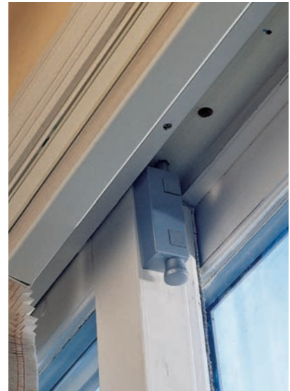
Attach a sliding-door lock to the frame of the sliding panel. Drill a hole for the deadbolt into the upper track. Then drill an additional hole a few inches away so you can lock the door in an open position.
