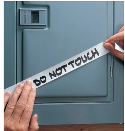
Close service panel door and post a warning sign to prevent others from turning on power while you are working on electrical projects.
