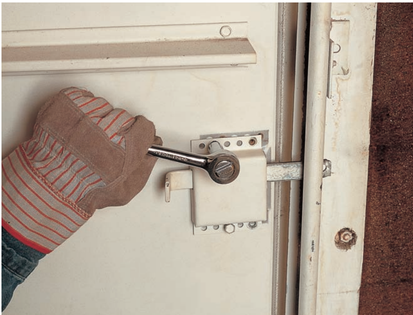
Alternative: Sometimes the lock bar won't lock the door because it won't slide into its opening on the door track. To fix this, loosen the guide bracket that holds the lock bar and move it up or down until the bar hits the opening.
