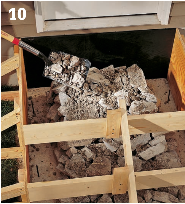
10 Fill the form with clean fill (broken concrete or rubble). Stack the fill carefully, keeping it 6" away from the sides, back, and top edges of the form. Shovel smaller fragments onto the pile to fill the void areas.
