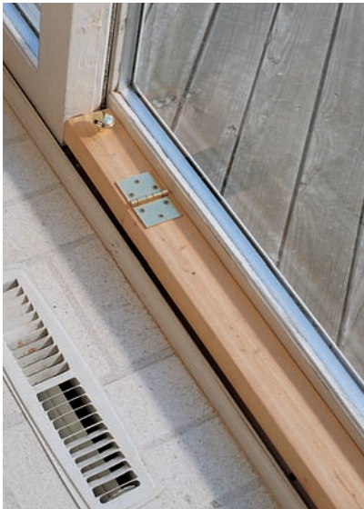
Make a custom lock for your door track, using a thick board and a hinge. Cut the board to fit behind the closed door, then cut it again a few inches from one end. Install a hinge so you can flip up the end and keep the door secure while it's ajar. Attach knobs to facilitate use.
