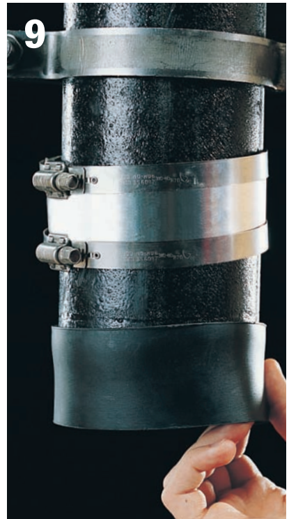
9 Make sure the cast iron pipe is seated snugly against the rubber separator ring molded into the interior of the sleeve.
