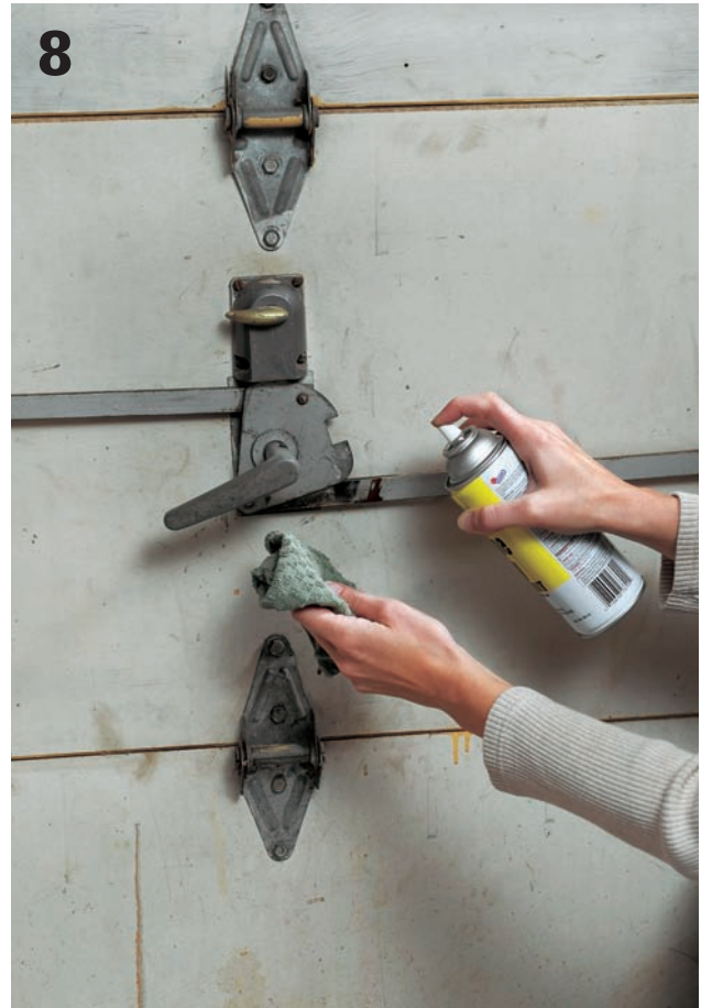
8 If a latch needs lubrication, use graphite in powder or liquid form. Don't use oil because it attracts dust that will clog the lock even more.
