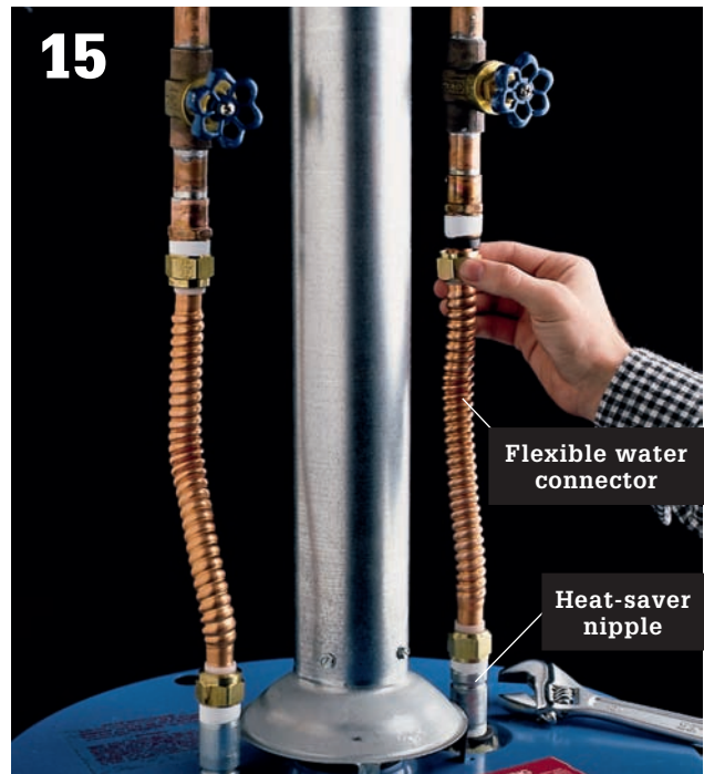
Connect the water lines to the heat-saver nipples with flexible water connectors. Tighten fittings with an adjustable wrench.
