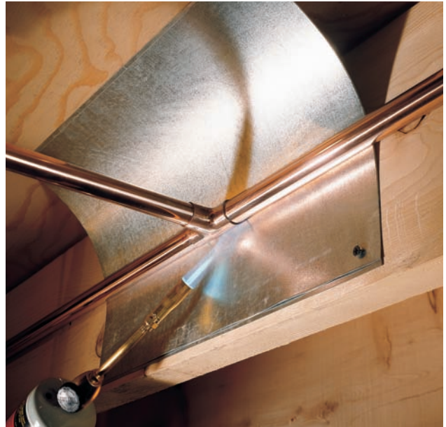
Protect wood from heat of the torch flame while soldering, using a double layer (two 18" × 18" pieces) of 26-gauge sheet metal. Buy sheet metal at hardware stores or building supply centers and keep it to use with all soldering projects.
