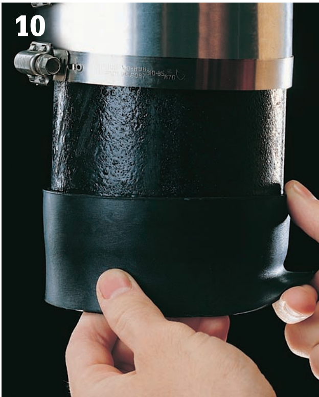
10 Fold back the end of each neoprene sleeve, until the molded separator ring on the inside of the sleeve is visible.
