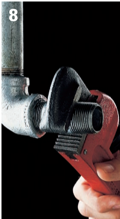
8 Screw first nipple into fitting, and tighten with pipe wrench.
