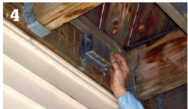
Remove any debris and materials that could block the air intake and exhaust.
