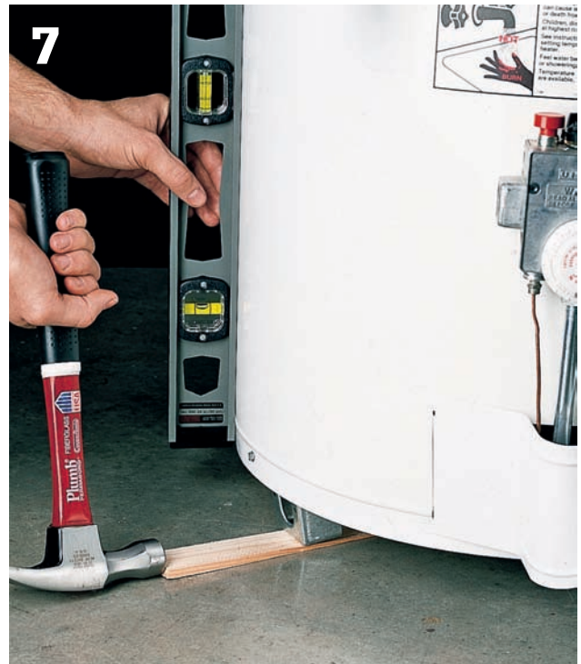
Level the water heater by placing wood shims under the legs.
