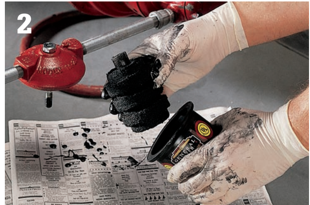
2 Twist the cartridge to remove it from the oil supply line. Ask your waste removal company for disposal instructions.
