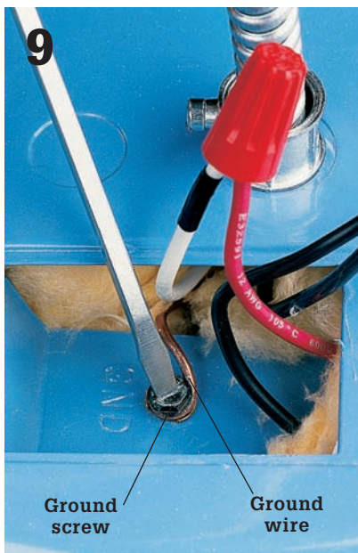
9 Attach bare copper or green ground wire to ground screw. Replace coverplate.
