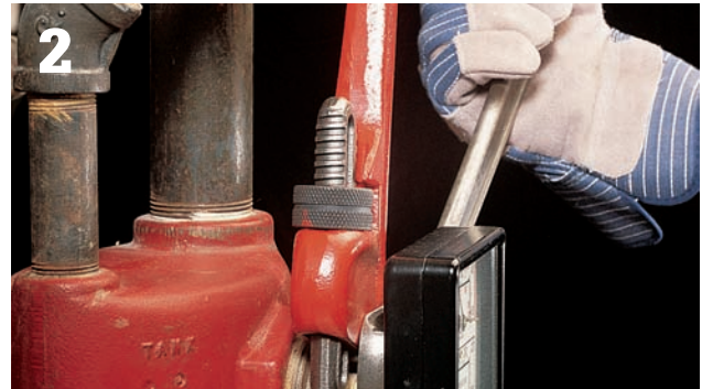
2 If the valve or gauge on top of the boiler is attached to a separate fitting, hold the fitting still with one wrench while removing the valve or gauge with another.
