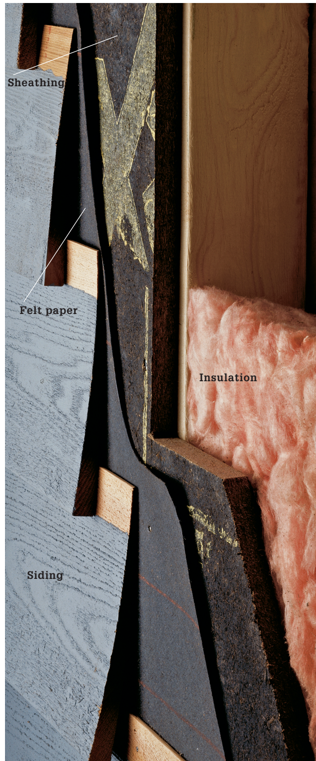
The exterior wall is composed of siding, housewrap or felt paper, and sheathing. Remove the siding without disturbing or damaging the sheathing.
