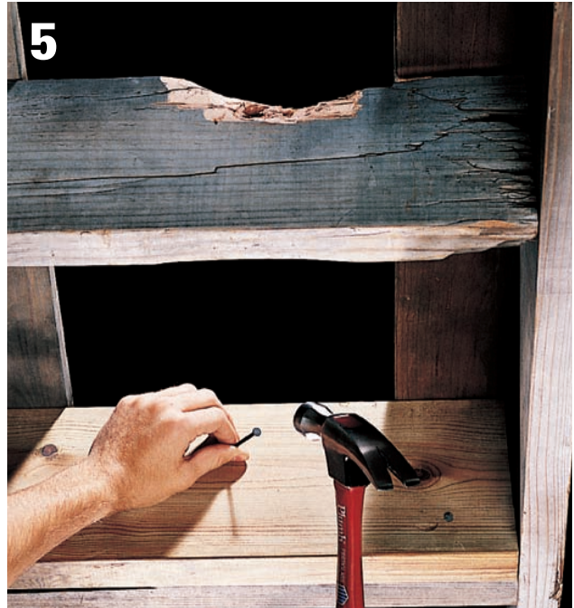
5 Treat all sides of sister joist with clear sealer-preserved, and let dry. Position sister joist tightly against the damaged joist, and attach with 10d nails driven every 2 feet.
