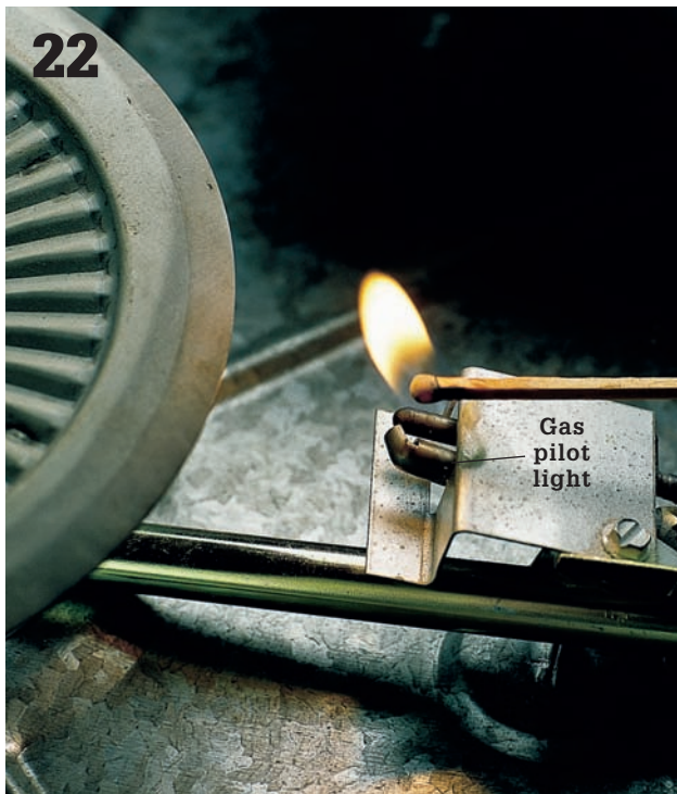
Light a match and hold flame next to the end of the pilot gas tube inside the burner chamber. Be sure to keep your face away from the opening.
