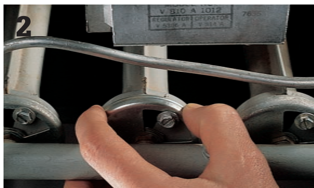
2 If the shutters are adjustable, you can set them yourself. Otherwise, call a professional for service.
