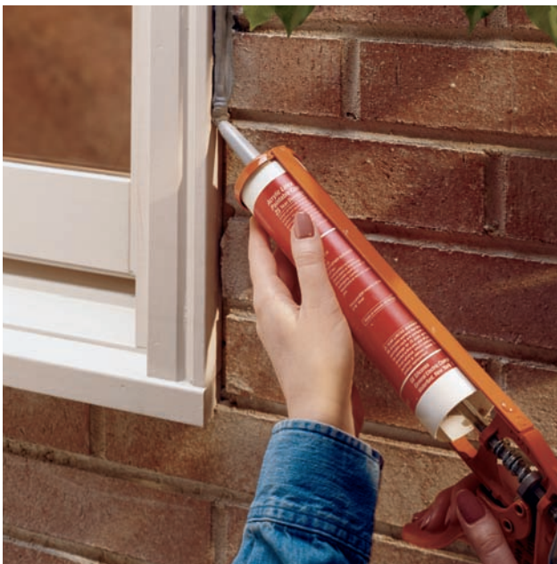
Use a caulk that matches your home exterior to seal the window and door frames.
