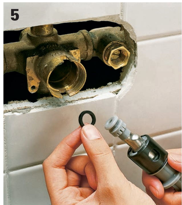
Flush valve body with clean water to remove sediment. Replace any worn O-rings. Reinstall cartridge and test valve. If faucet fails to work properly, replace the cartridge.
