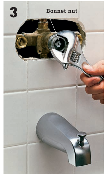
Unscrew and remove retaining ring or bonnet nut, using an adjustable wrench.
