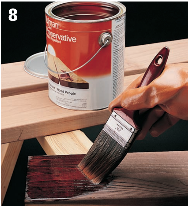
8 Apply a coat of sealer-preserved or staining sealer to all sides of the new decking boards.
