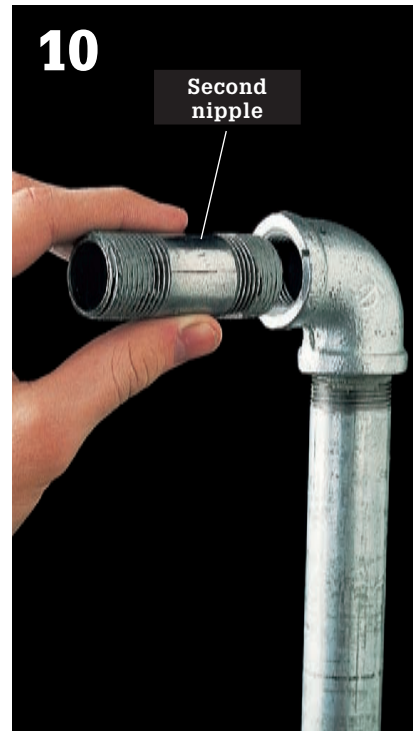
10 Screw second nipple onto other fitting. Tighten with a pipe wrench.
