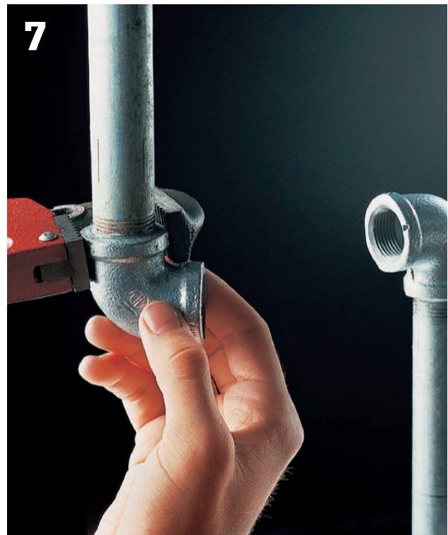
Screw new fittings onto pipe threads. Tighten fittings with two pipe wrenches, leaving them about 1/8 turn out of alignment to allow assembly of union.
