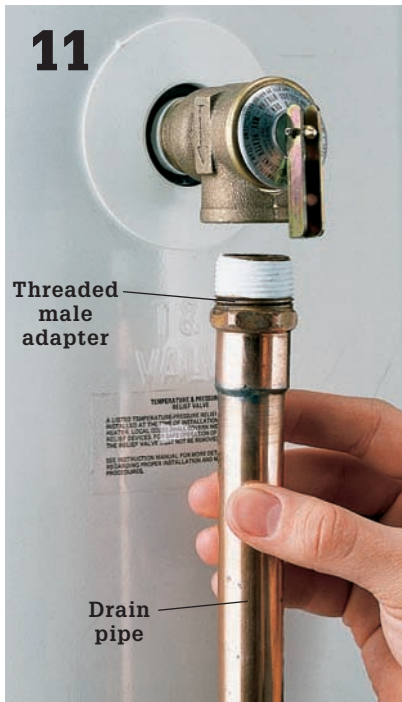
Attach a copper or CPVC drain pipe to the pressure-relief valve, using threaded male adapter. Pipe should reach to within 3" of floor.
