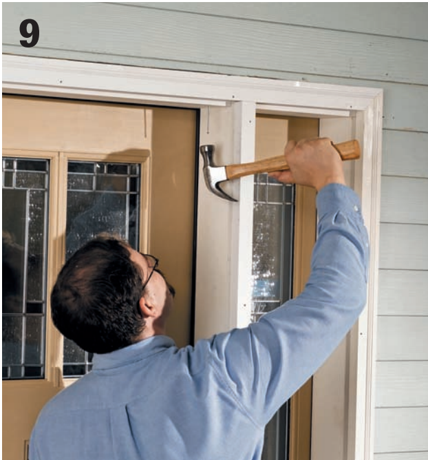
9 Drive finish nails at all remaining locations, following the nailing schedule in the manufacturer's installation instructions.
