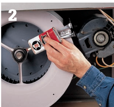
2 Remove the covers to the oil ports and add a few drops to each port.
