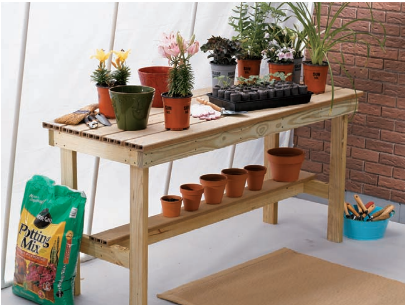
This potting bench has a 28 × 71" top and is built with four 2 × 4s and three standard-size decking boards. The handy pot shelf below the bench top is made with a cutoff from one of the deck boards.
