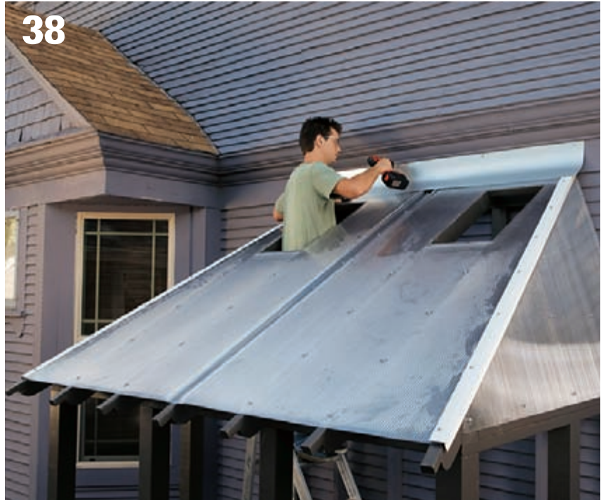
38 Cover the gap between the standalone greenhouse structure and the house with metal flashing. Aluminum handy flashing (12" width) can be fastened to the house and lightly creased so it extends over the gap and forms a seal without any physical connection to the greenhouse.
