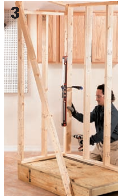
3 Fasten the wall frames. Attach the shed walls to one another and to the base platform with 2½" screws. Use a square and level to check that the walls are plumb and square.
