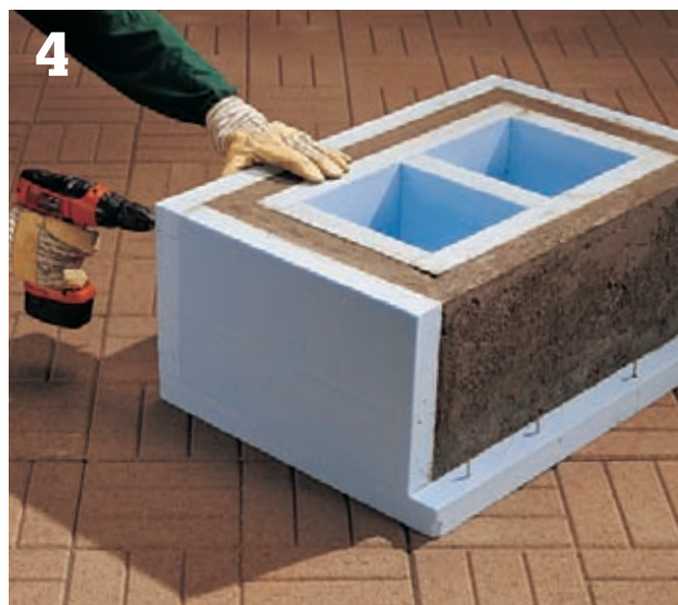
After the planter has dried for 48 hours, remove the screws and carefully disassemble the forms.
