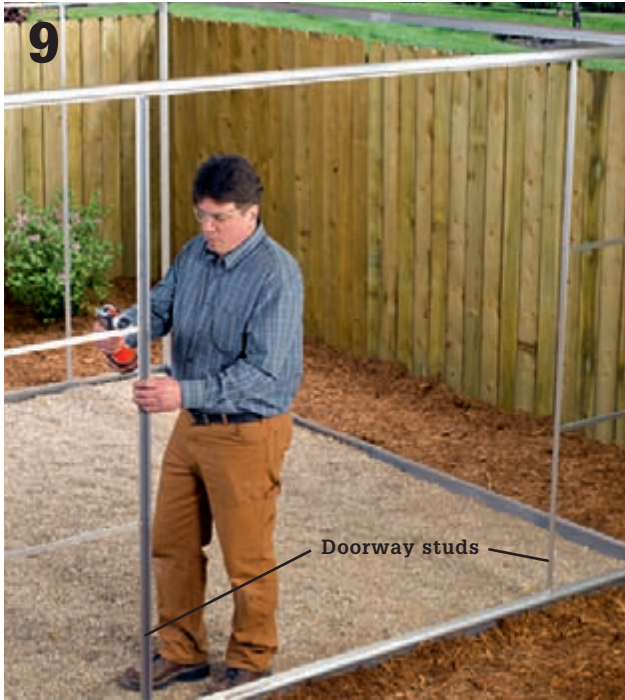
9 Install the doorway studs at either side of the greenhouse door, on the front end of the building. Install the side studs along both side walls of the greenhouse.
