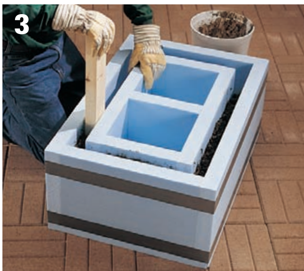
Center the inner form within the outer form, and then tamp hypertufa between the two, forming the walls.
