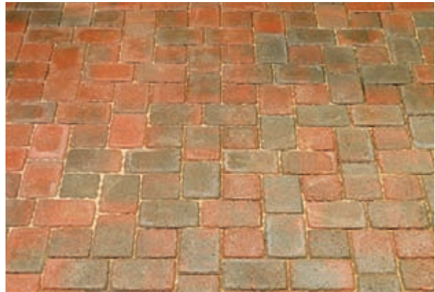
Concrete pavers set in sand offer a longlasting, stable floorcovering that breathes and allows for good drainage.
