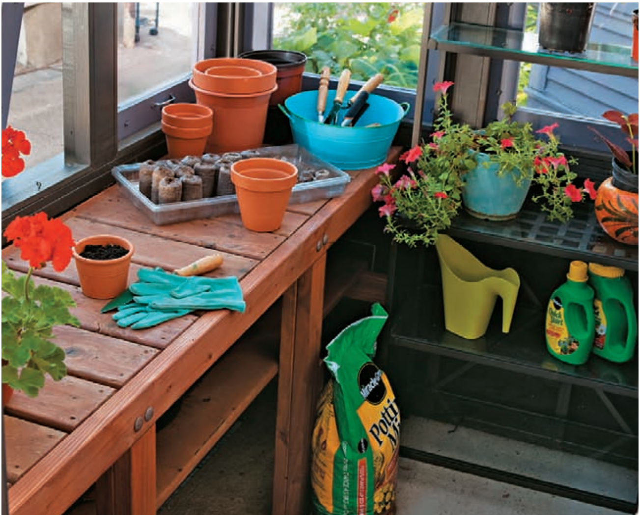
This potting bench uses the structural members of a greenhouse kneewall for support. The five slats at the right end can be removed to access a shelf for buckets and planters.
