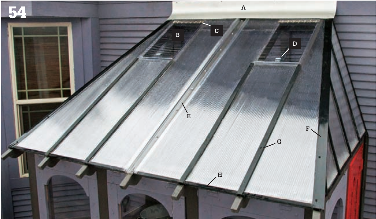
54 Add trim elements to complete the roof. Parts of the roof trim system include: Flashing over ridge (A); Clear vent panel (B) attached with piano hinge (C) and automatic closer (D); Seaming strip (E); Metal drip cap for edges (F); ¼ x 1½" wood battens at rafter locations (G); vinyl cap molding at eave edges (H).
