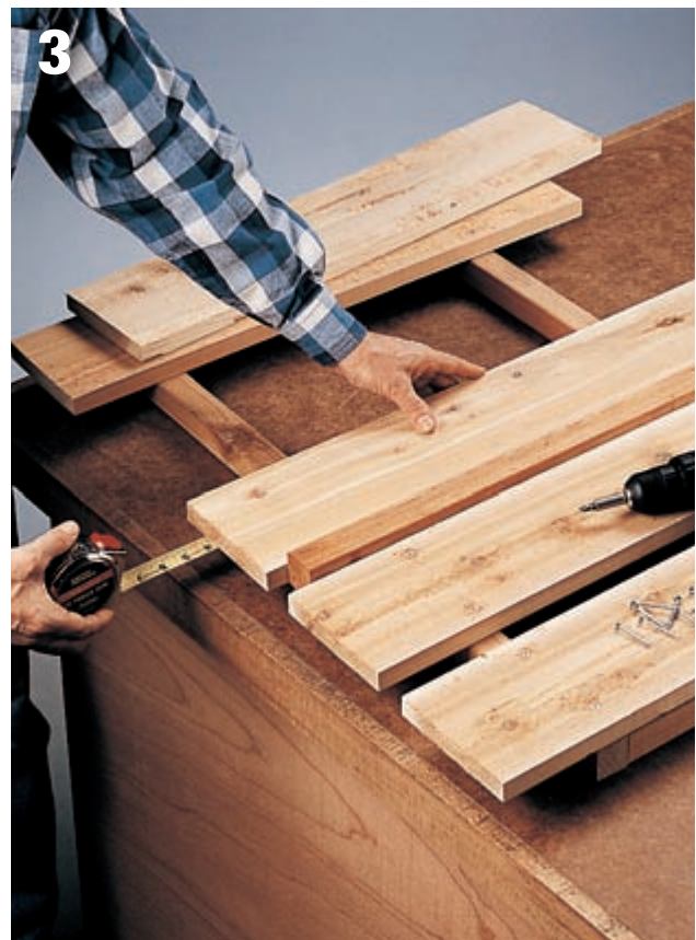
Continue to attach slats. The inner slats should be 1\frac{1}{2} " apart, with the ends 4" below the bottom of the frame.
