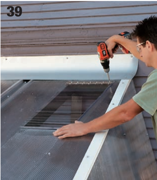
39 Install roof vent covers. (Here, the installation of the covers was postponed to allow access through the vent holes for installing flashing.) Use a piano hinge to attach each roof vent cover to the roof.
