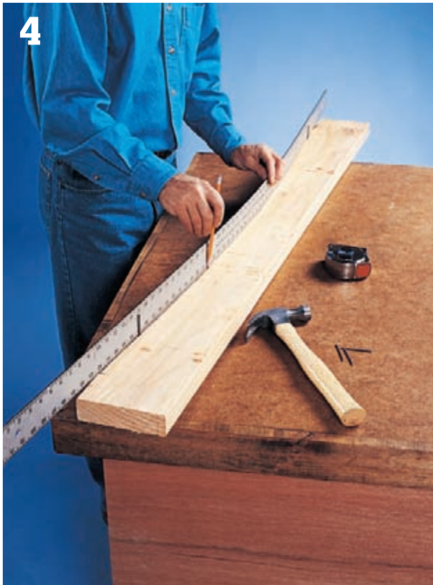
4 Mark the profile cuts on the aprons. Use a flexible ruler pinned between casing nails to trace a smooth arc.
