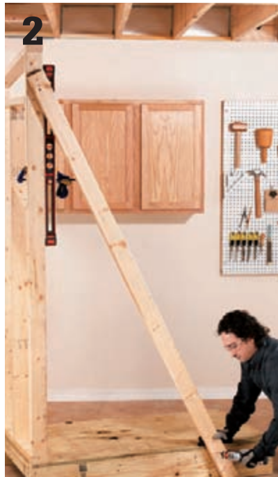
2 Raise the walls. Use a scrap of wood as a brace to keep the wall plumb. Attach the brace to the side-wall frame and to the base platform once you have established that the wall is plumb.
