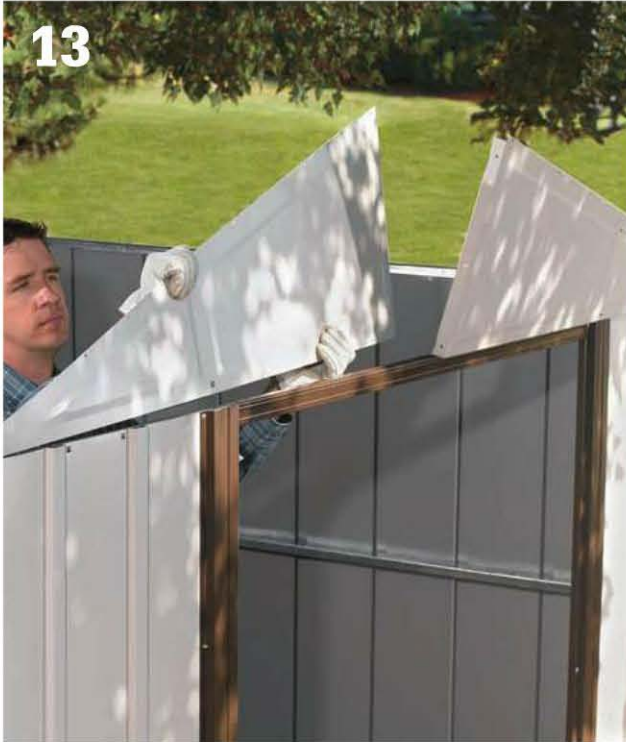
13 Insert the shed gable panels into the side frames and the door track and slide them together so the fastener holes are aligned. Attach the panels with the provided fasteners.
