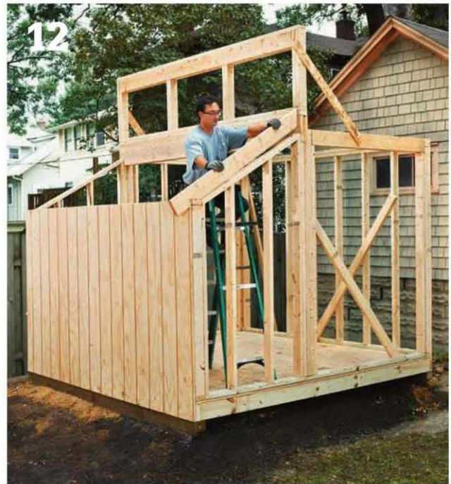
12 Cut one of each "A" and "B" pattern rafters from a single 16-ft. 2 × 6, using the RAFTER TEMPLATES (page 94). Both roof planes have a 6-in-12 slope. Test-fit the rafters and make any necessary adjustments, then use the patterns to cut eight more rafters of each type. Install the rafters as shown in the REAR FRAMING and FRONT FRAMING (page 91). Toenail the top ends of the "B" rafters to the main header.
