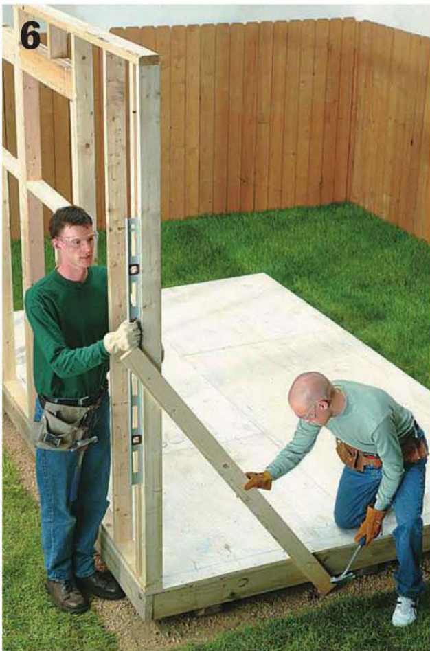
Nail the bottom plate to the floor frame , then plumb the wall and secure it with end braces.
