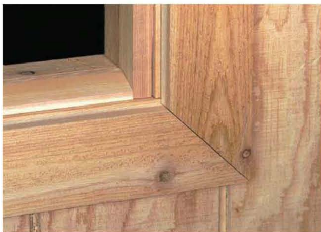
Window trim with miter joints
