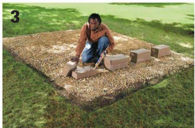
Bind stacked blocks together with exterior-rated construction adhesive to prevent shifting.
