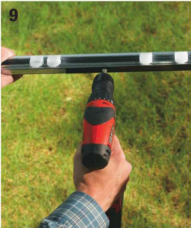
9 Attach the moving and nonmoving parts for the upper door track to the side frames if your shed has sliding doors.
