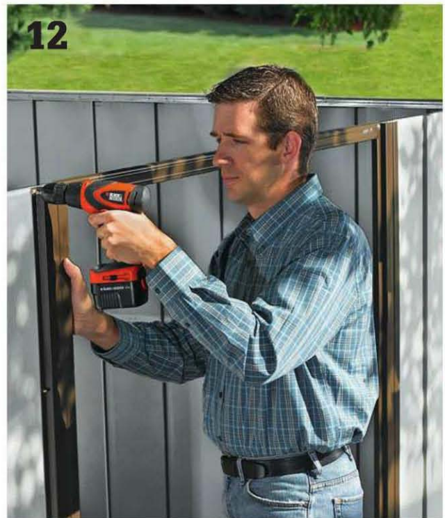
12 Fasten the doorframe trim pieces to the frames to finish the door opening. If the fasteners are colored to match the trim, make sure you choose the correct ones.
