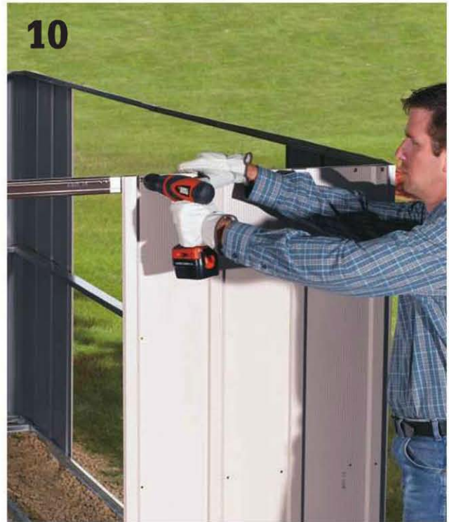
10 Fasten the shed panels to the top frames , making sure to that any fasteners holes are aligned and that crimped tabs are snapped together correctly.
