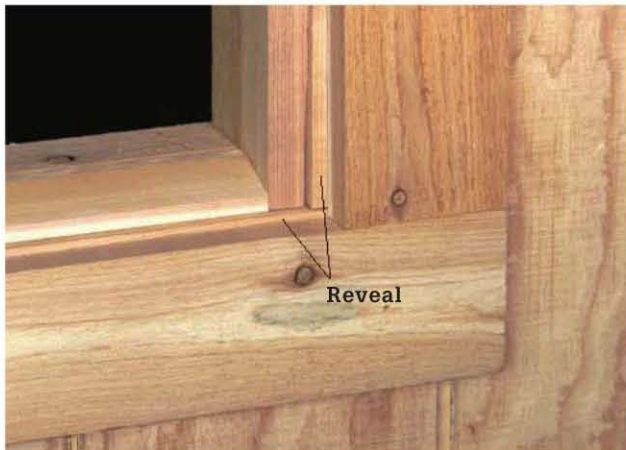
Window trim with butt joints
