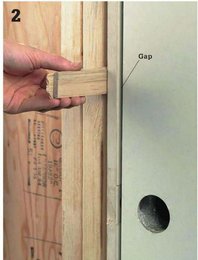
Shim the latch jamb , using the gap between the door and the jamb as a gauge. Make sure the gap is consistent.
