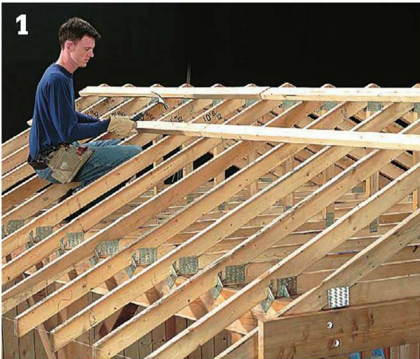
Install the purlins across the rafters, then add blocking at the gable ends.
