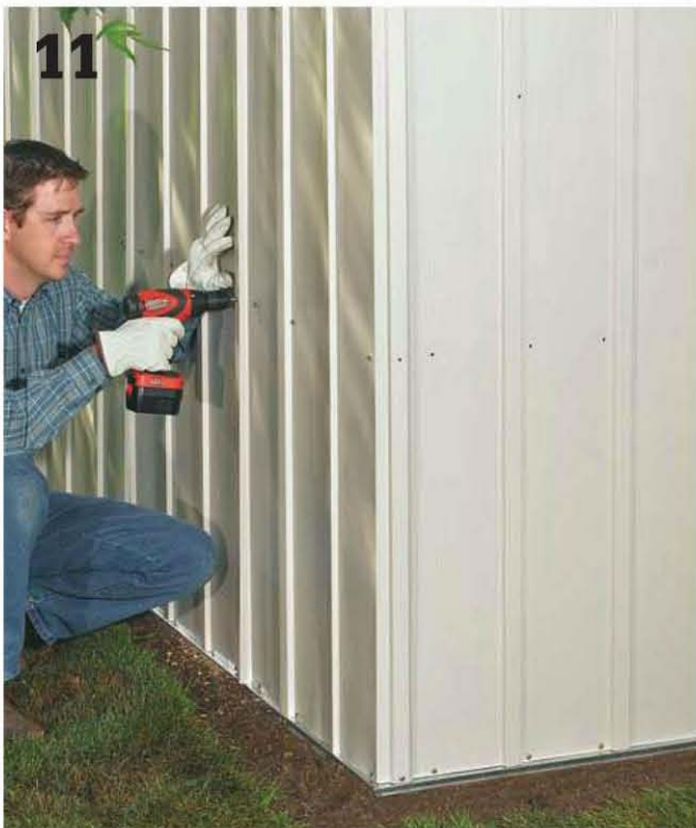
11 Fill in the wall panels between the completed corners, attaching them to the frames with the provided fasteners. Take care not to overdrive the fasteners.
