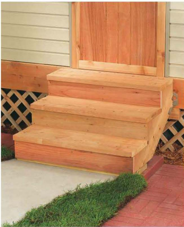
Option: Add riser boards to enclose each step.
