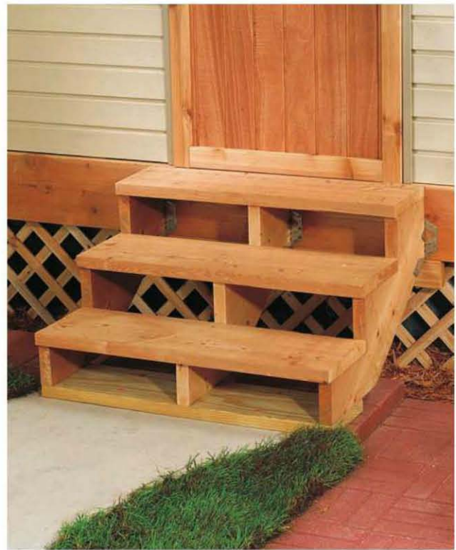
Option: Leave off riser boards for an open staircase.
