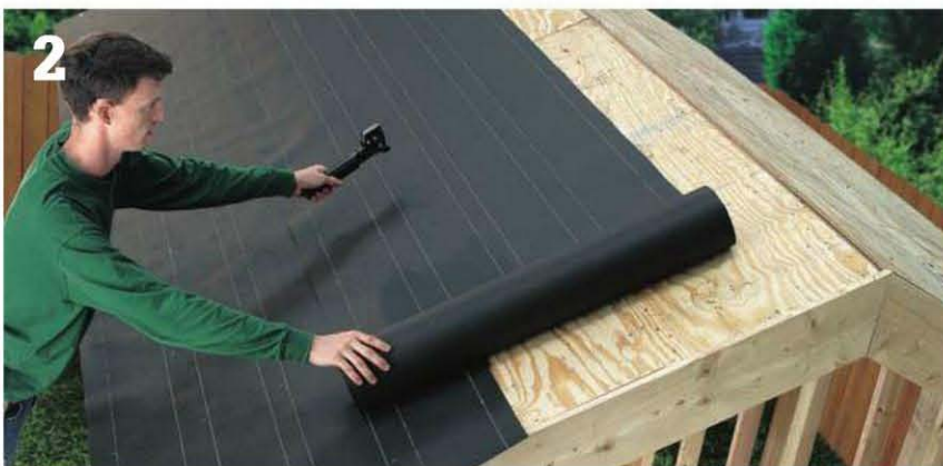
Apply building paper from the bottom up, so the lower paper is overlapped by the paper above it.
