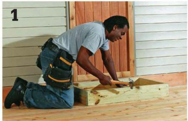
Assemble the frame pieces with pairs of 16d common nails.
