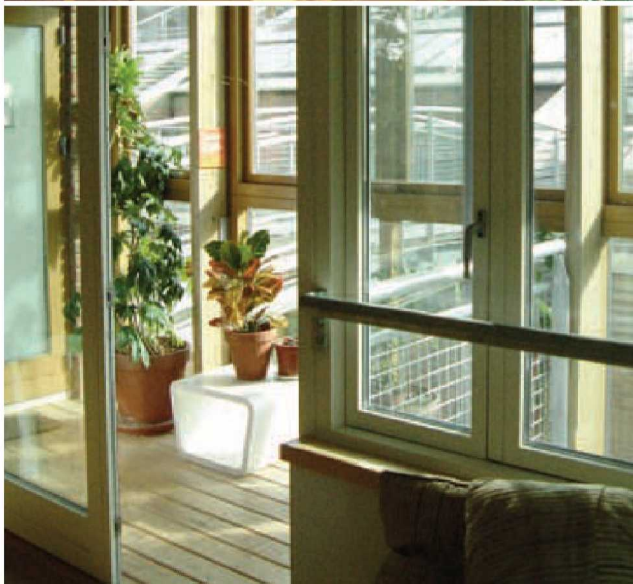
Top: A lobby reduces heat loss, and acts as an airlock. Middle: This conservatory is single-glazed, but has an insulated roof to reduce heat loss and overheating in summer. Bottom: This sunspace provides passive solar heat gain.
