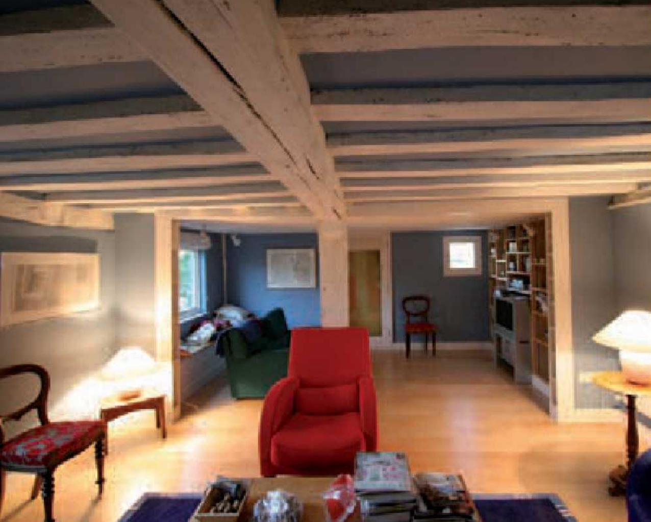
Left: The original house was stripped back to the timber frame and restored. Right: The recent bedroom extension is built using hemp.
