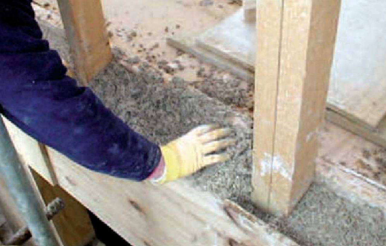
Left: Walls are constructed by packing a mix of lime and hemp into formwork to fully enclose the timber frame. Right: The hemp/lime mix is built up to the underside of the roof, which forms an airtight construction.
