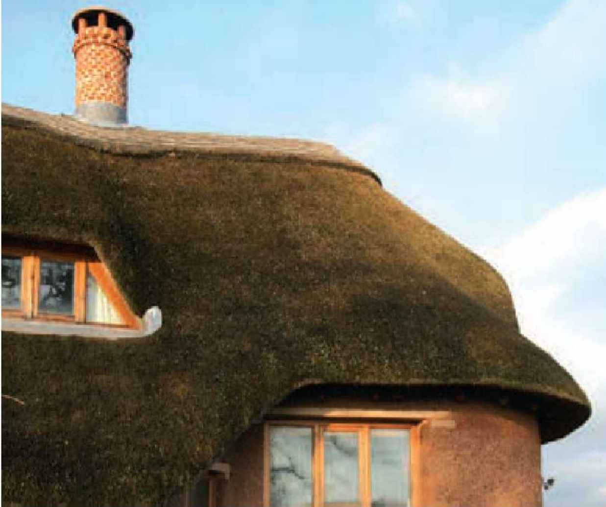
Thatch is a renewable roofing material with moderate insulating properties.
