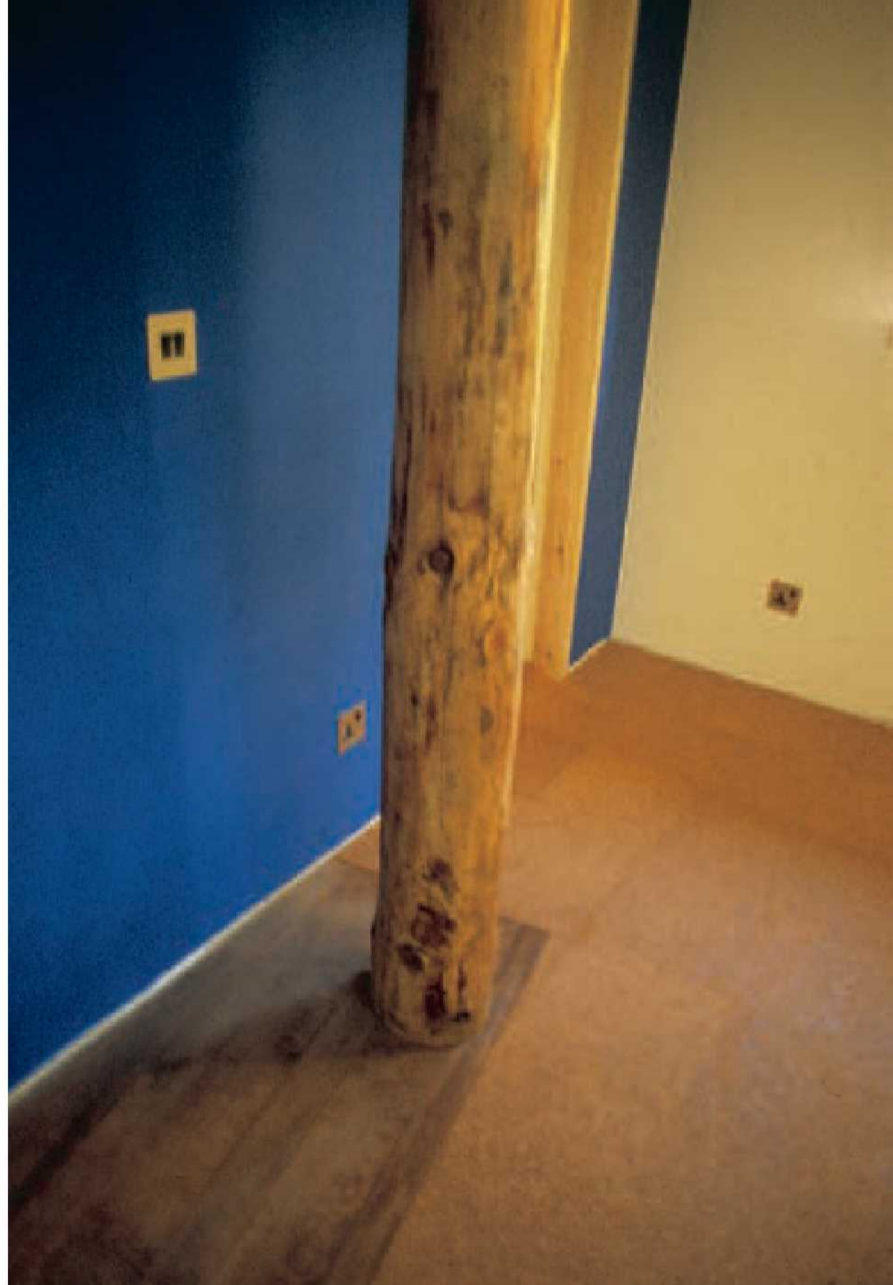
Colour and textures: reused oak and natural cork flooring, natural emulsion paint on the walls.
