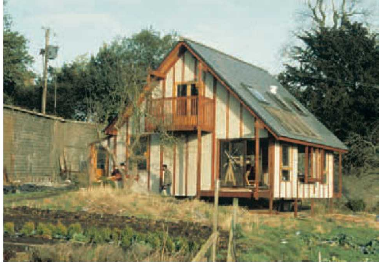
This Segal Method house was taken down and moved from Glasgow to a new site in Fife in the east of Scotland. The original arrangement included a large conservatory, but the plan was substantially amended when the house was rebuilt.
