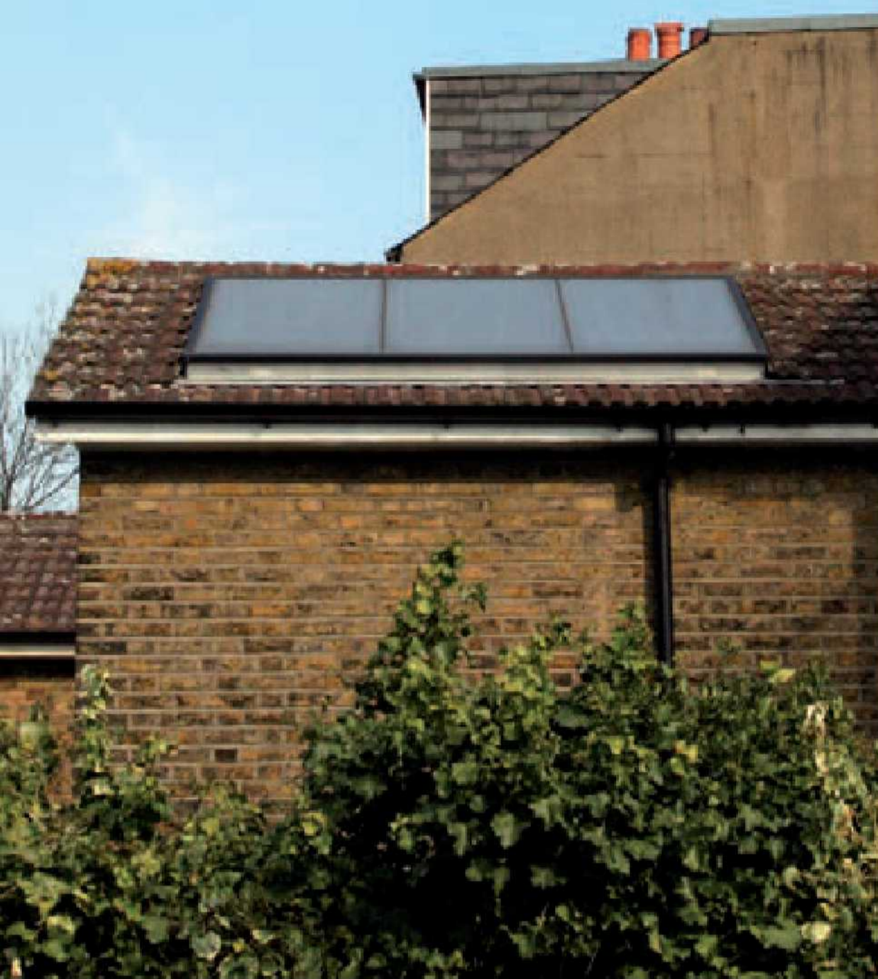
Most new and half existing homes can accommodate solar hot water panels, which will provide up to half the hot water requirement.
