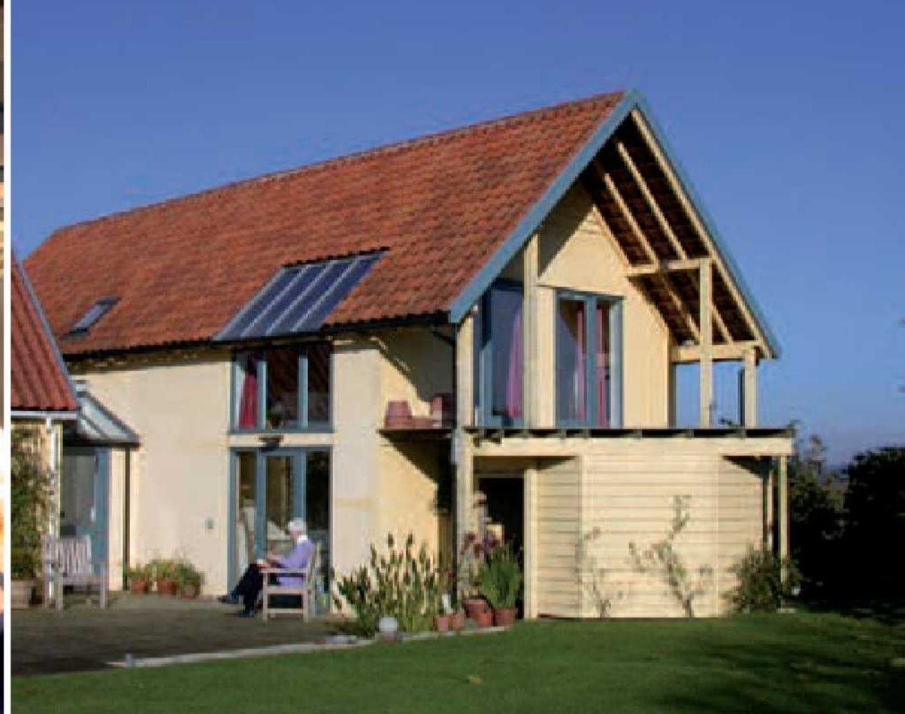
Left: The original house was stripped back to the timber frame and restored. Right: The recent bedroom extension is built using hemp.
