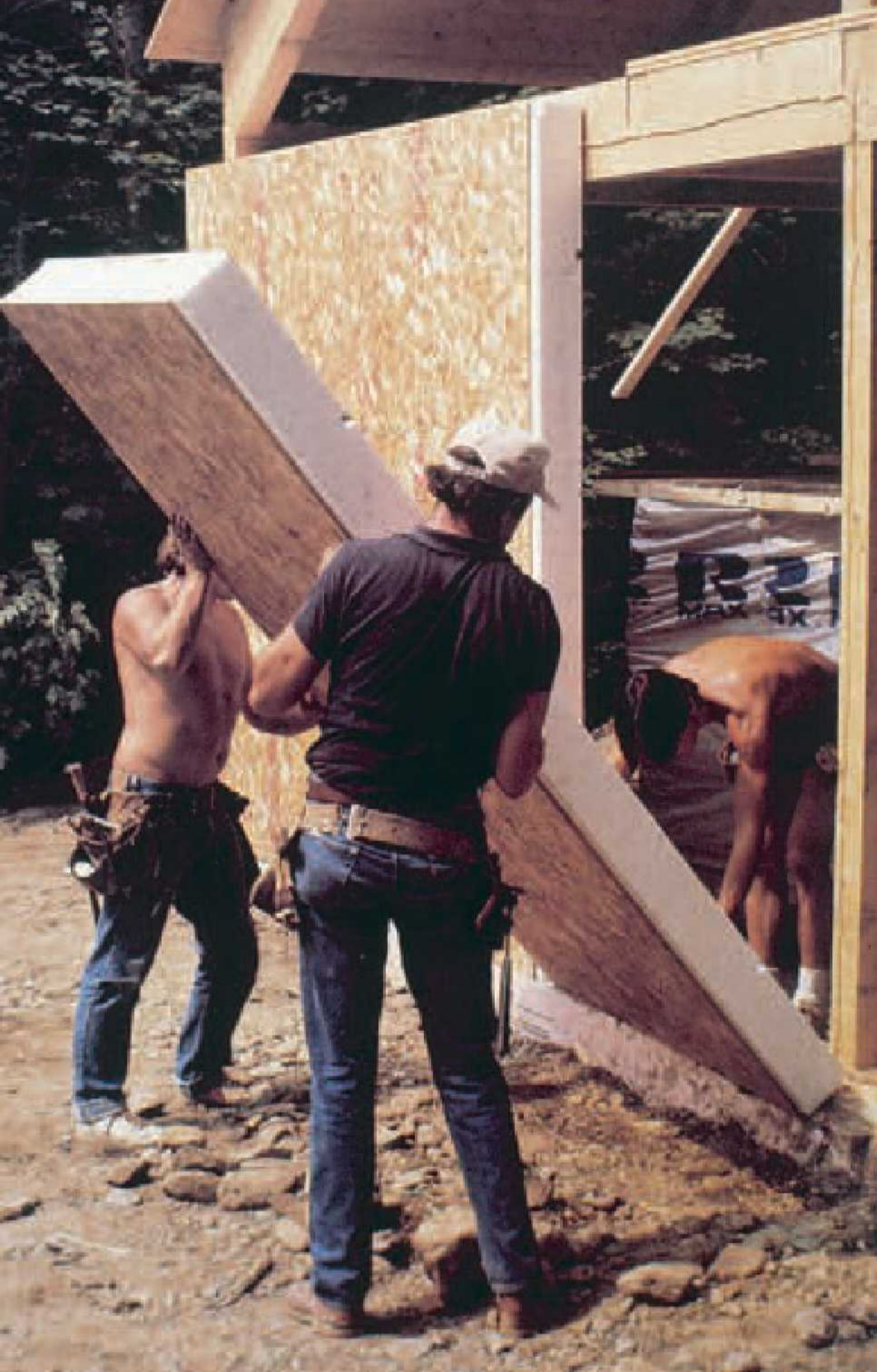
Structural Insulated Panel Systems (SIPS) are made from foam plastic insulation sandwiched between OSB boards. They can be used for walls and roof to quickly create a well-insulated, airtight envelope.
