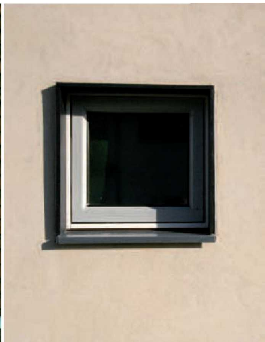
Left: Douglas fir is classified as a moderately durable species, here used as cladding without any applied finish to eliminate maintenance. Middle: Tile hanging is another lightweight, maintenance-free cladding. Right: Lime render is preferred to cement render because it requires less energy to manufacture and is less susceptible to cracking.
