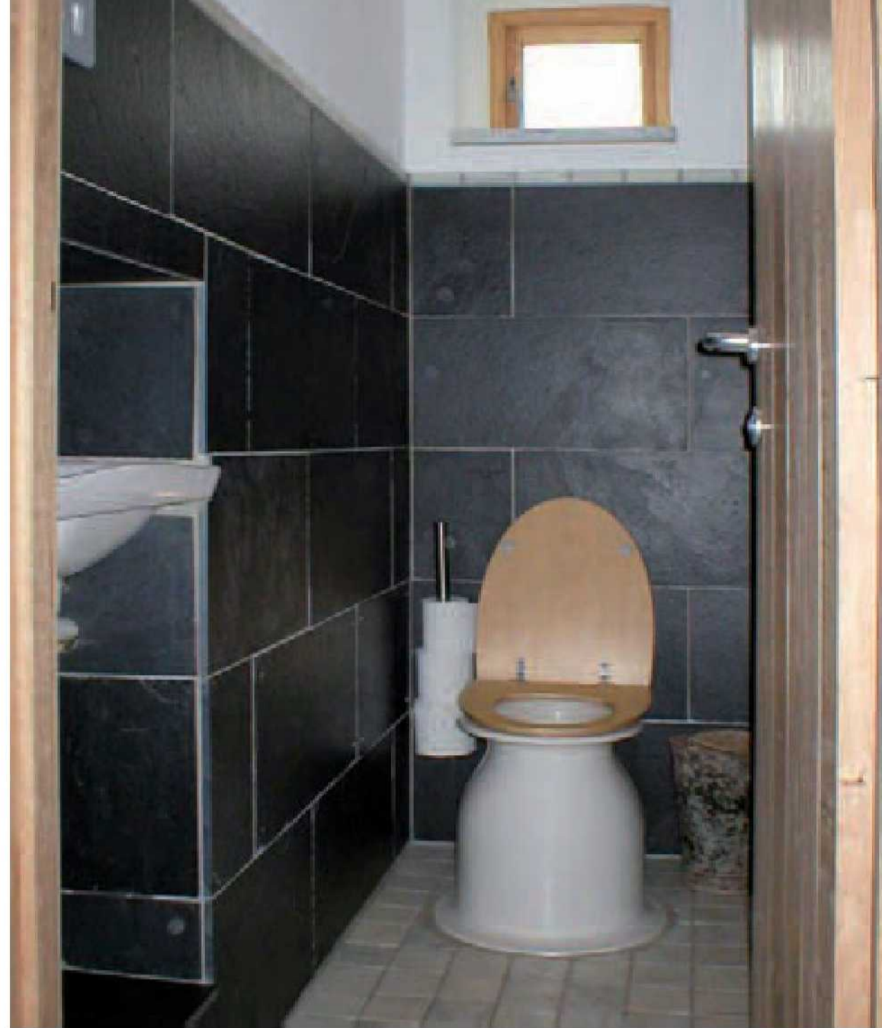
The compost toilet requires the occasional handful of wood shavings, and has a small extract ventilator so that it produces no odour.
