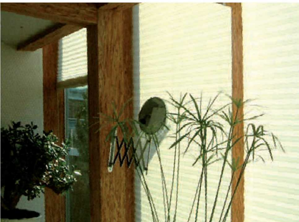
The posts and beams of this house are made from Parallel Strand Lumber, PSL, also known as Parallam. Made from strands of wood bonded together under pressure, it is strong and dimensionally stable.
