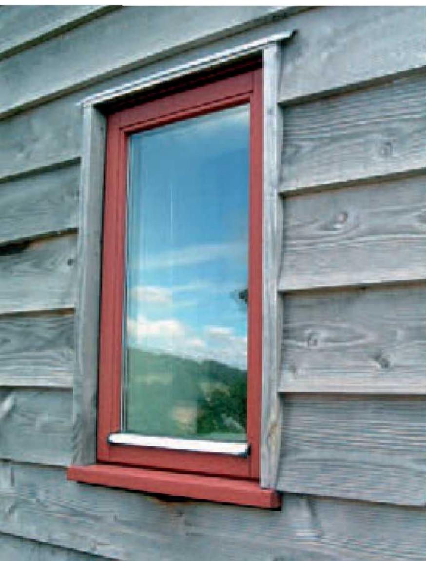
Left: Douglas fir is classified as a moderately durable species, here used as cladding without any applied finish to eliminate maintenance. Middle: Tile hanging is another lightweight, maintenance-free cladding. Right: Lime render is preferred to cement render because it requires less energy to manufacture and is less susceptible to cracking.
