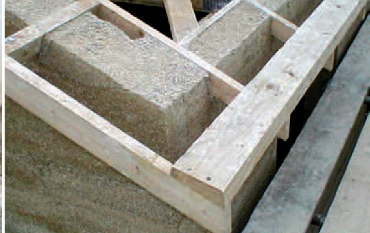
Left: Walls are constructed by packing a mix of lime and hemp into formwork to fully enclose the timber frame. Right: The hemp/lime mix is built up to the underside of the roof, which forms an airtight construction.
