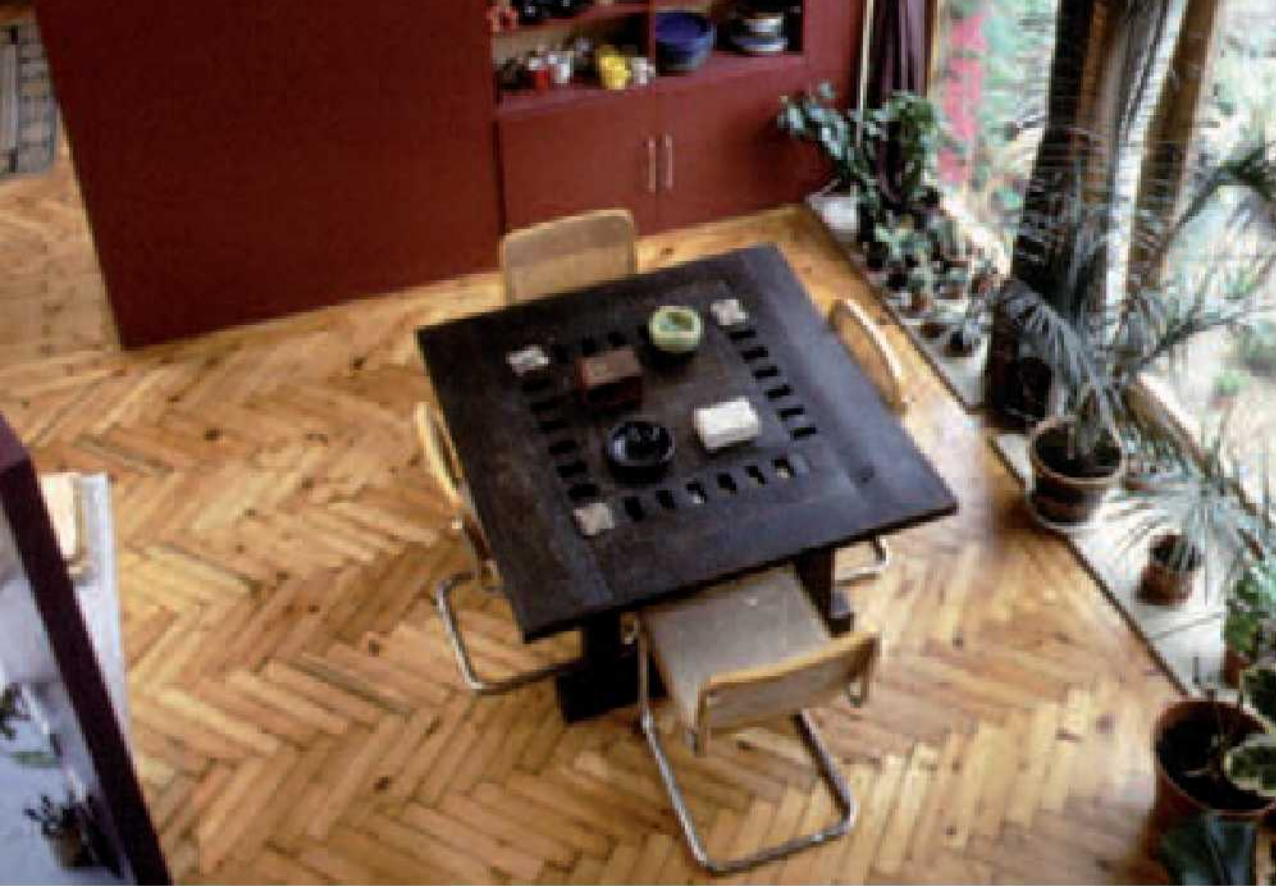
Left: The owner saw the wood blocks being thrown out, but they make a really good-looking floor. Right: Second-hand bricks often have much more character than machine-made new bricks. However, second-hand materials may not be readily available in all areas.
