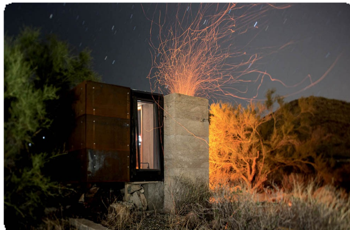
ABOVE: Concrete courtyard and chimney
