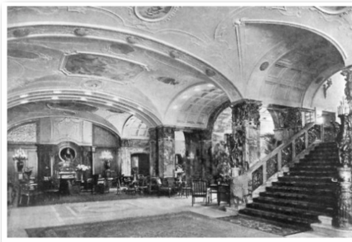
[Image] Hotel Adlon lobby
