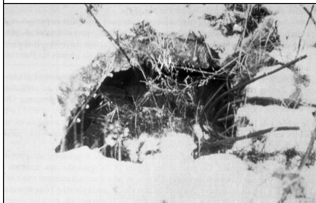
Illustration 7: Alleged Zyklon B input hatch in the ceiling of mortuary 1 (‘gas chamber’) of crematorium II. It is clearly visible that the reinforcing bars in the reinforced concrete were not even removed; they were merely bent back.
