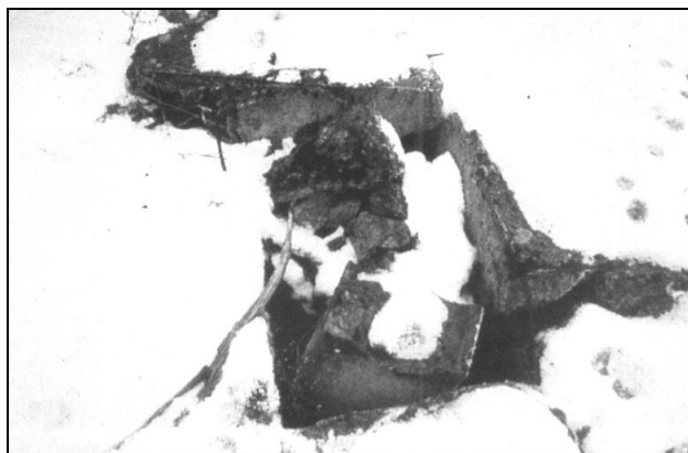
Illustration 5: Cleanly cut ventilation hole in the ceiling of the furnace room, opening into upper story. Note the damage caused by blasting.
