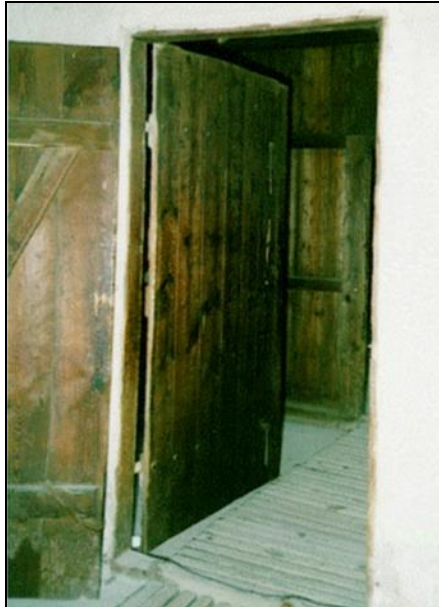
Photograph XVII: Barrack 41, gas chamber, north door. The inside of the door is marked by the typical discolorations that are also visible on the outside of the south door (Photograph XVIa); hooks for the latches are missing from the door frame, unlike on the frame of the south door (Photograph XVI). (© Carlo Mattogno)
