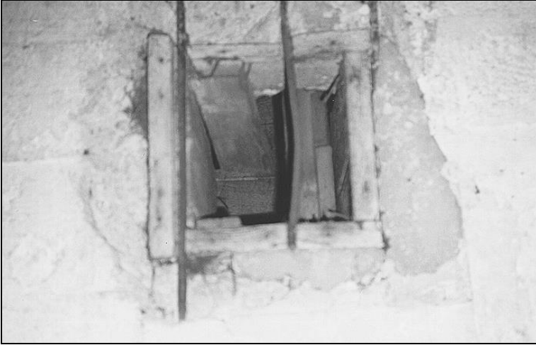
Photograph XI: Disinfestation facility, Barrack 41, Chamber I, opening in the ceiling. (© C. Mattogno.)
