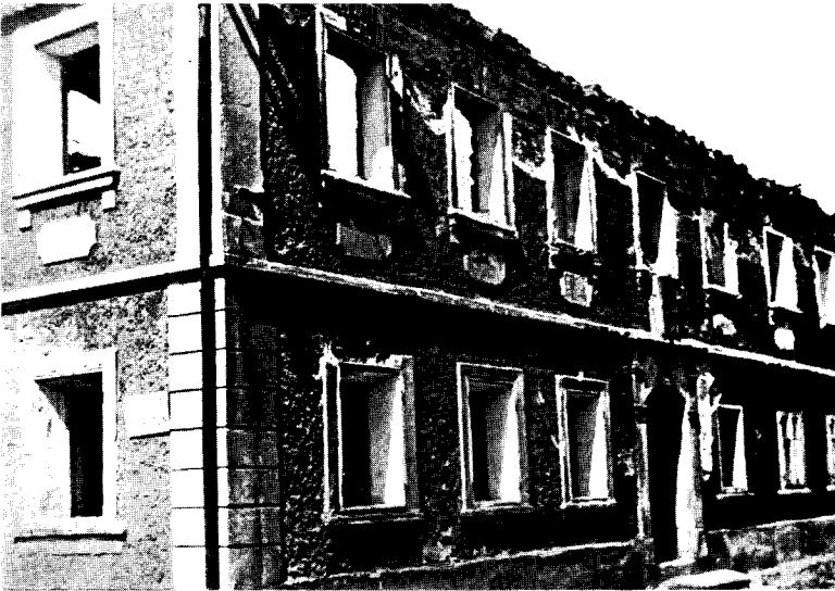
Derelict German School in Eger-Karlsbad District.
