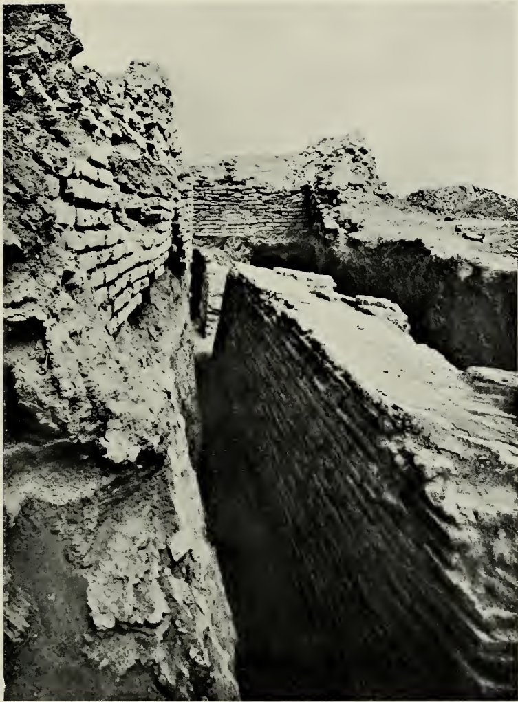
OUTER FACE OF A FOUNDATION-WALL AT TELLO, BUILT BY UR-BAU, PATESI OF SHIRFURLA.
