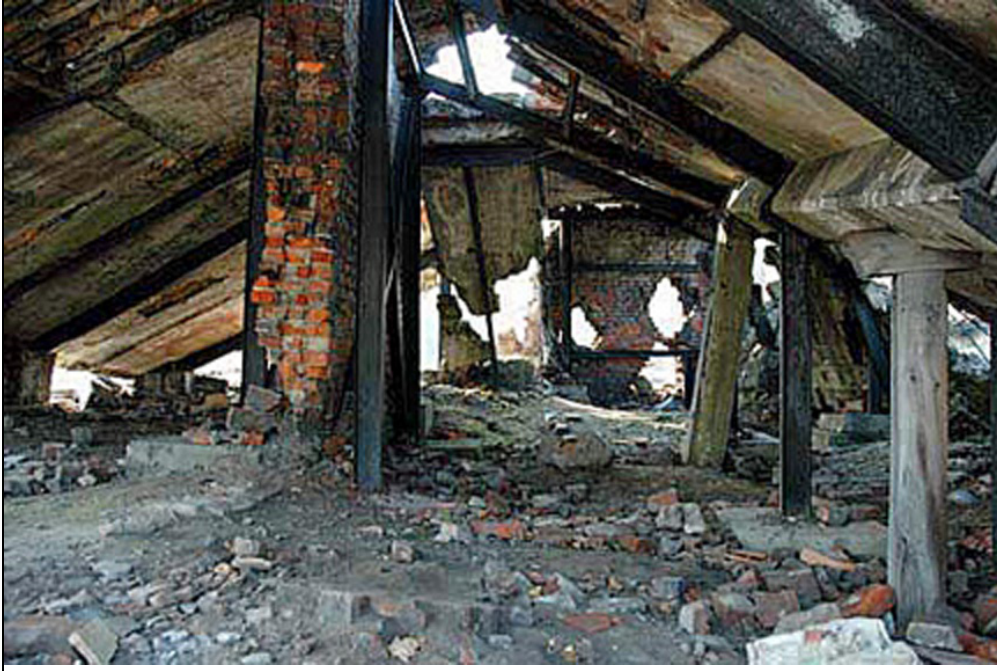
Illustration 14: Under the collapsed roof of the furnace hall of Krema II, Auschwitz-Birkenau.
