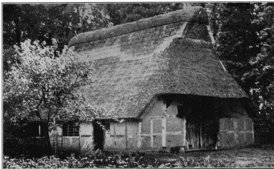
Lower Saxony farmhouse, half-timbered with clay
