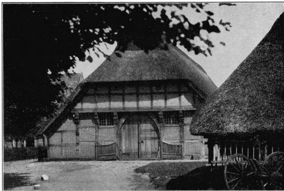
Lower Saxony farmhouse, half-timbered with clinker (Oldenburg)
