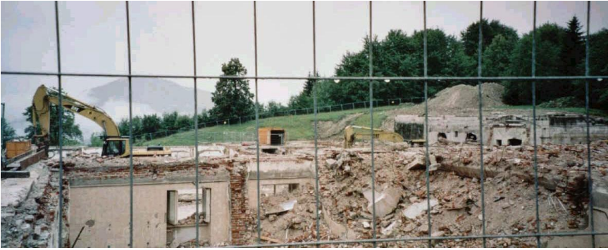
Demolition of the Platterhof at Obersalzberg
