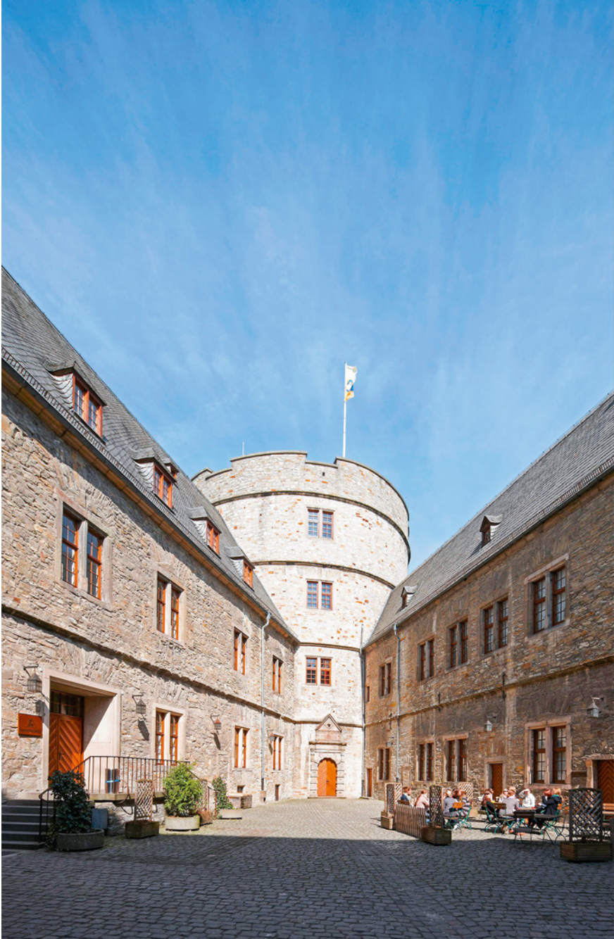
View of the inner courtyard toward the northern tower.
