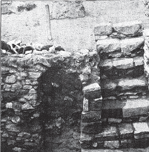
Fig. 4 Stone staircase and niche in the cellar
