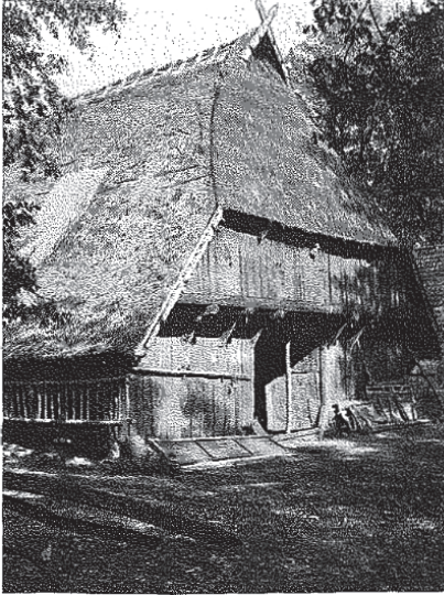
Fig. 3. full farm in Hupsahl, district of Celle. The entire stable side of the farmhouse shows oak timberwork. Exceptionally strong borking of the roof gable with headbands on the outside and heavy wooden nails. Soon after 1600.
