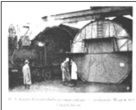
Fig. 13: A lice-ridden train enters a railway gassing tunnel in Budapest. 112
