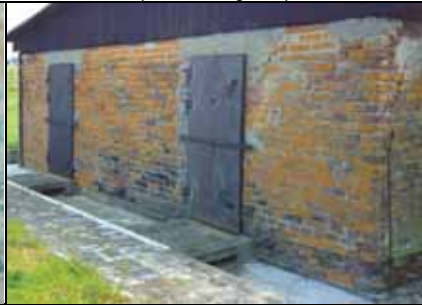
Fig. 64: Zyklon B disinfestation installation, chambers II and III (exterior wall), of barrack 41 in Majdanek camp. (© Carlo Mattogno 333 )
