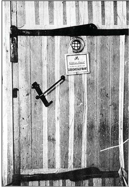
Fig. 32: Wooden disinfestation chamber door at Auschwitz, rendered provisionally gas-tight with peephole and metal protection grid. This is what the gas-tight doors for the homicidal “gas chambers” are supposed to have looked like. Note the extremely flimsy lock.
