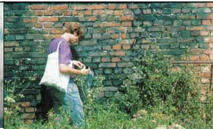
Fig. 60: Exterior southwest wall of the Zyklon B disinfestation wing of BW 5b in the Birkenau camp.
