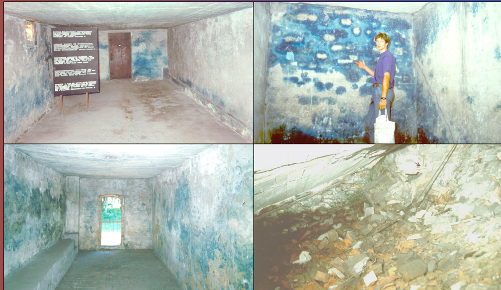
Blue staining of delousing chamber walls, as a result of exposure to Zyklon B: Majdanek (top left), Auschwitz-Birkenau (top right and front cover), Stutthof (bottom left). No staining can be found in the ruins of the morgue no. 1, the alleged 'gas chamber' located in the former crematorium II of Auschwitz-Birkenau (bottom right).
