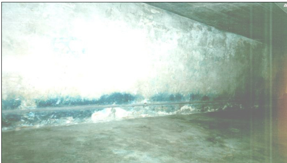
Photograph XIII: Disinfestation facility, Barrack 41, Chamber III, east wall.
