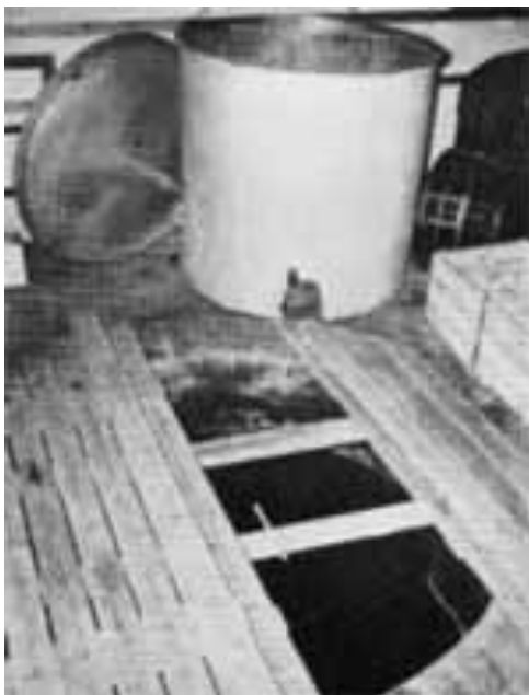
The reactor pit and alloy vessel in the Berlin-Dahlem bunker laboratory — the Virus House
