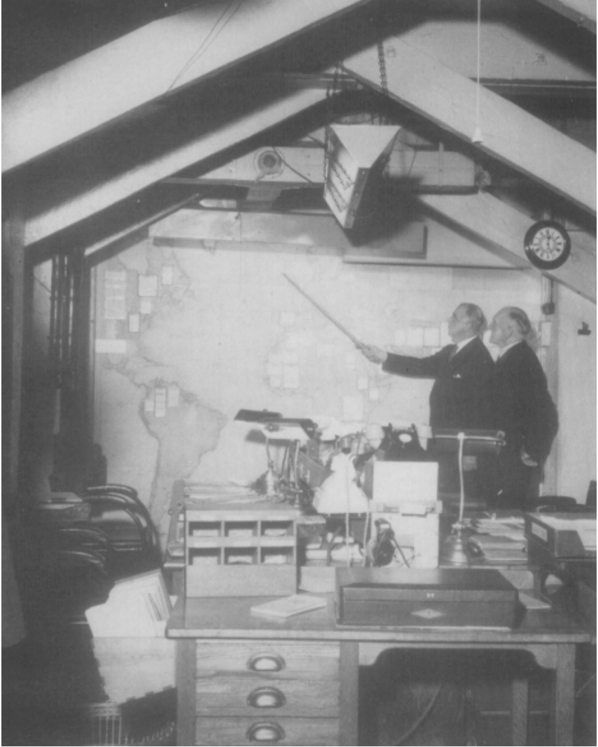
The secret underground headquarters of the war cabinet and the chiefs of staff in Marsham-street, Westminster, London. The building, designed to hold over 2,000 people, included radio and power stations. Shown here is Lord Ismay in the map room of the underground headquarters. With him is Mr G. Ranse, to whom all correspondence was addressed during the war, when the war cabinet offices were a top-priority secret.
