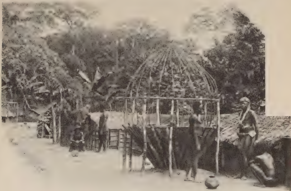
CONSTRUCTION OF A NATIVE STOREHOUSE, TURUMBU.
