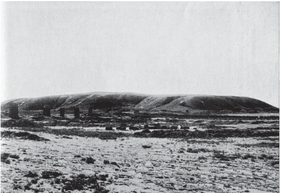
Fig. 16: The Akapana hill fortress in Tihuanaku. The fortress can be seen in the background, its ground plan, which is in the typical staircase shape, can be seen in the shadow effect. In the foreground on the left the western wall of the Kalasasaya solar observatory, on the right the Palace of Sarcophagi Phot. Professor Arthur Posnansky in La Paz.
