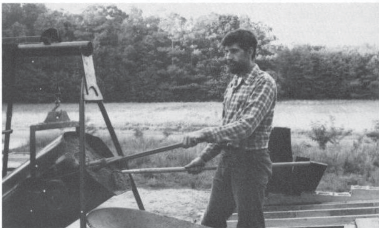
Fig. 10-6. Mr. Greenlaw using a home-made concrete mixer.
