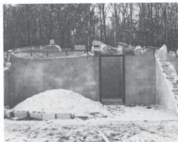
Fig. 2-13. Underground construction above virgin grade.
