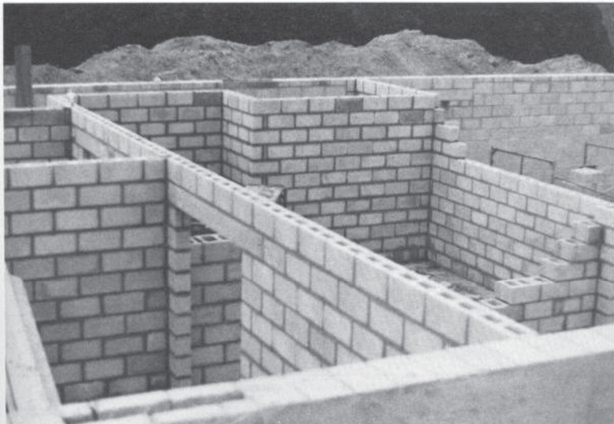
Fig. 8-5. Final stage of blocklaying.
