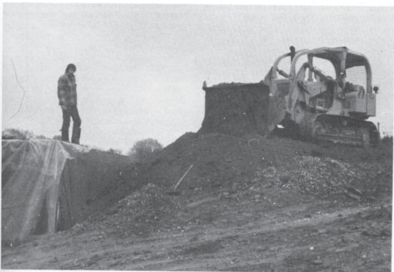
Fig. 13-11. Don't get into a rush and let the bulldozer go on the roof. This is me guarding against possibility. (My neighbors thought I was going to jump, but I fooled them.)
