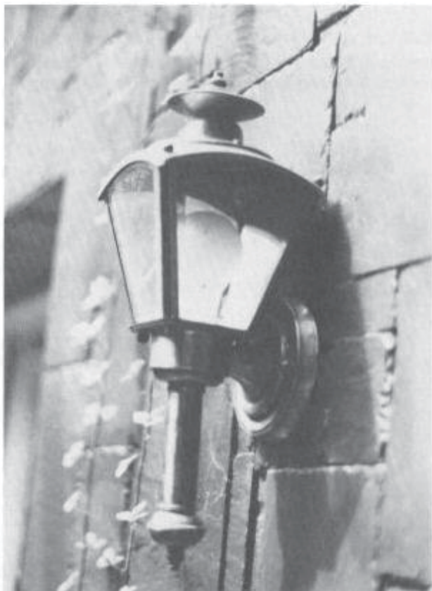
Fig. 16-12. Wall lighting is necessary.
