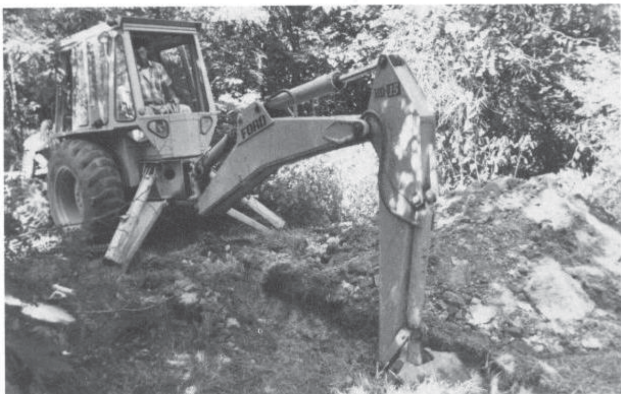
Fig. 4-5. A backhoe in the digging position.
