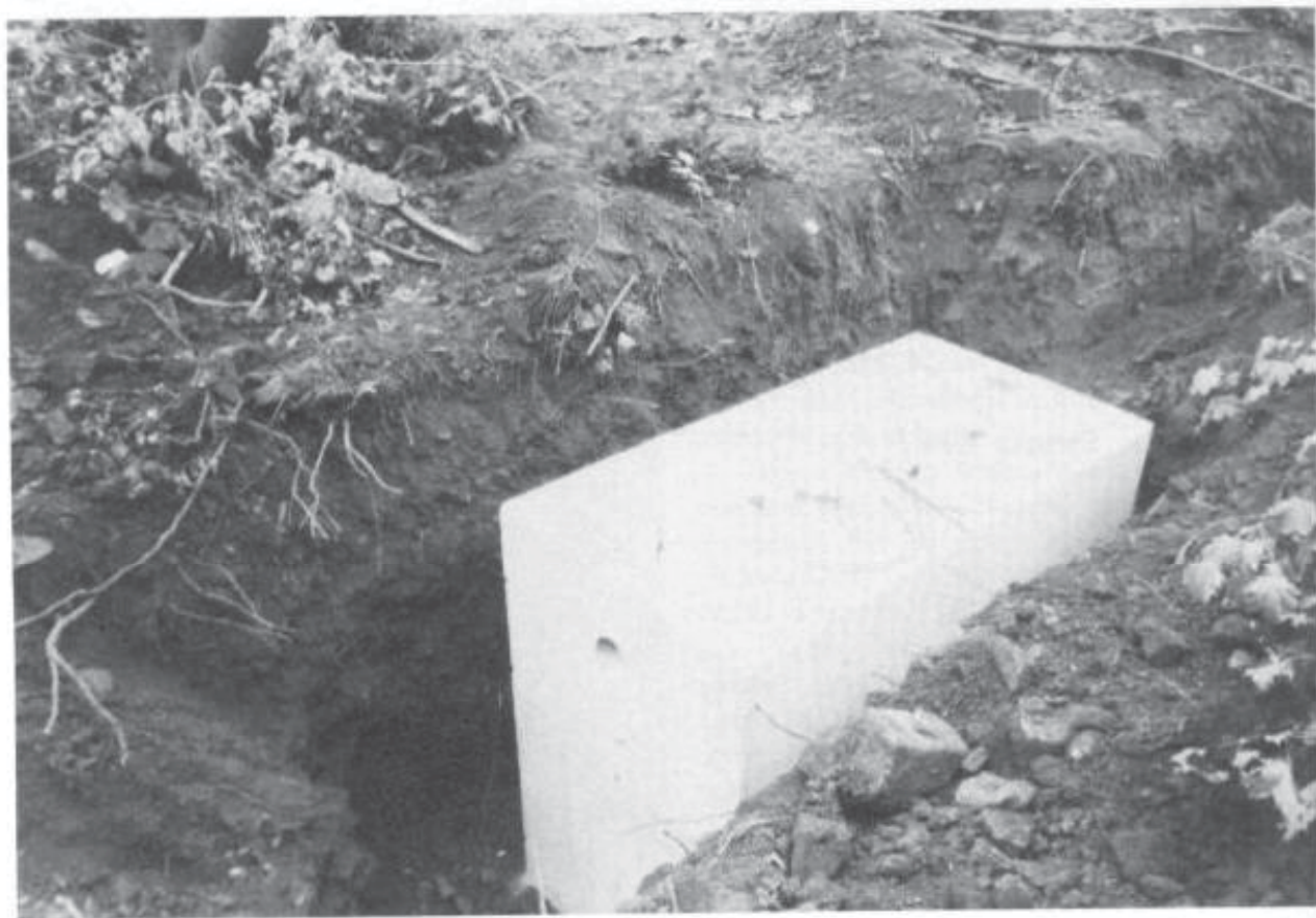
Fig. 6-7. Concrete septic tank in place.
