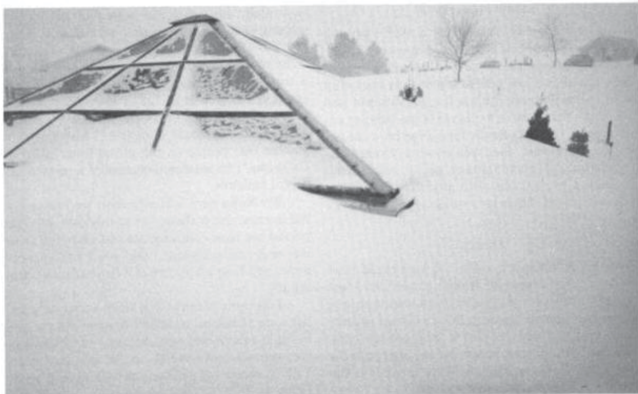
Fig. 1-2. Typical view of my skylight after a snow storm.
