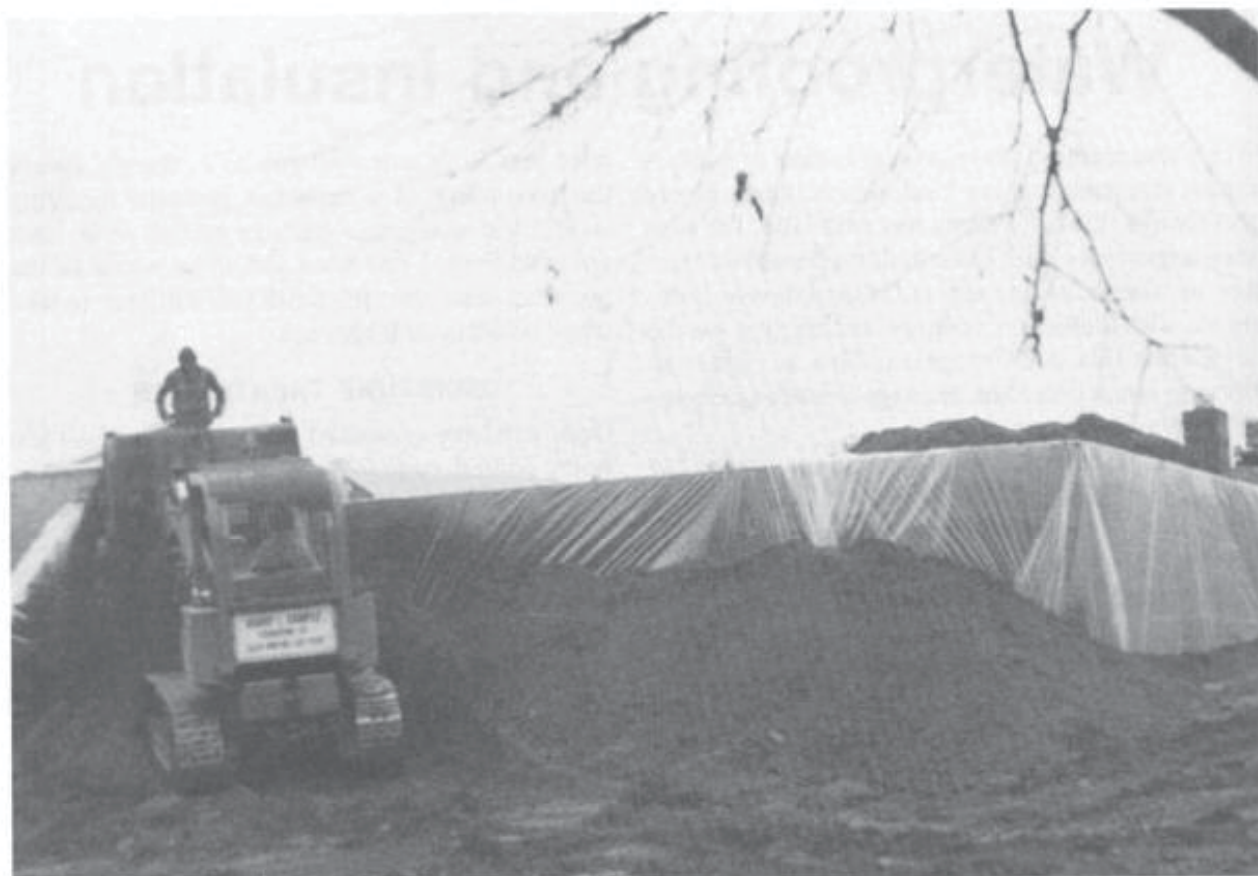
Fig. 11-1. The structure was coated with two coats of hot tar and then wrapped in 6 mil polysheets.
