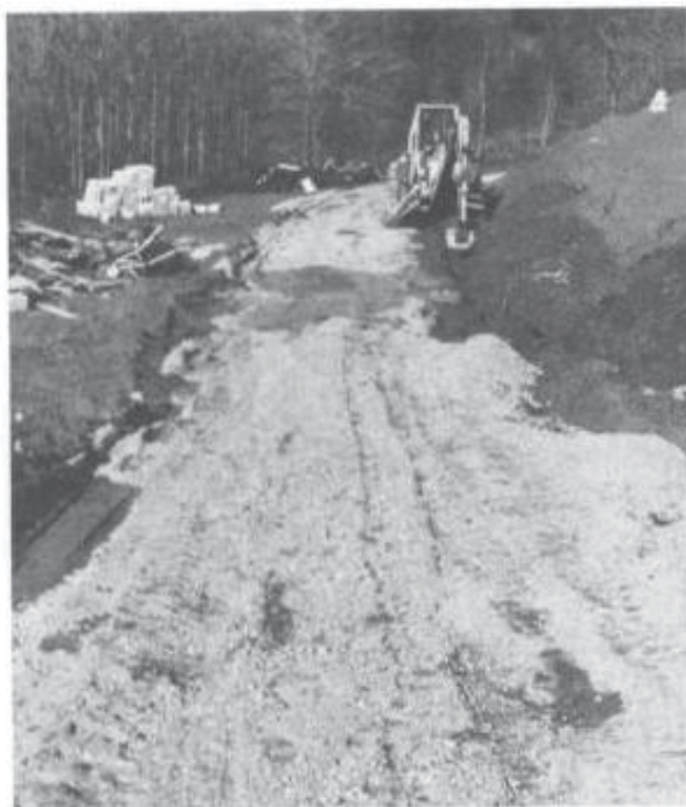
Fig. 6-4. Cutting the driveway on a new building site.
