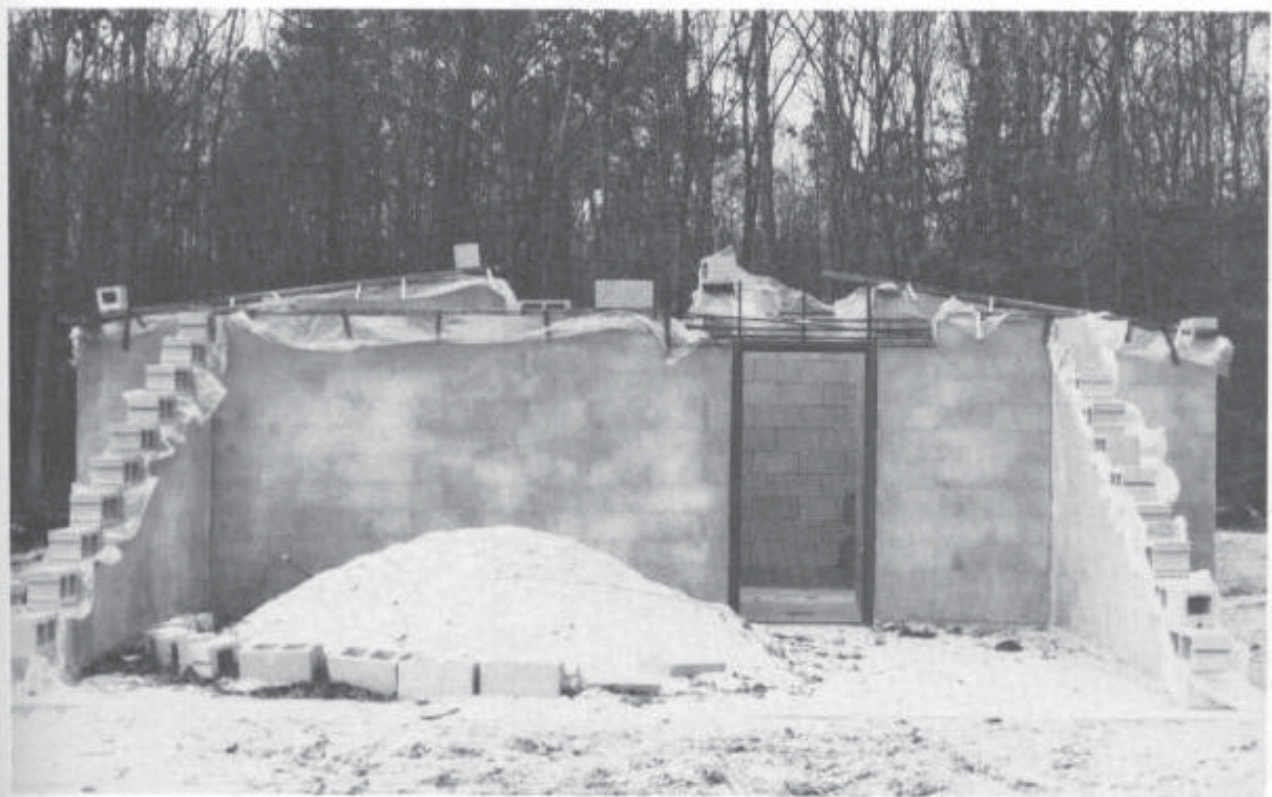
Fig. 10-8. Front view of block construction.
