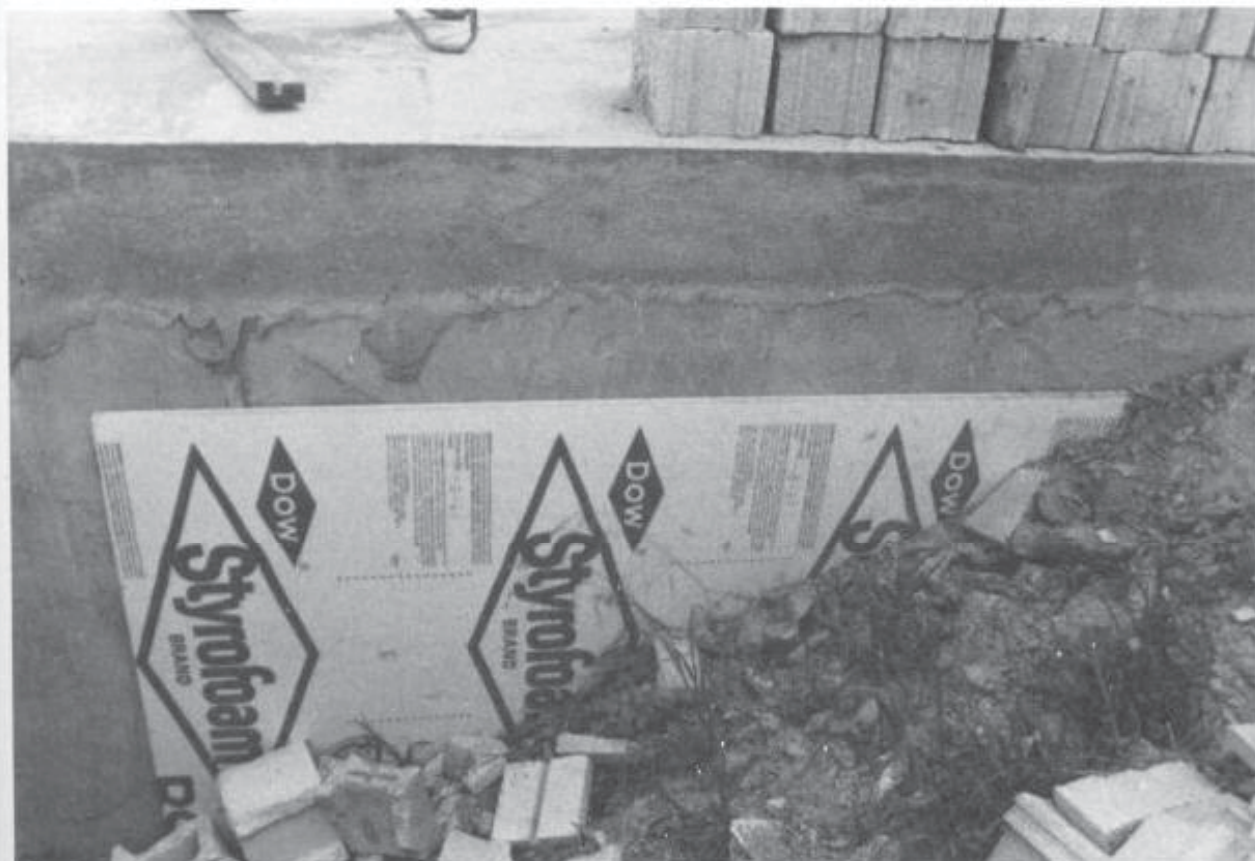
Fig. 11-7. Insulation board can be used on the roof. Use high-density, water proof material.
