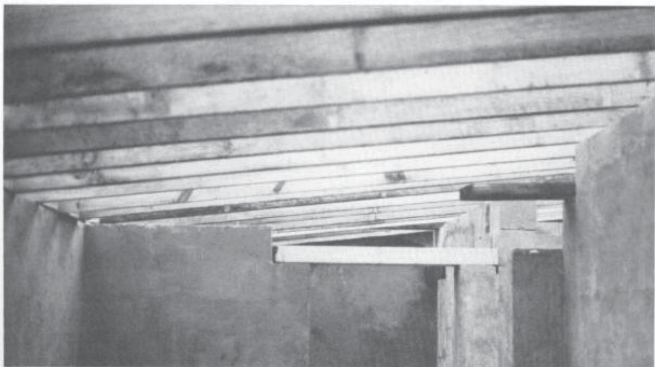
Fig. 10-7. Notice block interior walls and sloped rafting.
