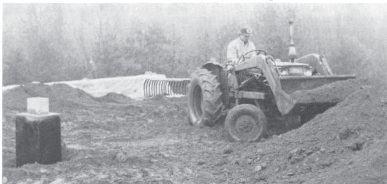
Fig. 13-9. A small tractor works well for placing earth on the roof.
