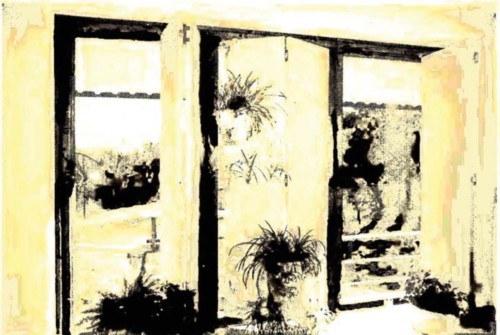
Closable, high "R" value, insulating panels in a house cantilevered into the trees.
