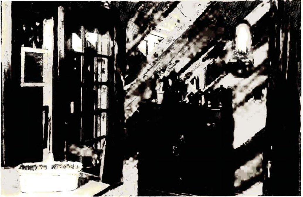
Walls of weathered hardwood scraps with occasional pieces of off-fall mirror. Designed by author for very special friends.
