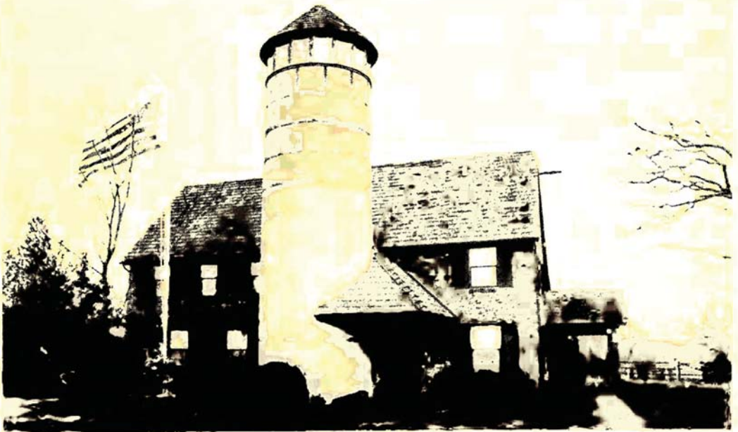
A Missouri farm residence built around a silo. Room on top has wood casement windows for walls.
