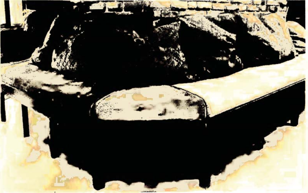
Artist Beverly Hopkins' self-executed built-in bench. The edge is faced with thin pieces of Brazilian rosewood installed with grain running end-to-end.
