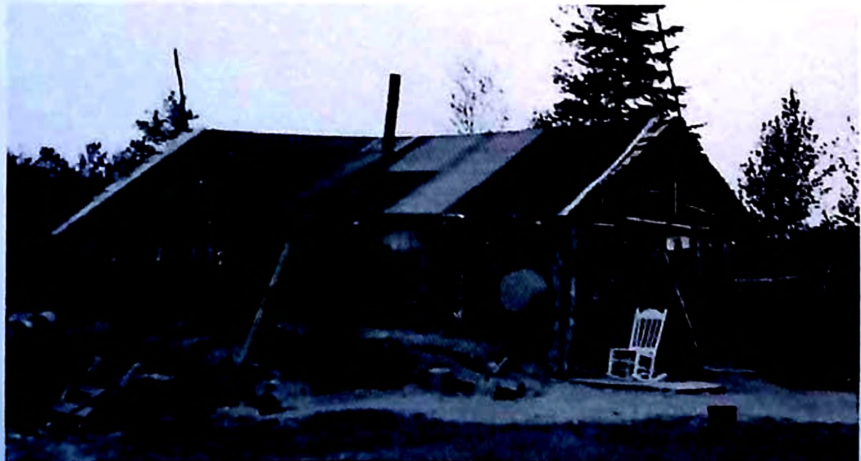
The minimum family housing that I have seen on my travels in the United States and Canada is this pole house in Canada. A family was actually living in it. It is made like a log fence with the logs stuck into the ground with an earth floor. It is too wasteful of wood.
