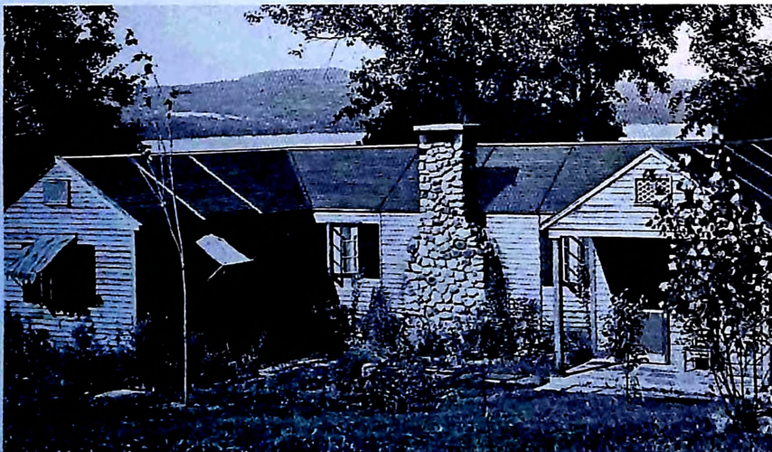
Middle and Bottom: The secret of making smaller houses attractive is to build in attractive surroundings and keep them neat. Keep junk and trash behind lattice or bushes. These 1930s houses were built long and narrow for a good view from every room. You can do this when land is plentiful. They cost more to heat but it may be worth it.
