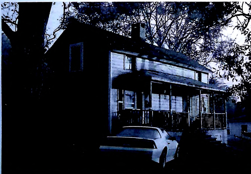
Traditional Southern mill house. They are good to live in, and will probably appreciate in time.
