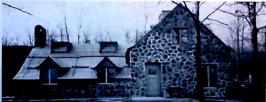
Flagg house shown finished and under construction
