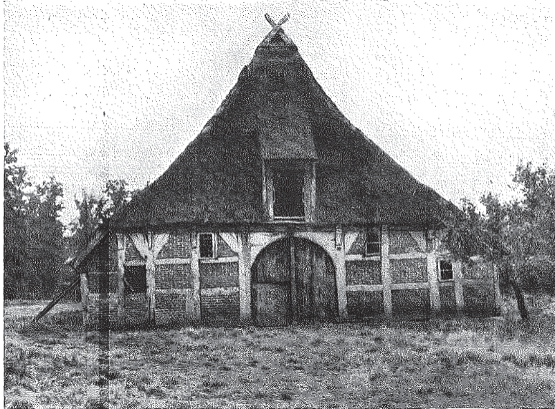
Fig. 1: Bauernhaus on a bollhos. Wall design in the old state. Modern roof extension. Built before 1600. Demolished in 1937. District of Soltau (north).": Author
