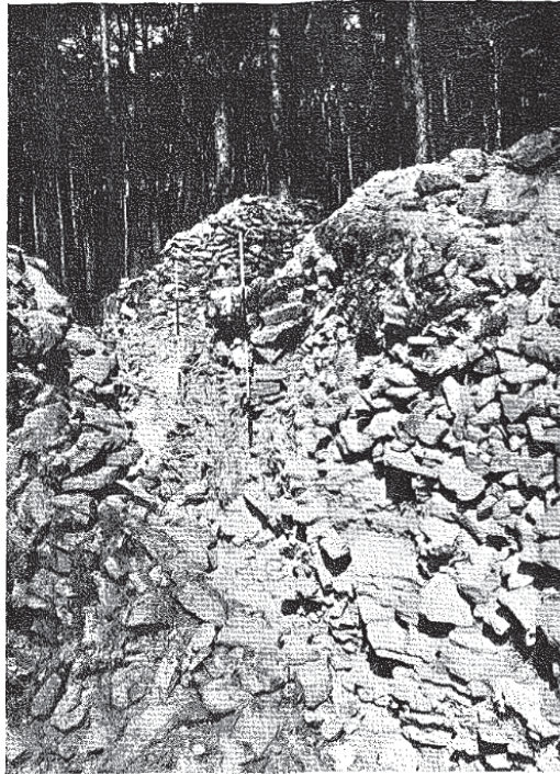
Fig. 5 Current profile of the crumbling wall
