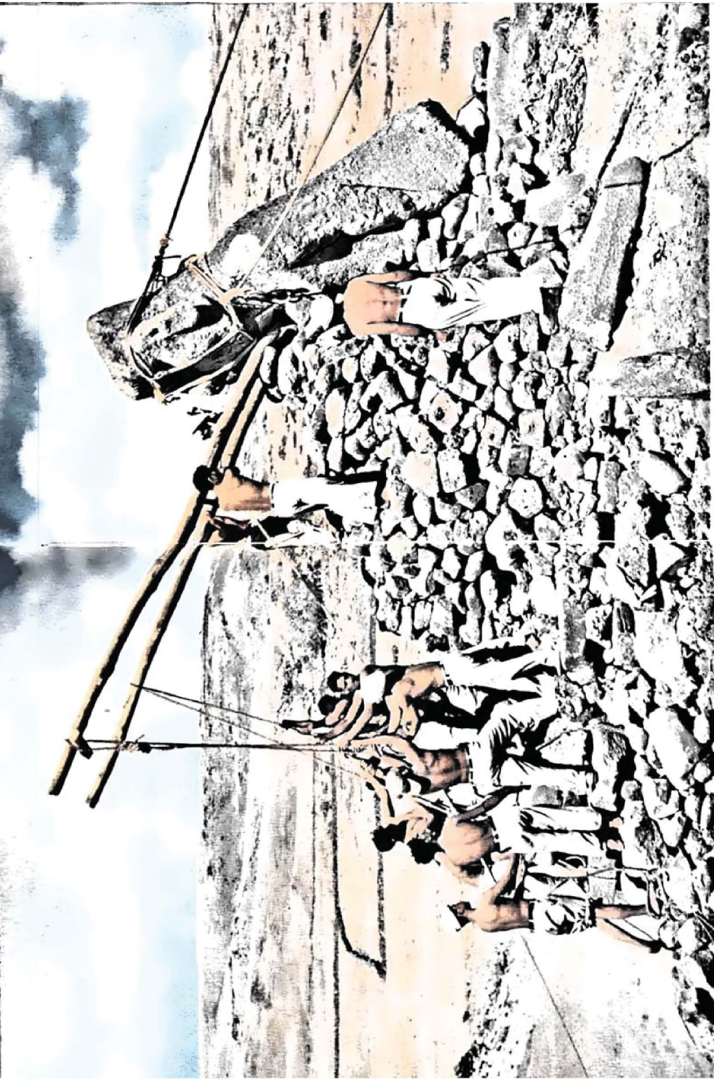
With a heap of stones under its stomach the figure moves upwards and backwards until it stands in its old place on the wall. Twelve men with poles and stones set it up in eighteen days. On the last day the giant is held by ropes to prevent it from toppling off the high wall when it is tilted into the standing position.
