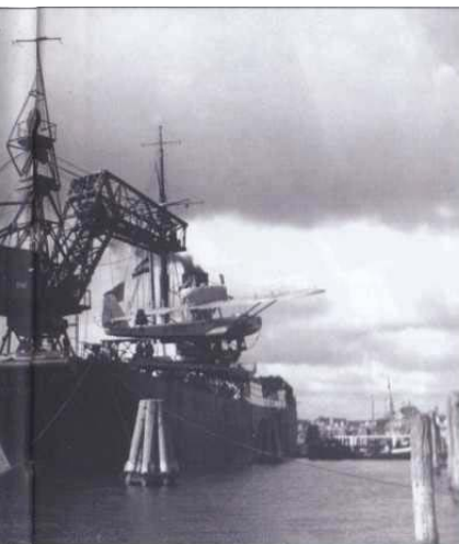
The "Westfalen" was equipped with a slewing crane. Becker could lift loads of 15 tonnes from ships at an angle of 15 degrees.
