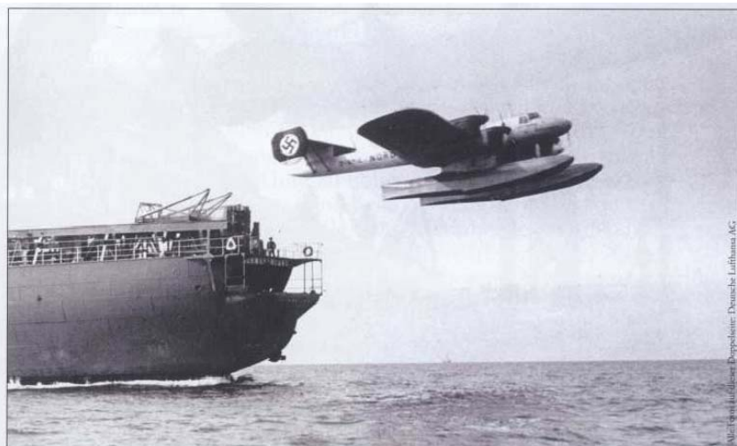
It is clear to see that the flying boats were catapulted backwards, which made the folding crane necessary.
