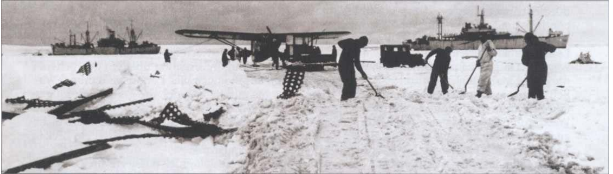
A crevasse is bridged with the help of steel and snow. "Little America" is given an airfield made of compacted snow, from where 29 reconnaissance flights are undertaken far into the interior of the continent.
