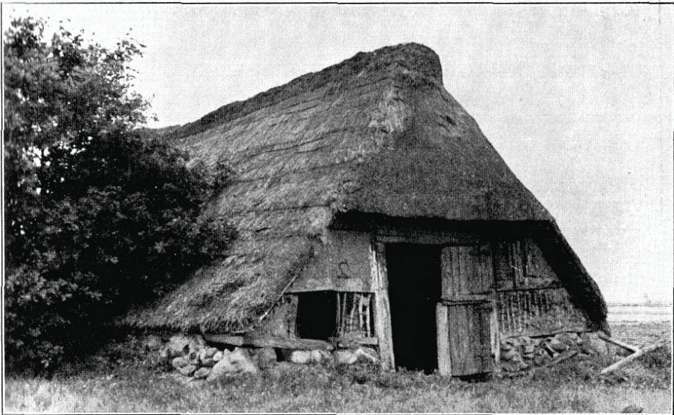
Roof on a boulder wall (Lower Saxony-Oldenburg)
