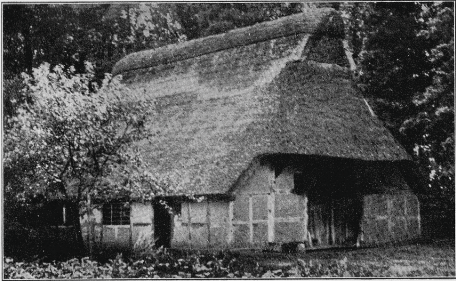
Lower Saxony farmhouse, half-timbered with clay
