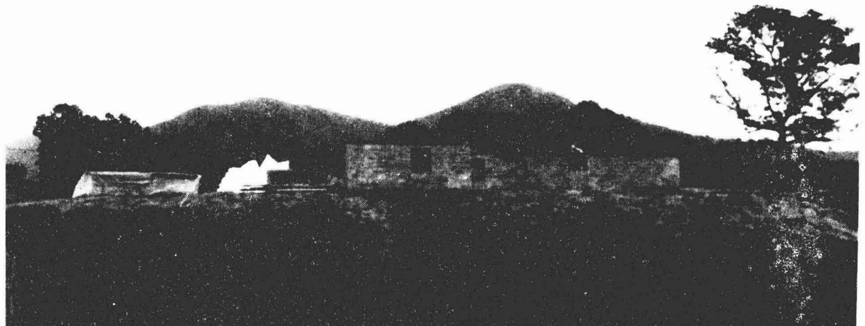
Site of the School looking at it from the West side. From this small
