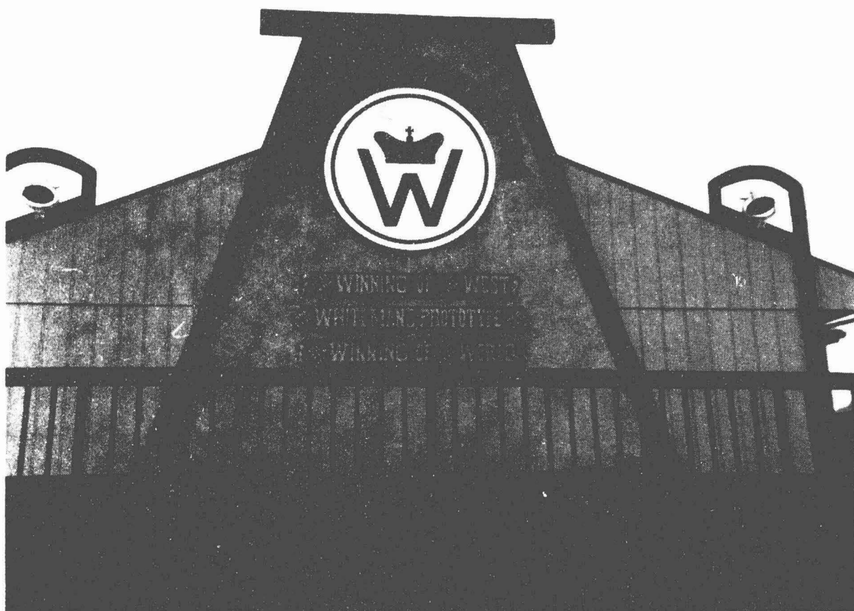
Close-up of the top floor of the front of the building, showing the Creator Logo and our three-tiered
