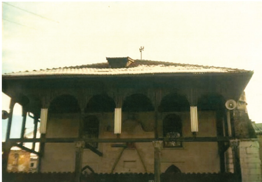
FIGURE 18 Magribija mosque. This photograph was taken before the start of the reconstruction work on the mosque, which has since been refurbished, and its old and rare wooden minaret, which was knocked down by a shell, has been replaced by a new stone one.
