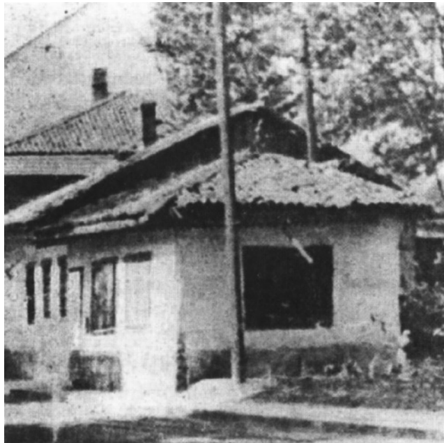
FIGURE 3 Gaziler Türbe sometime before its demolition in 1950. (From Vesna Mušeta-Aščerić, Sarajevo i njegova okolina u XV stoljeću: između zapada i istoka, Sarajevo, 2005; image reproduced with the author's permission.)
