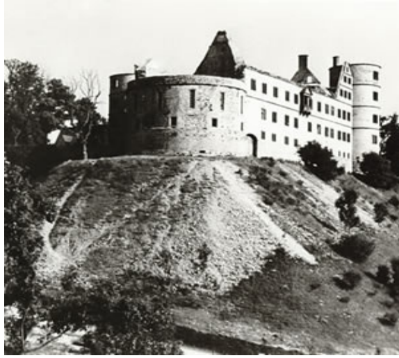
The damaged North Tower, photographed in 1950.
