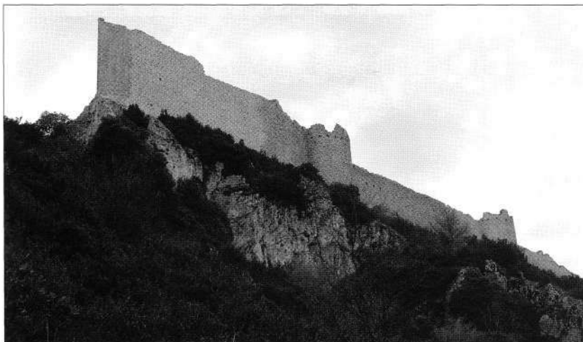
When approaching the hilltop fortress of Peyrepertuse, the first sight of the defences is the imposing northern wall overlooking the gorge. This 120m-long wall is over 1.2m thick and has two towers. At the near end is a triangular-shaped bastion while the entrance to the castle is located at the far end. (Author's collection)
