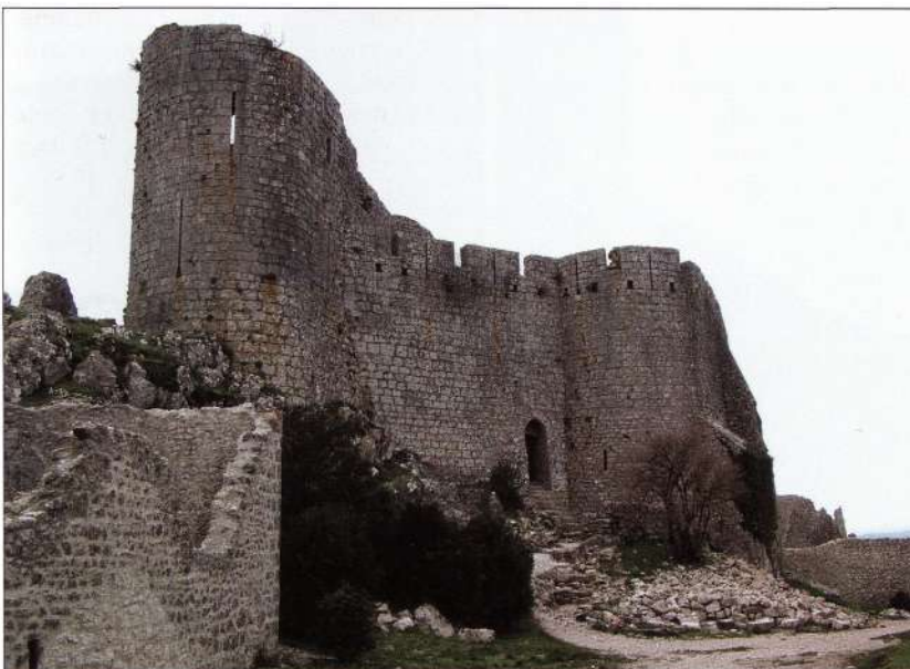
The imposing central keep of Peyrepertuse dominates the lower enceinte of the castle. It consists of two separate structures – a church and living quarters – joined by thick, crenellated walls creating an interior courtyard. (Author's collection)
