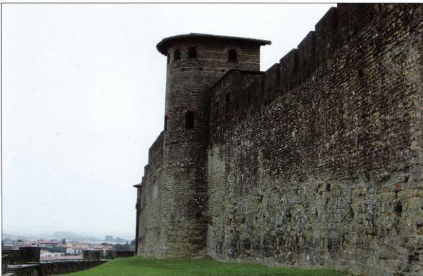
This semicircular tower in the walls of Carcassonne has all the hallmarks of the original Gallo-Roman fortifications of the city. Its shape is characteristic of the defences of the late Empire, updated over time to form part of the medieval fortifications. (Author's collection)
