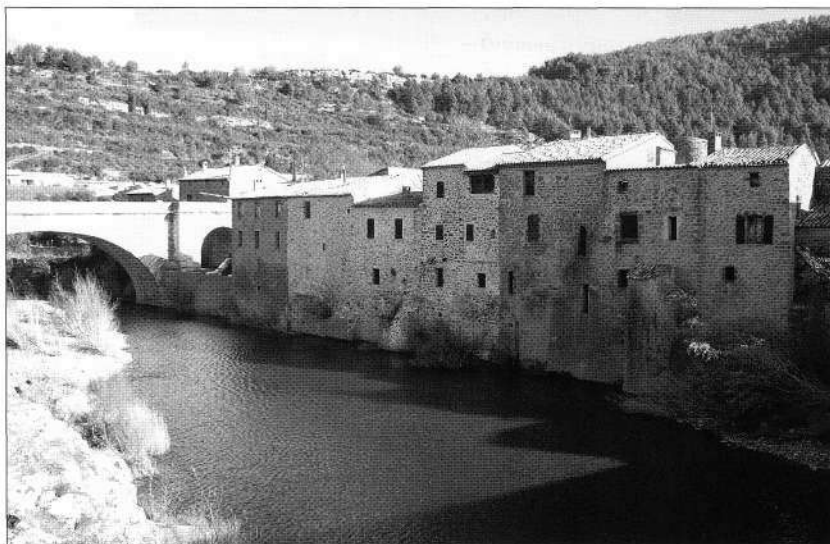
The walls of the town of Lagrasse provide a good example of a medieval system of integrated defence, with the houses backing onto the River Orbieu forming an exterior wall that protects the site. (Author's collection)
