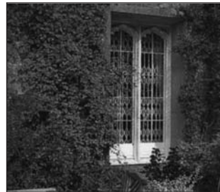
Window grilles need not be unattractive.
