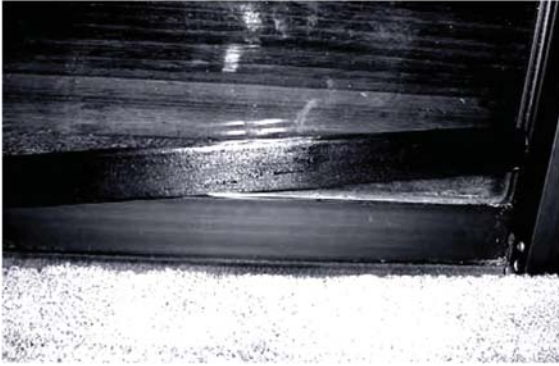
Board out of place to show how to block sliding doors and windows.
