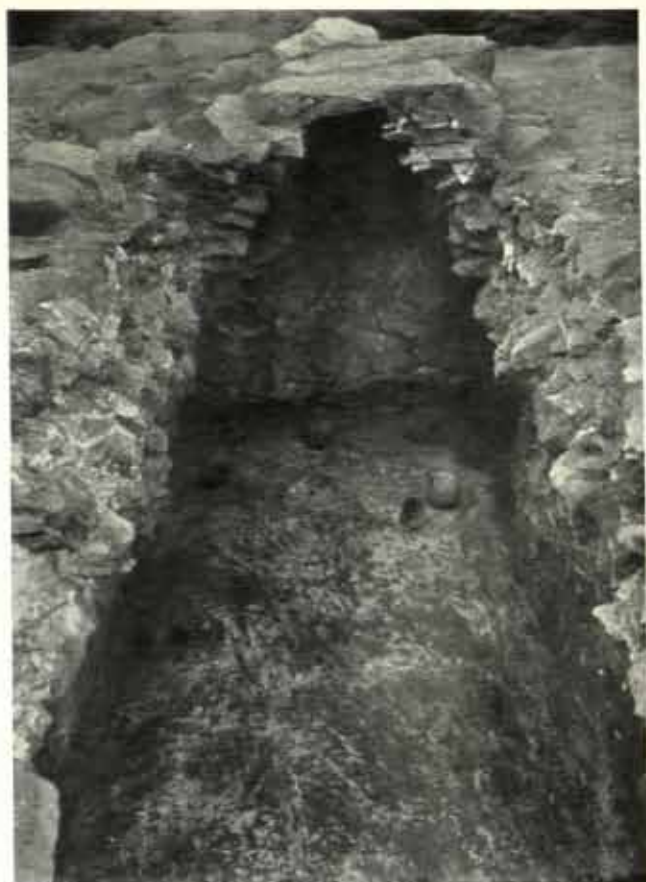
24, a . A corbel-vaulted stone tomb-chamber, Ur (p. 70)
