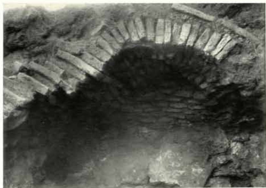
26, a . A tomb-chamber with a brick vault ending in an apse, Ur (p. 71)
