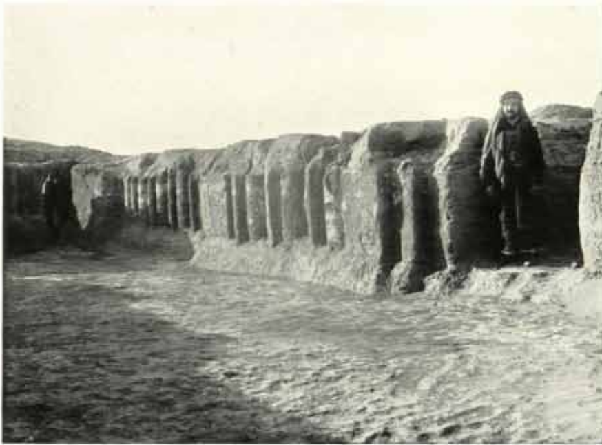
7, c. A wall decorated with half-columns 7th century B.C. (p. 40)
