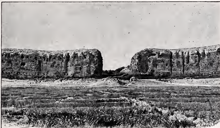
PART OF THE WALLS OF EL-KAB ON THE NORTHERN SIDE. 2
