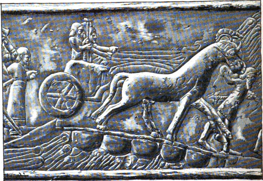
THE KING'S CHARIOT CROSSING A BRIDGE. 1
