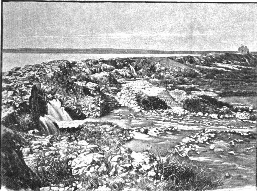
THE DYKE AT BAHR EL-KADES IN ITS PRESENT CONDITION. 1
