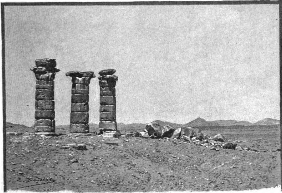
THE THREE STANDING COLUMNS OF THE TEMPLE OF SESEBI. 4
