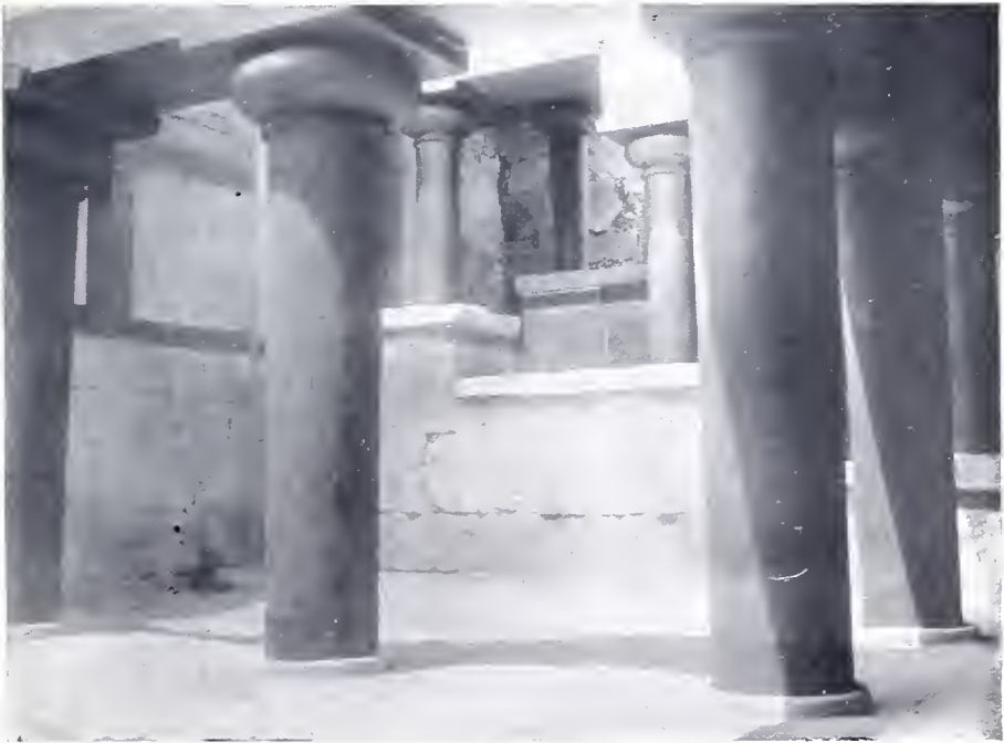
2 GRAND STAIRCASE: LOWER FLOOR
