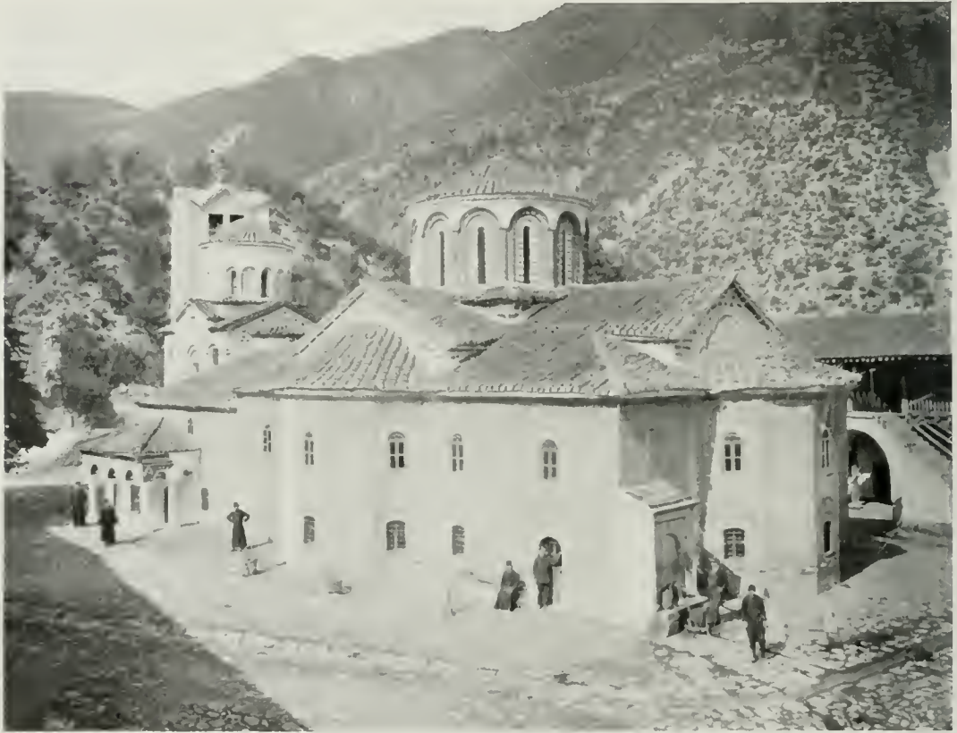
Fig. 39. — The principal church in the monastery of Batshkovo, built in 1604.
